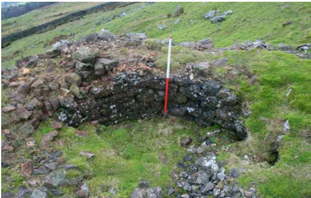
Plate 9: The top of the draw kiln, showing a corner of the rectangular tower and the infilled cylindrical furnace chamber, looking west. The stone forming the inner edge is vitrified.
