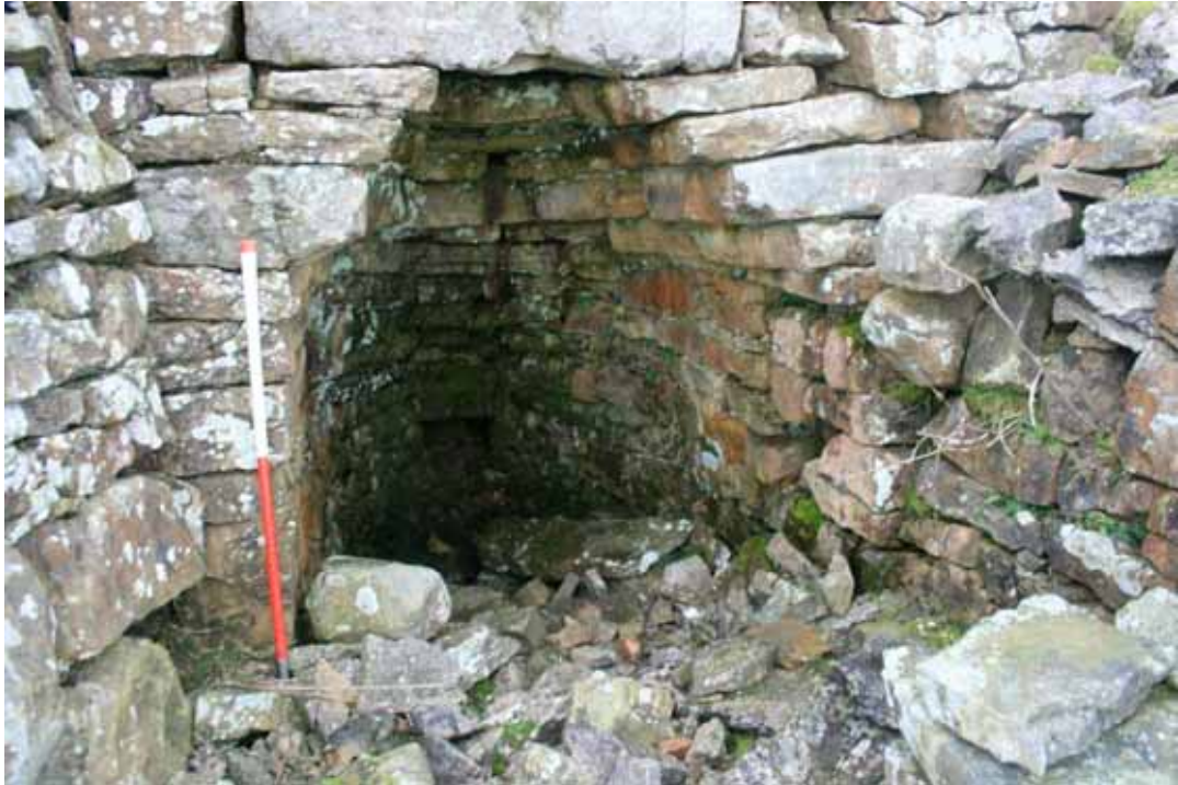
Plate 8: Detail view of the corbelled furnace aperture
