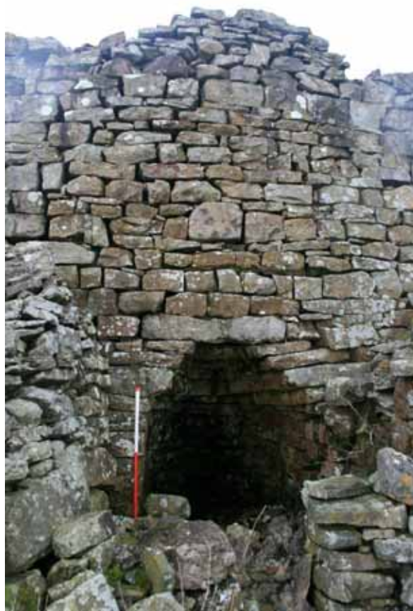
Plate 7: View of the front of the lime kiln (Site 30)
