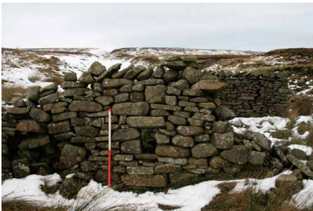
Plate 21: A keep-hole built into an internal wall, with a more recently rebuilt wall in the background (Site 27)
