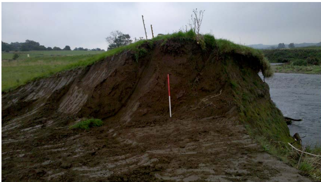
Plate 6: Cross-section through embankment 101 , looking south
