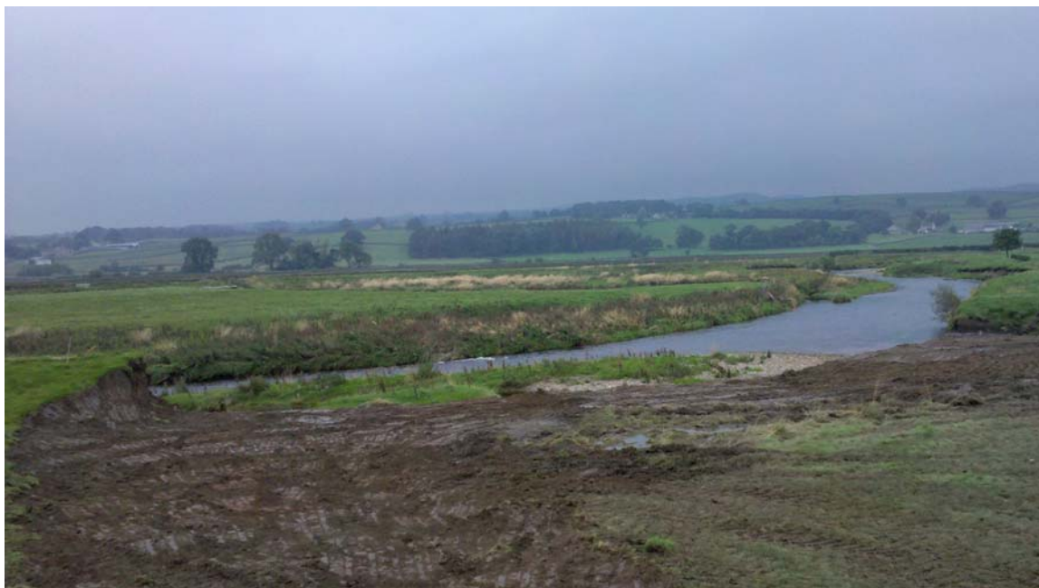
Plate 4: The area adjacent to the river Ribble following the removal of most of embankment 101 , looking north-west
