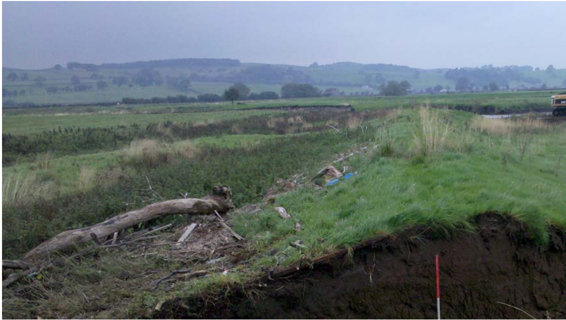
Plate 7: Cross-section through embankment 105 , looking north
