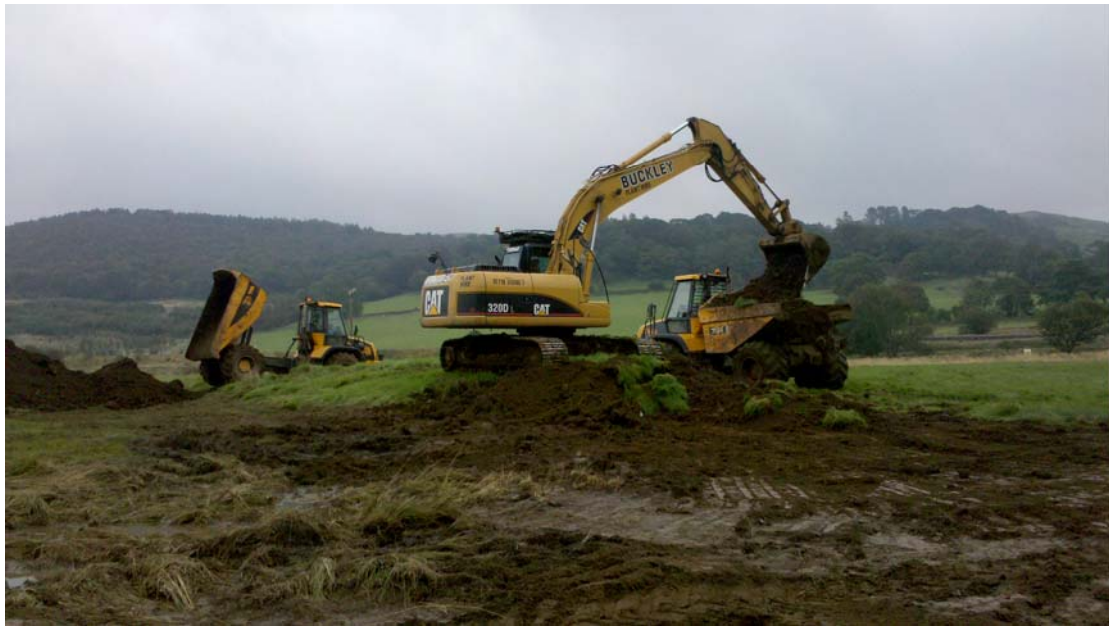
Plate 5: Embankment 103 during ground works, looking south-east
