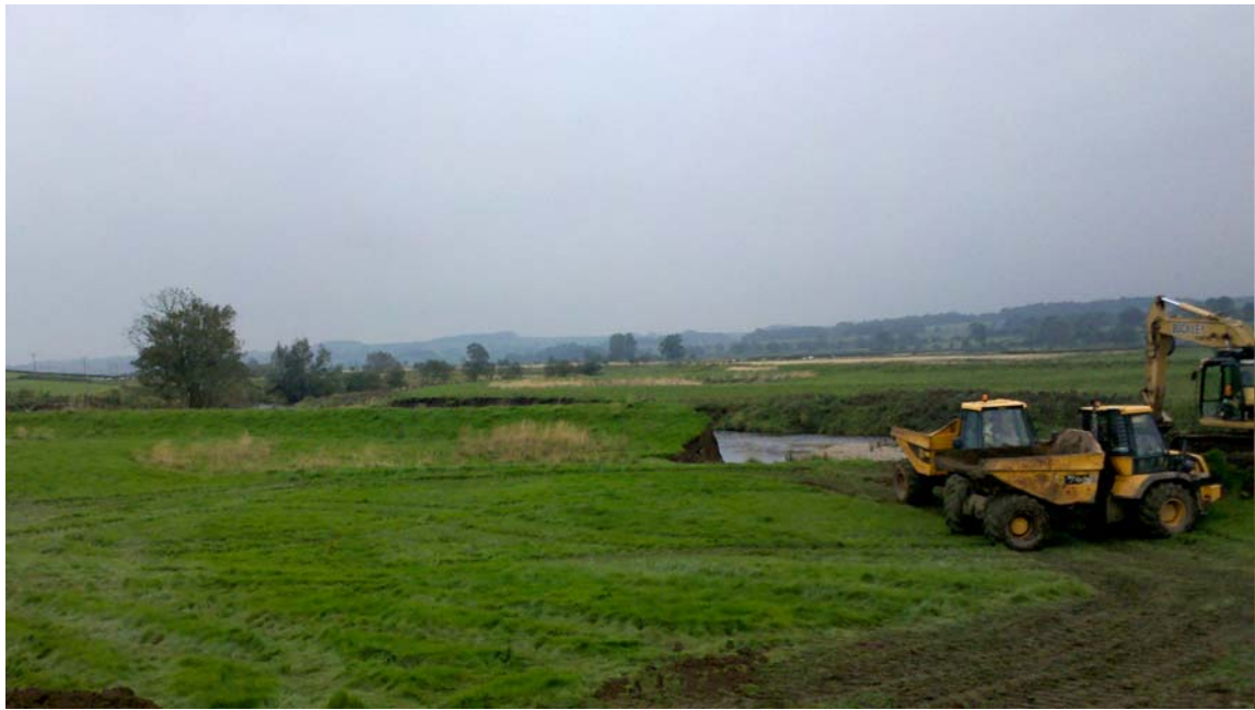
Plate 3: Embankment 105 , looking south-west
