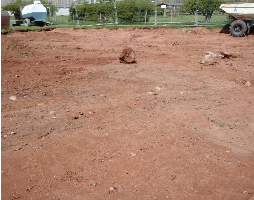
Plate 3: Phase 2 stripping, general view looking north
