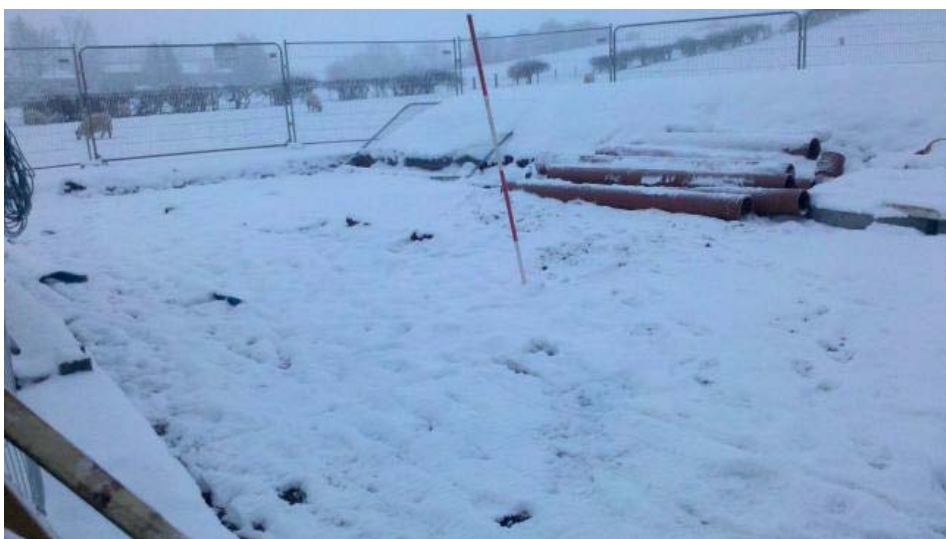
Plate 1: Phase 1, general view of the stripped area illustrating the harsh weather conditions
