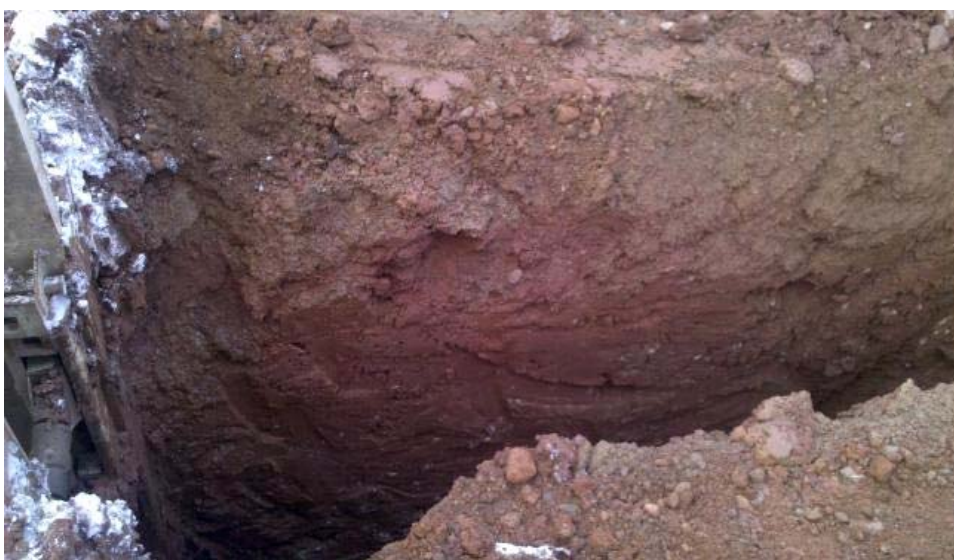
Plate 2: Phase 1, south-facing section through the pipe-trench
