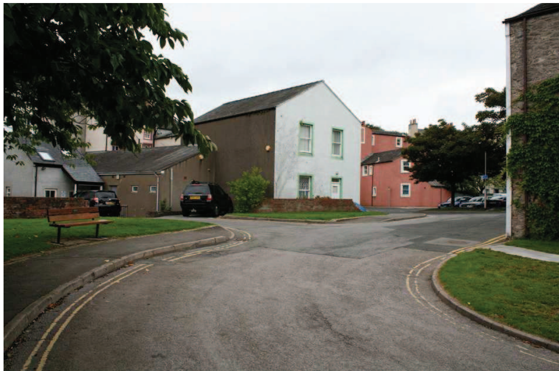
Plate 21: Area of proposed flood wall and gate on Market Place, looking north-east
