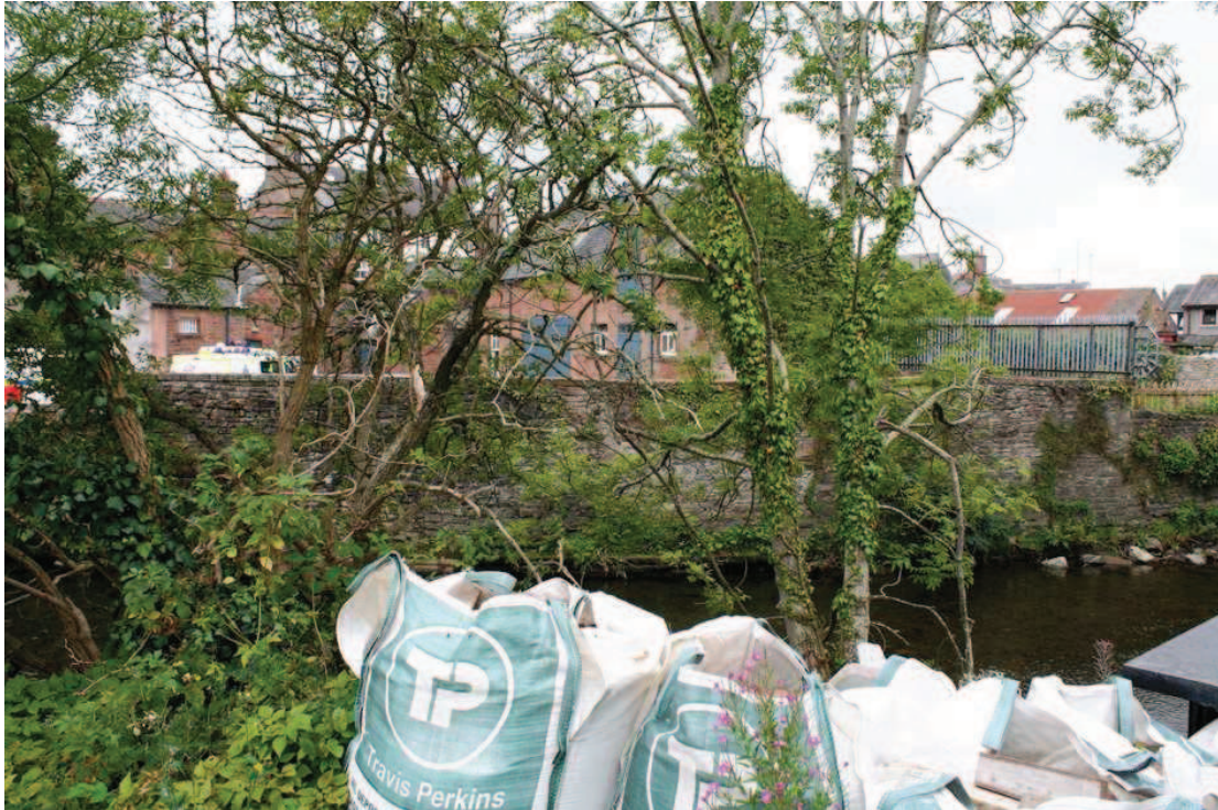
Plate 16: Flood wall to the rear of listed building, no 2 Main Street (Site 38), looking north
