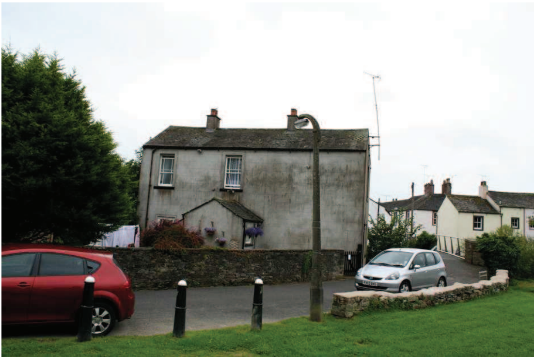
Plate 30: View of listed Foundry House (Site 37), looking south
