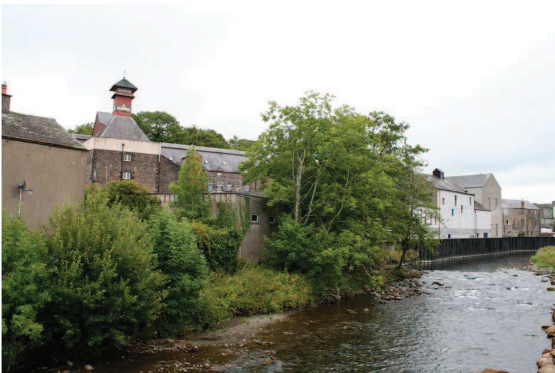
Plate 26: View of listed building (Site 33) towards emergency defence wall, looking north-east
