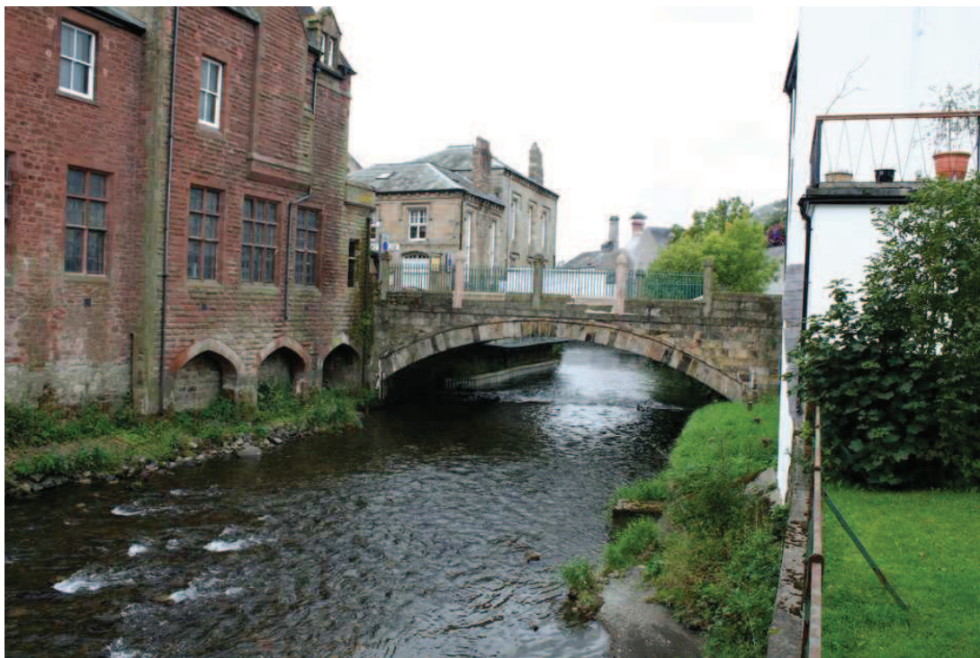
Plate 14: Bank (no 1 Main Street; Site 57), and listed Cocker Bridge (Site 34), looking north-north-west
