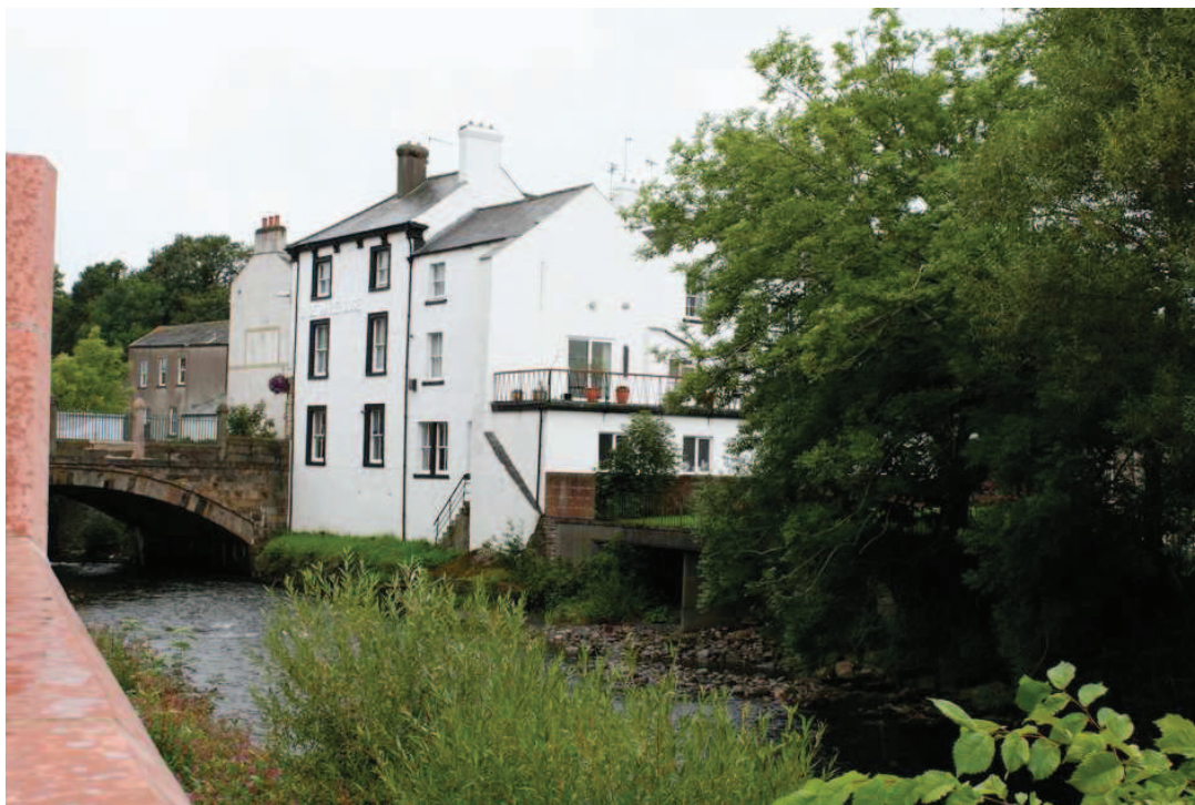
Plate 23: View of nos 41-43 Market Place (Site 59) and Cocker Bridge (Site 34) from south side of river, looking north-east
