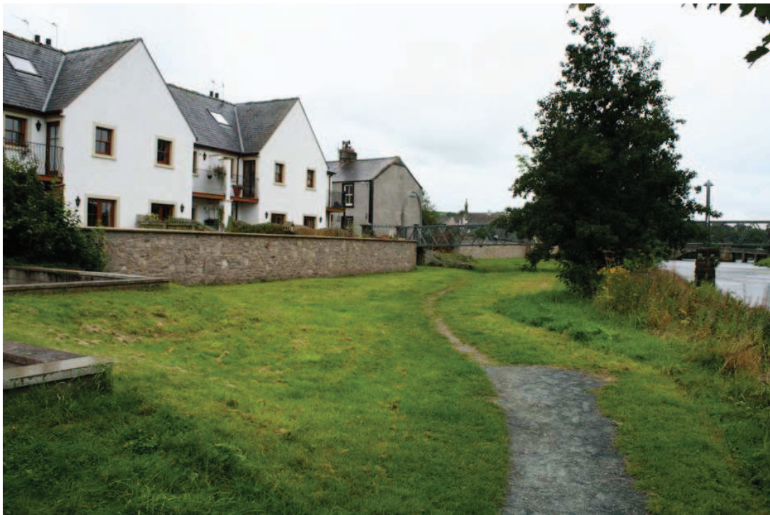
Plate 42: Existing flood defences at nos 1-3 Bridge Street Close, looking south-west
