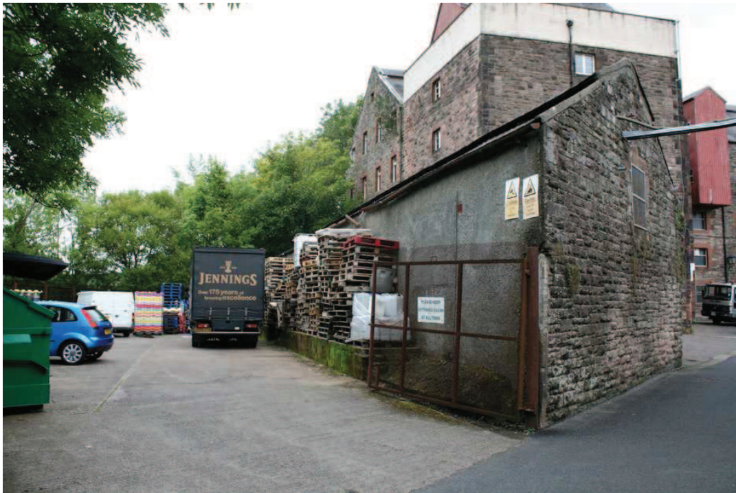
Plate 29: View of unlisted brewery building proposed to be flood proofed, looking north-east
