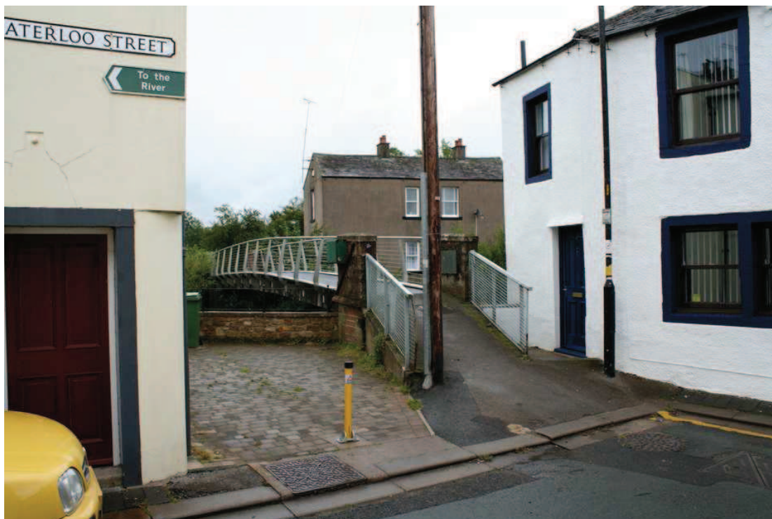
Plate 33: View of no 7 High Sand Lane (Site 60) and area of proposed floodgate, looking north-east
