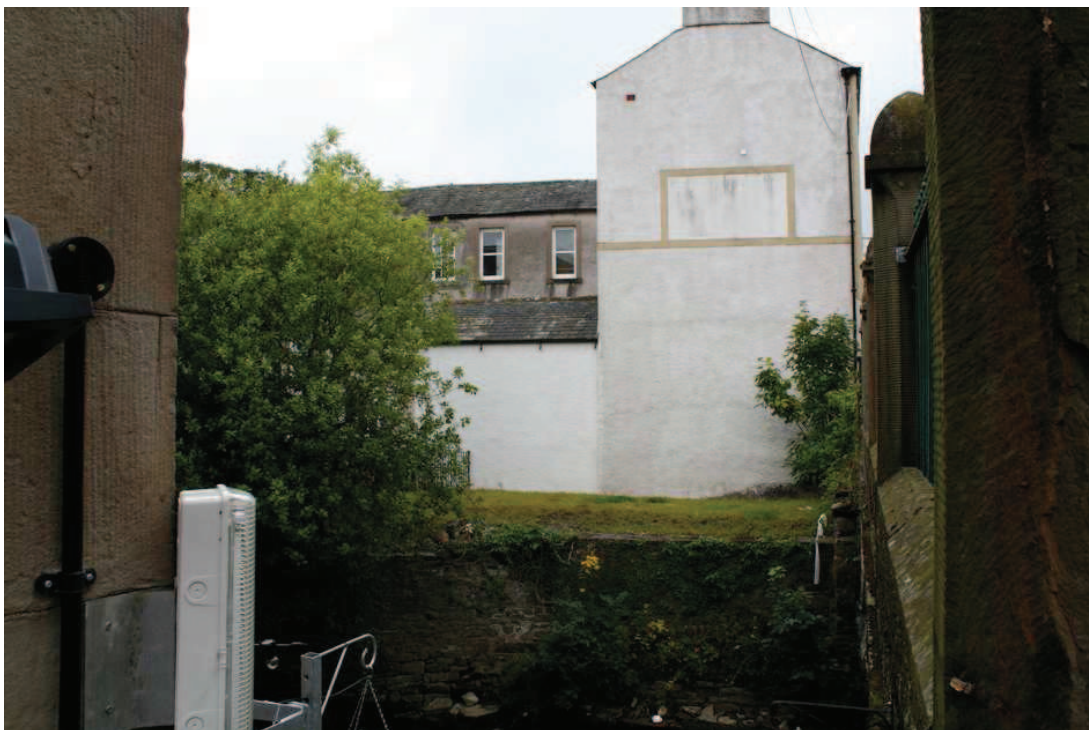
Plate 15: View of listed building (Site 42) on north-east side of Cocker Bridge (Site 34), looking east
