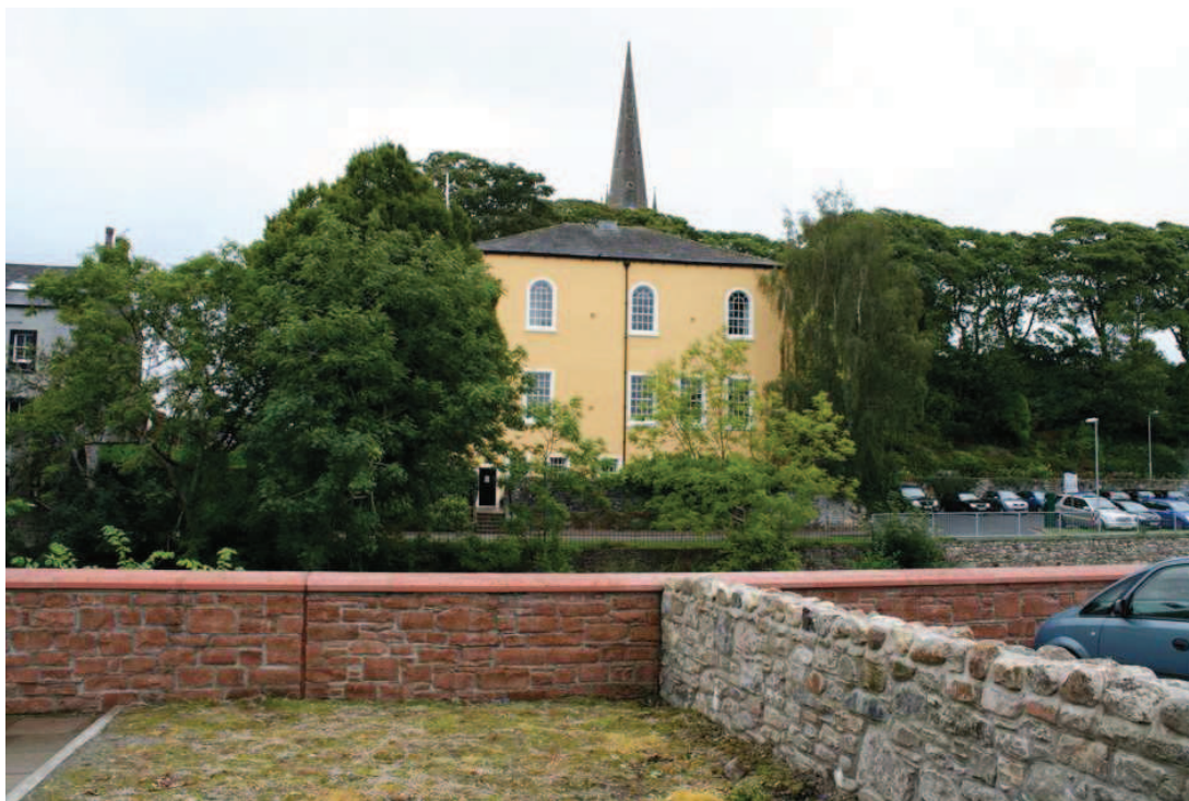
Plate 10: View over emergency flood wall to listed Town Hall (Site 41), looking east
