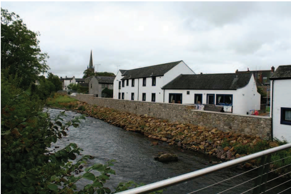
Plate 31: Area of emergency defence wall, looking south-east
