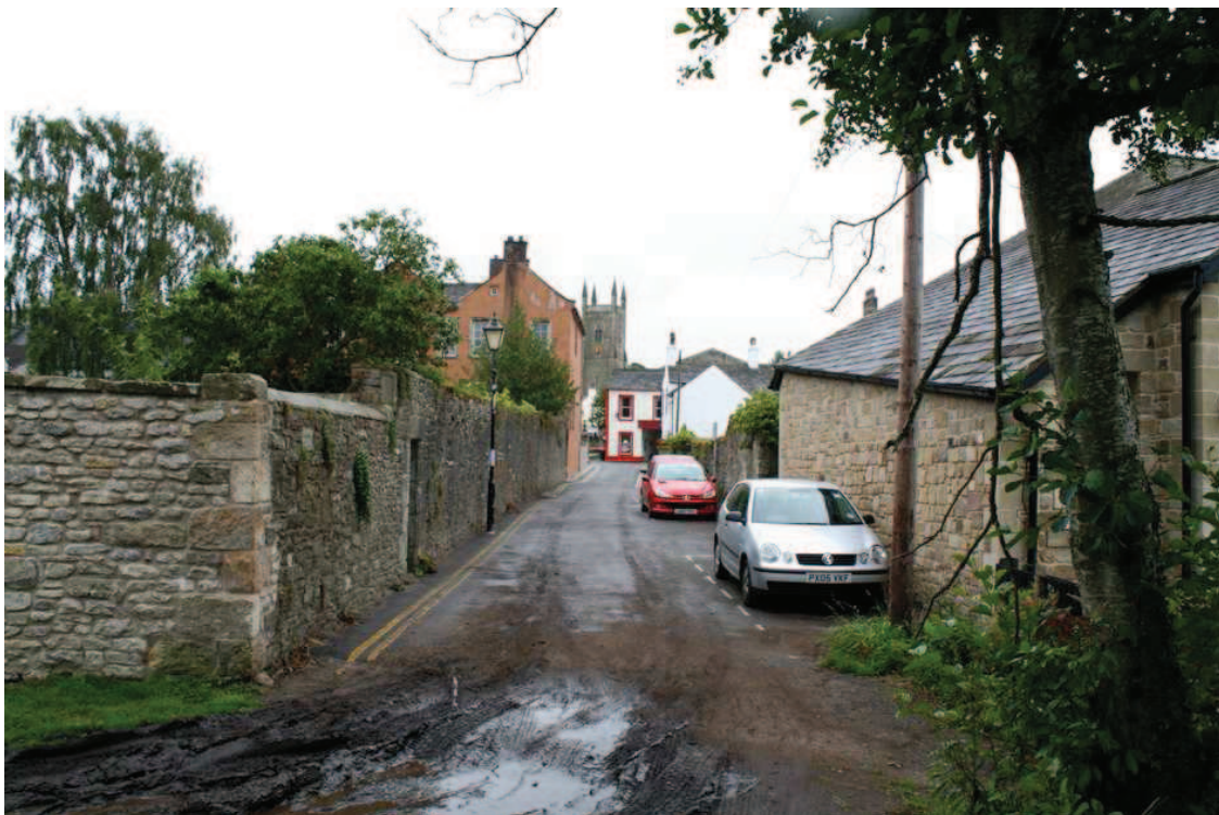
Plate 45: View from proposed Low Sand Lane floodgate, looking south
