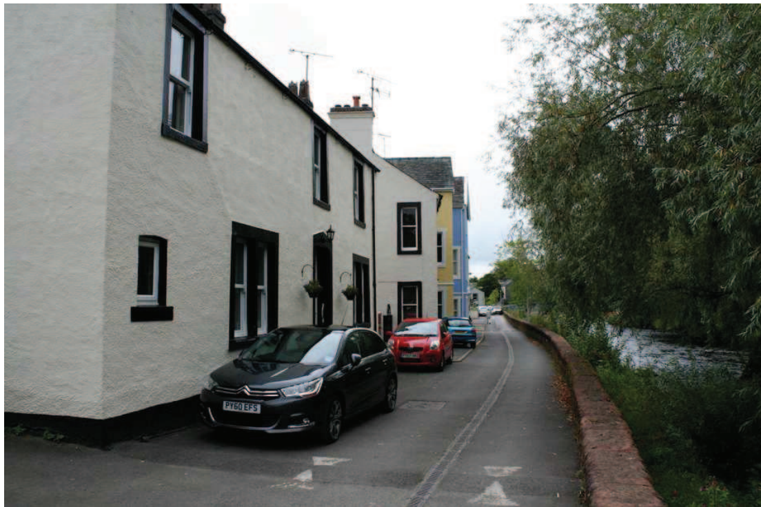
Plate 5: Rubby Banks Road, looking north
