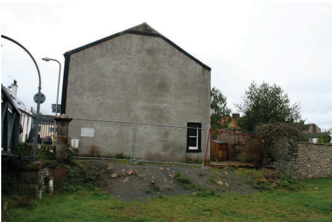
Plate 44: Damaged wall north of no 2 Bridge Street, looking south
