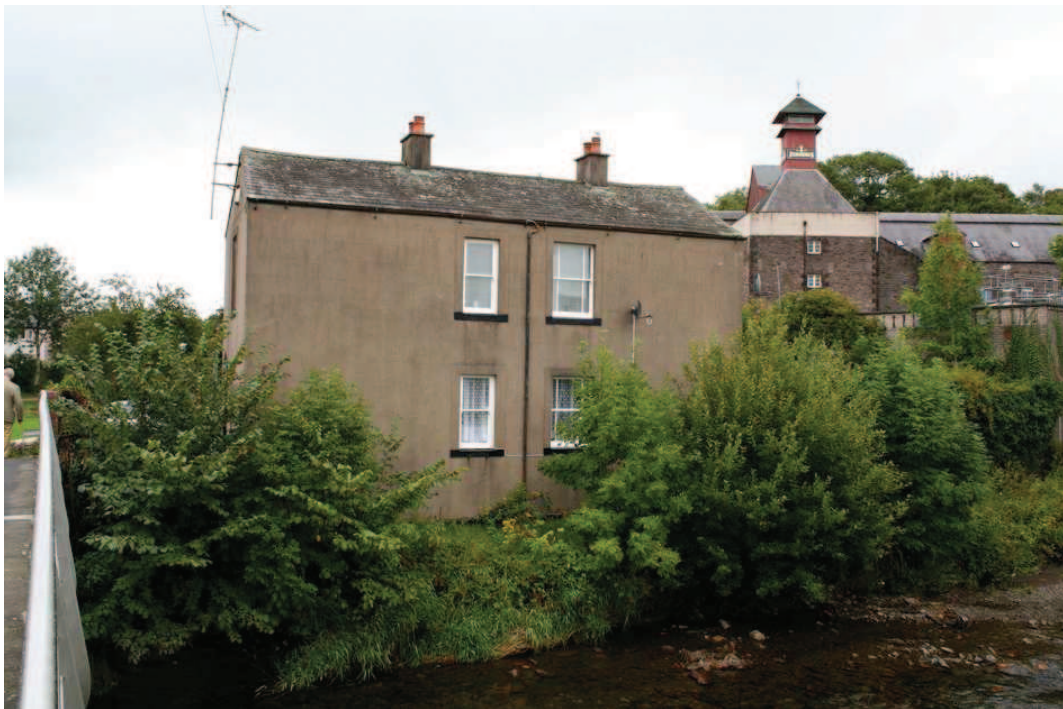
Plate 27: View of listed Foundry House (Site 37), looking north-north-east
