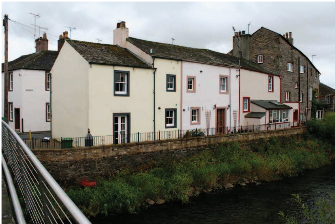
Plate 34: View of nos 19-23 Waterloo Street, looking south-west
