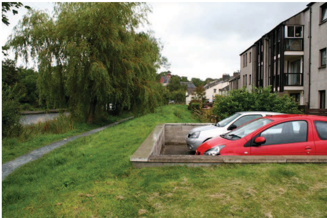
Plate 39: View of area of proposed flood defence wall north of Waterloo Street, looking east
