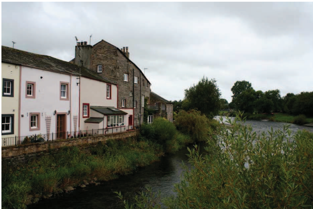
Plate 35: View of Wharton Mill, looking west-south-west
