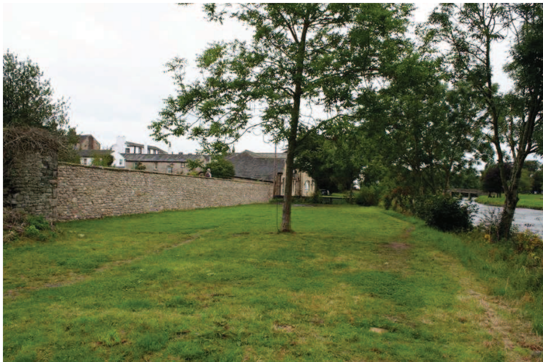
Plate 43: Existing flood defences at Wordsworth house (Site 19), looking south-west
