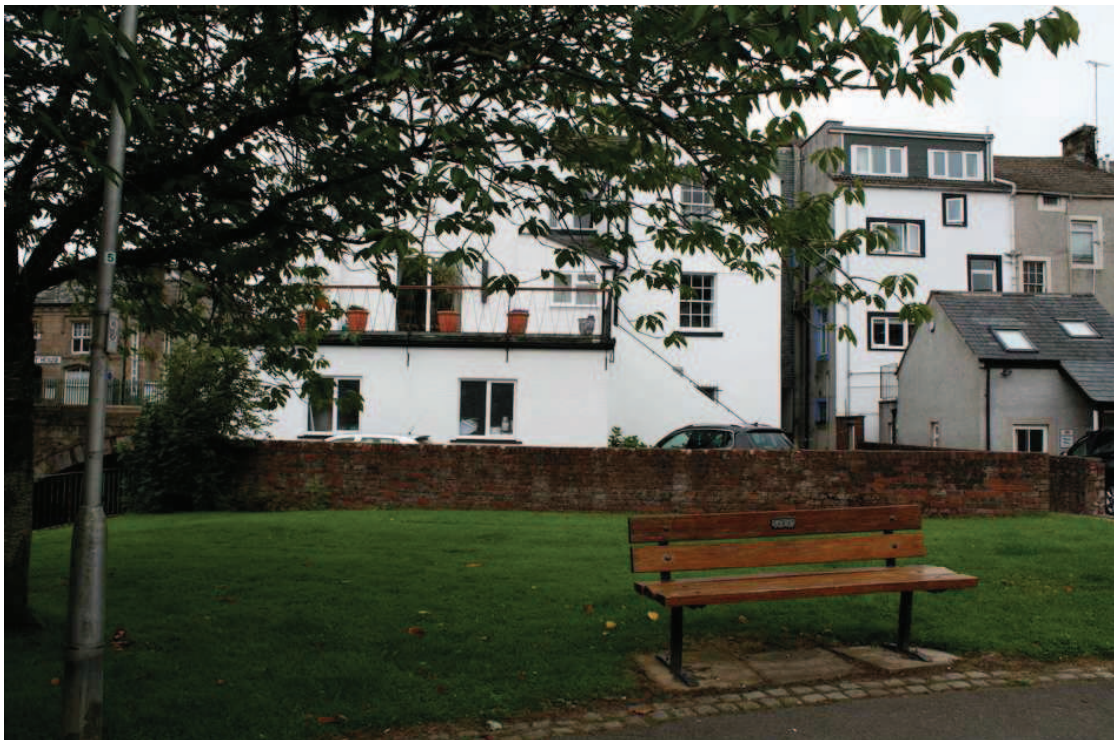
Plate 20: Existing flood wall behind nos 41-43 Market Place (Site 59), looking north
