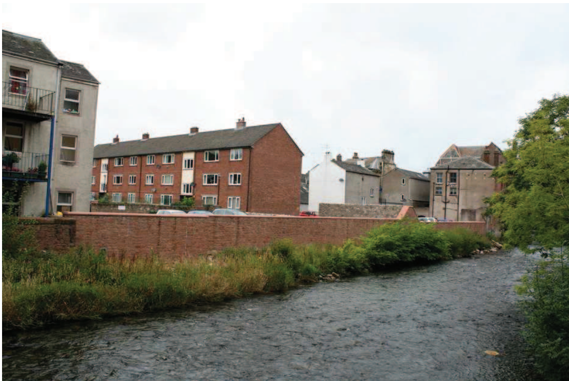
Plate 9: Emergency flood wall north of Hatter's Croft (Site 35), looking north-west
