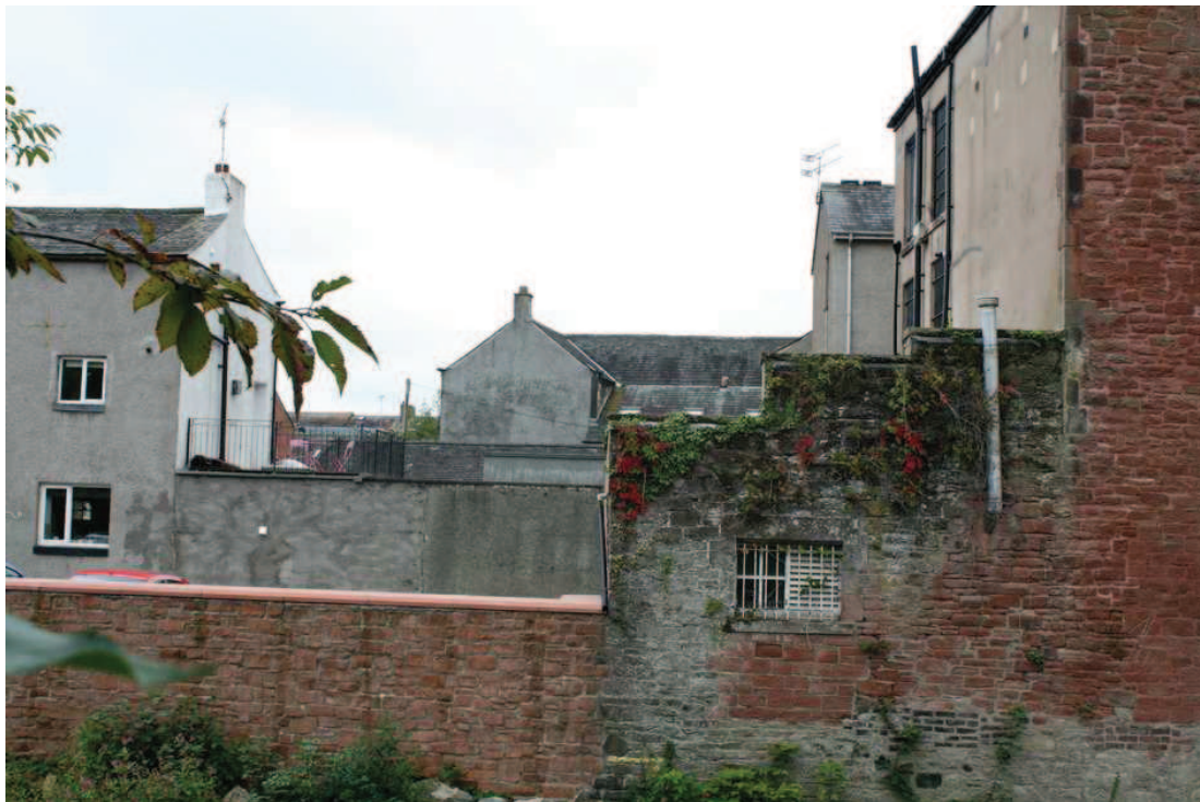
Plate 11: Rear of bank (no 1 Main Street; Site 57) and emergency flood wall, looking west
