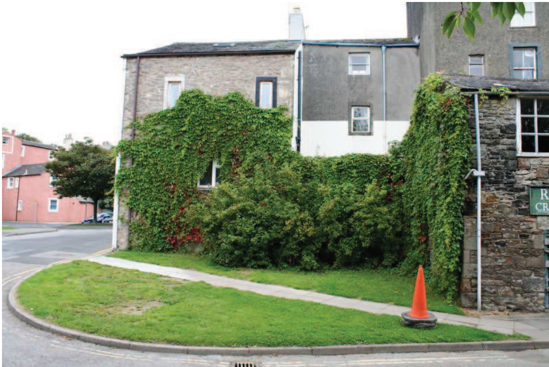
Plate 18: View of nos 6-8 Market Street, looking east
