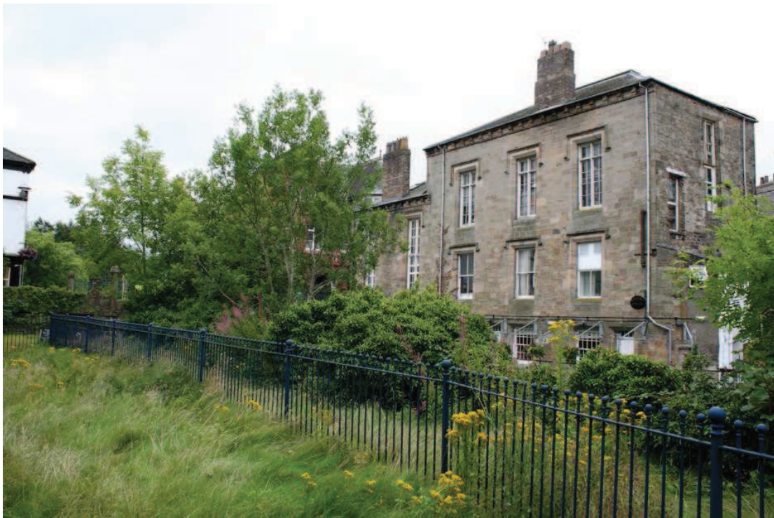
Plate 12: View of listed no 2 Main Street (Site 38), looking south-west
