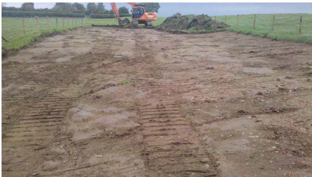
Plate 2: A portion of the pipeline easement following the removal of topsoil
