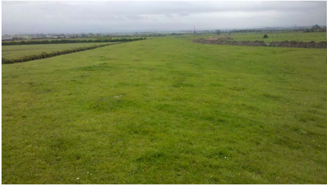
Plate 4: The raised linear embankment of the former Kirtlebridge, Annan, and Brayton Branch Railway
