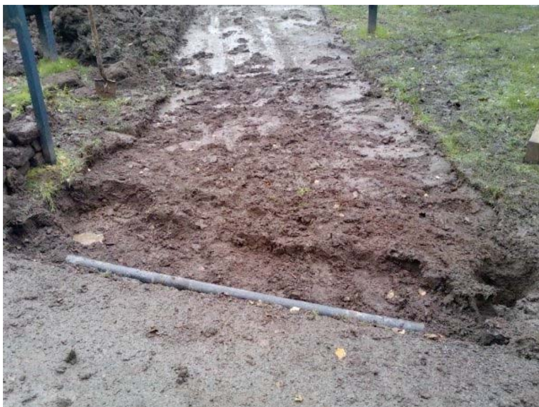
Plate 3: View of the access path following removal of the cobbles and installation of the pipe
