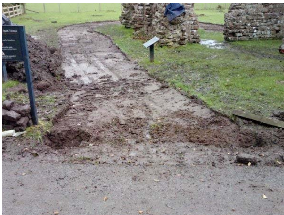
Plate 4: View of the wet conditions along the excavated pathway
