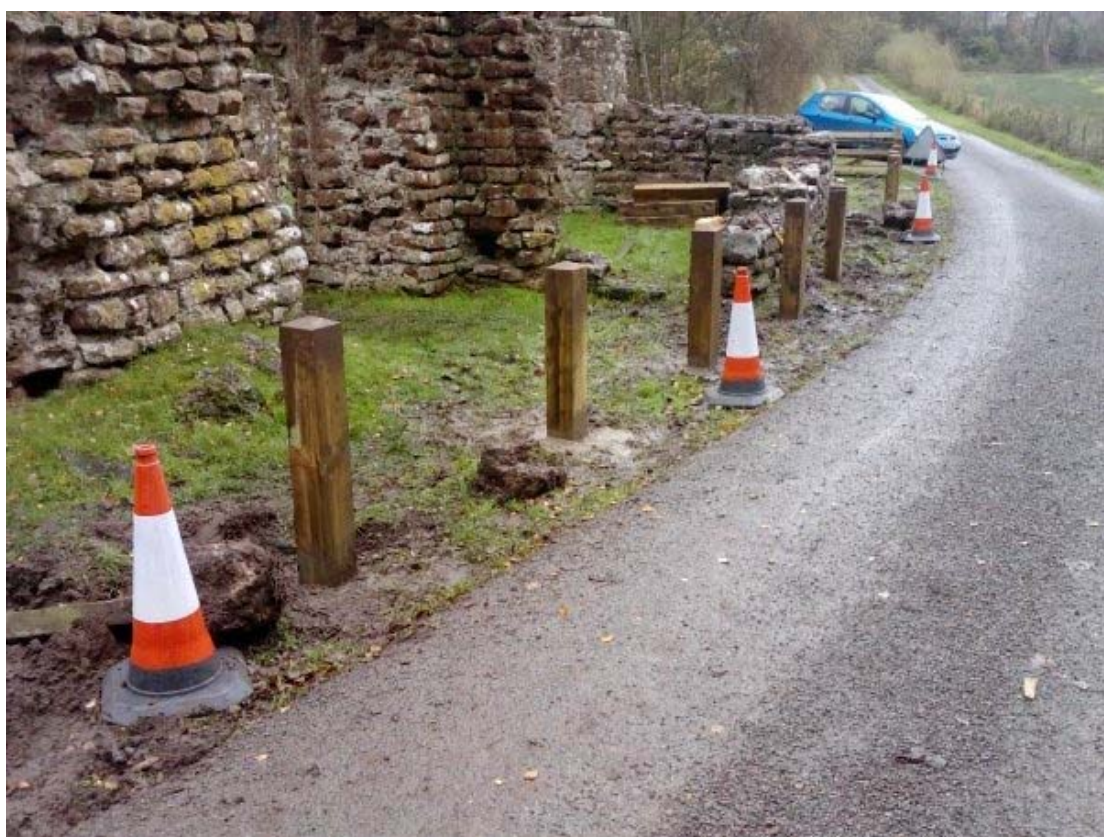
Plate 2: Bollards on roadside
