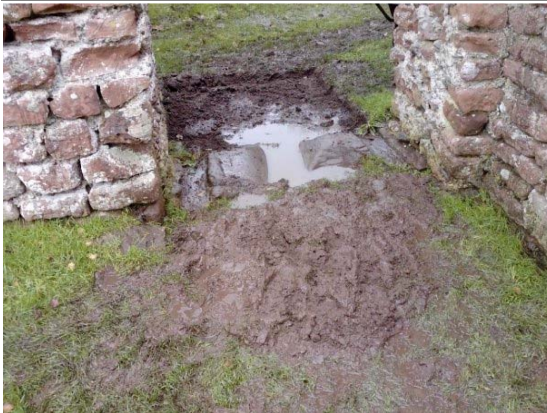
Plate 5: View of one of the doorways that has been excavated on one side and levelled up on the other side prior to the laying of the strengthening mesh
