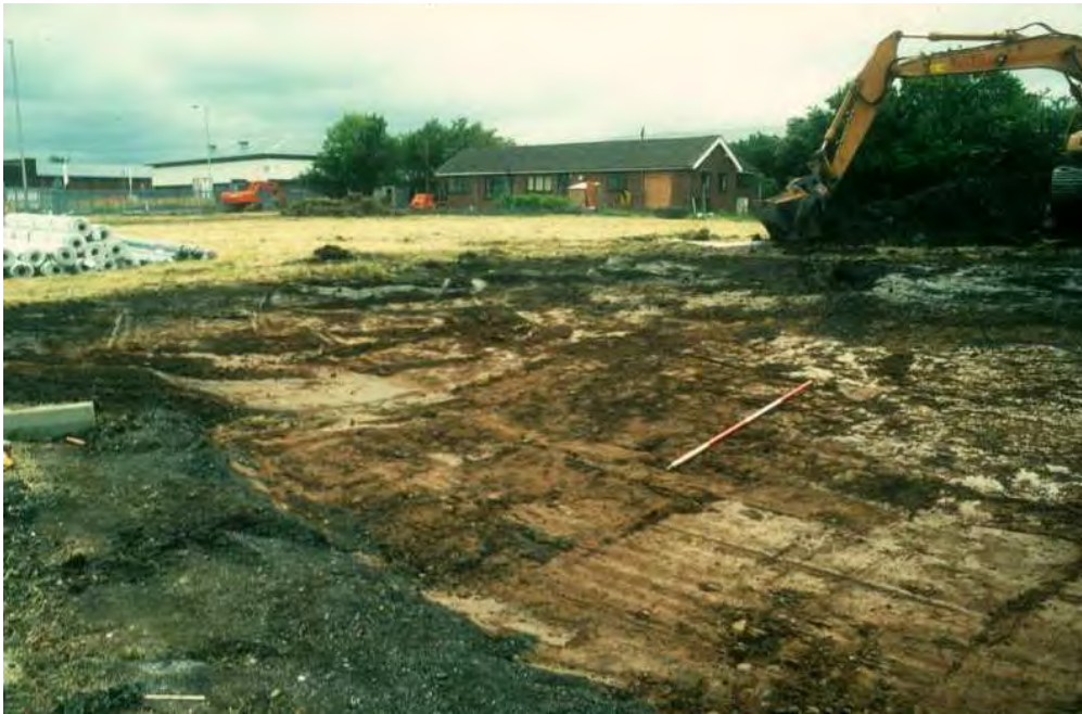
Plate 1: General view of the site during topsoil stripping
