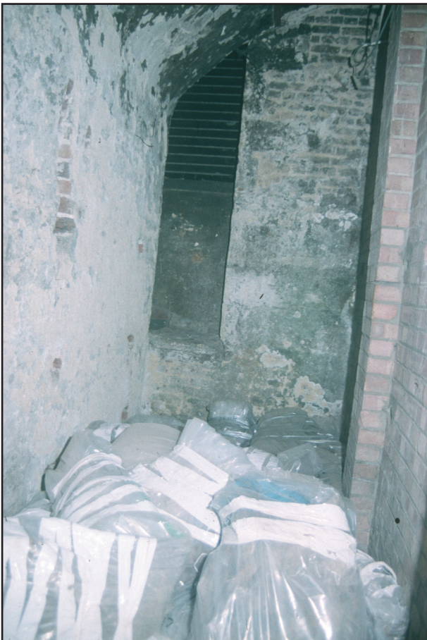
Plate 2.23: Vault 7 looking north
