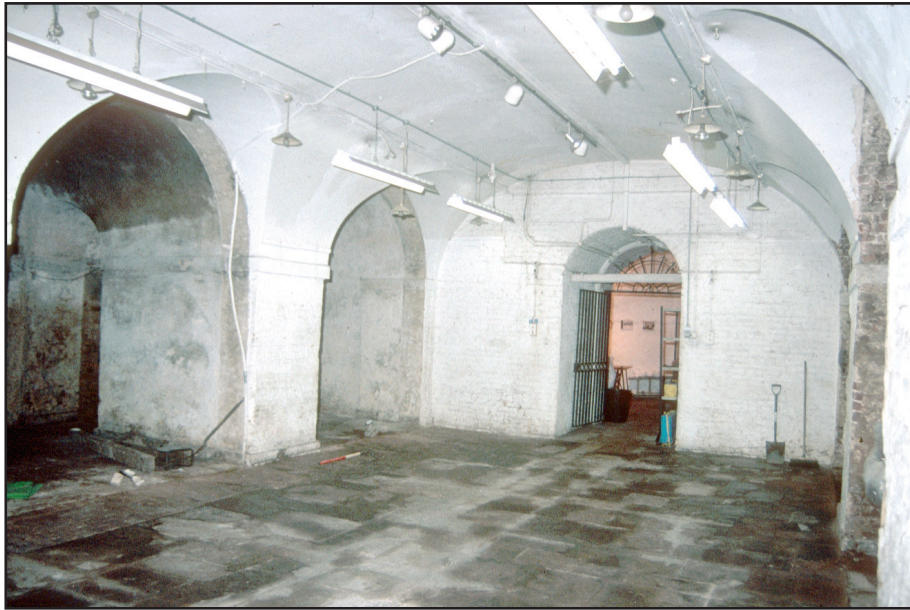
Plate 2.1: Main central vault looking south
