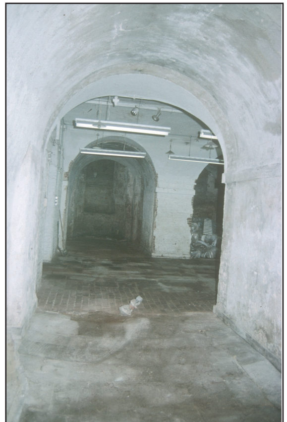
Plate 2.12: Vault 3 looking west
