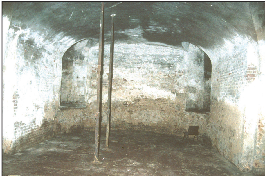
Plate 2.5: Vault 1 looking east
