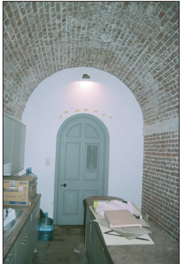
Plate 2.24: Vault 8 looking east
