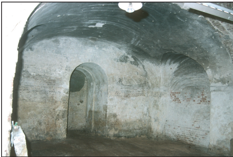
Plate 2.19: Vault 6 looking north-west
