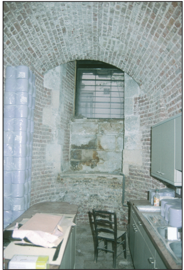
Plate 2.22: Vault 8 looking west
