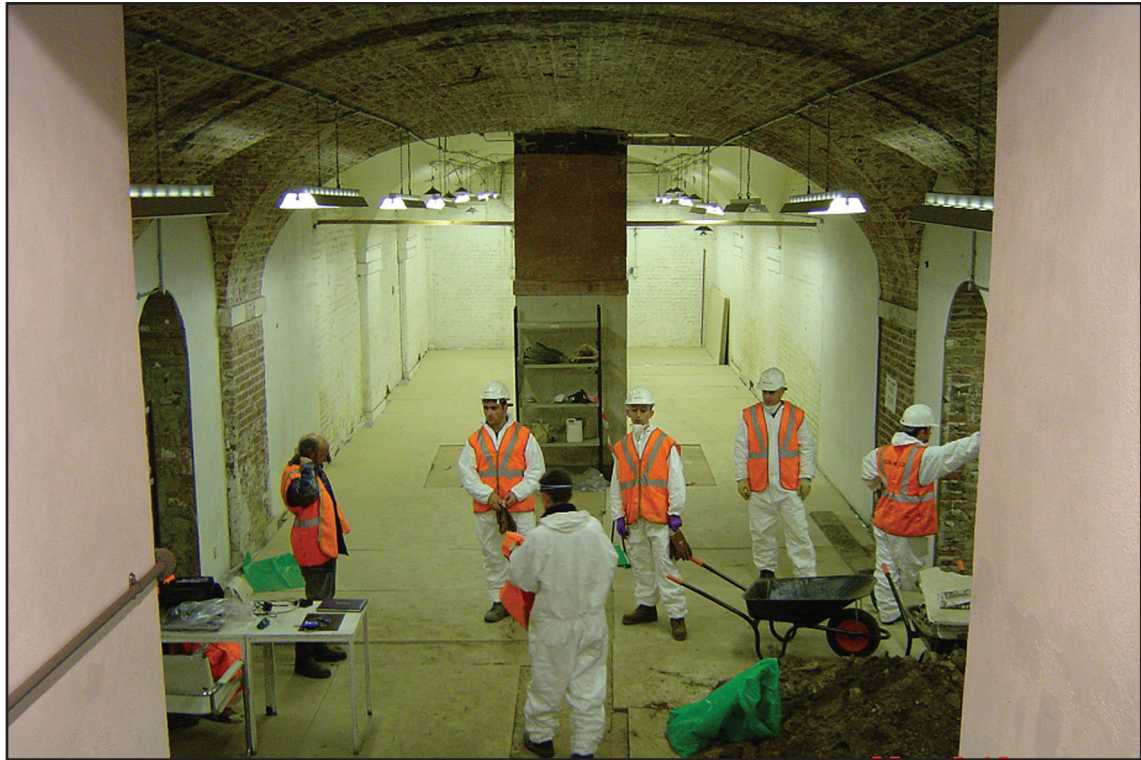
Plate A.1: The crypt before work commenced
