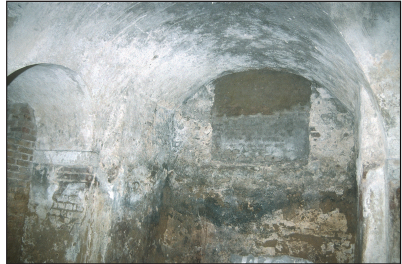
Plate 2.18: Vault 5 looking west
