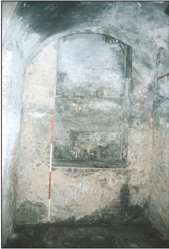
Plate 2.9: Vault 2 looking east
