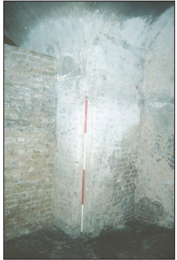
Plate 2.10: Vault 2 looking north-east
