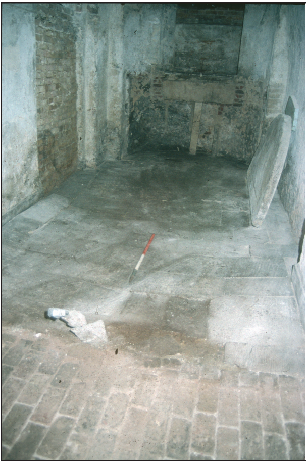
Plate 2.13: Floor of Vault 3 looking east
