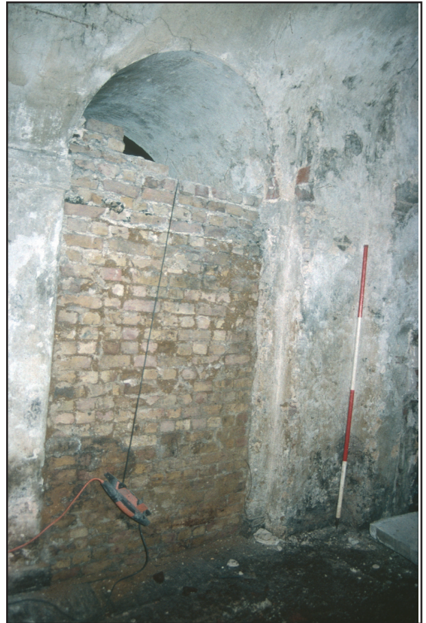
Plate 2.14: Blocked doorway between Vaults 2 and 3. Looking north-east
