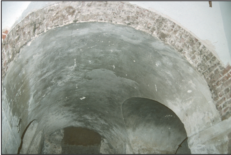
Plate 2.17: Vault 5 showing location of removed wall
