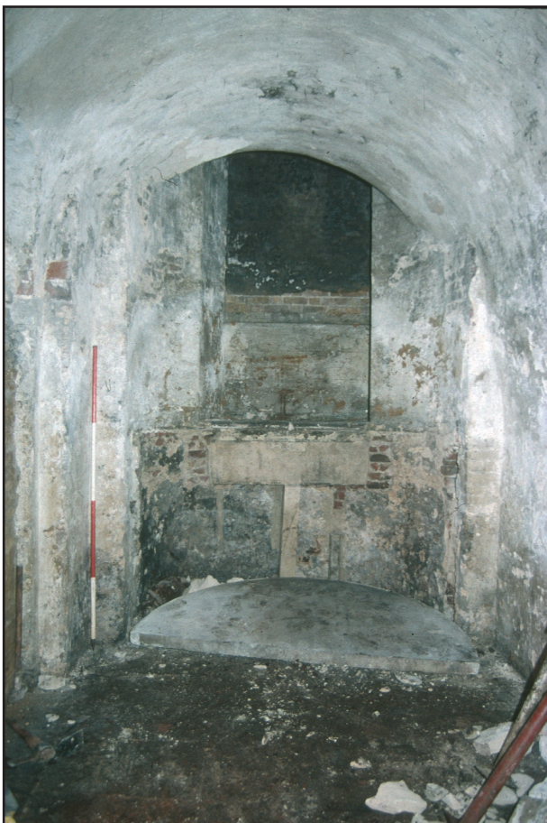
Plate 2.15: Vault 3 looking east
