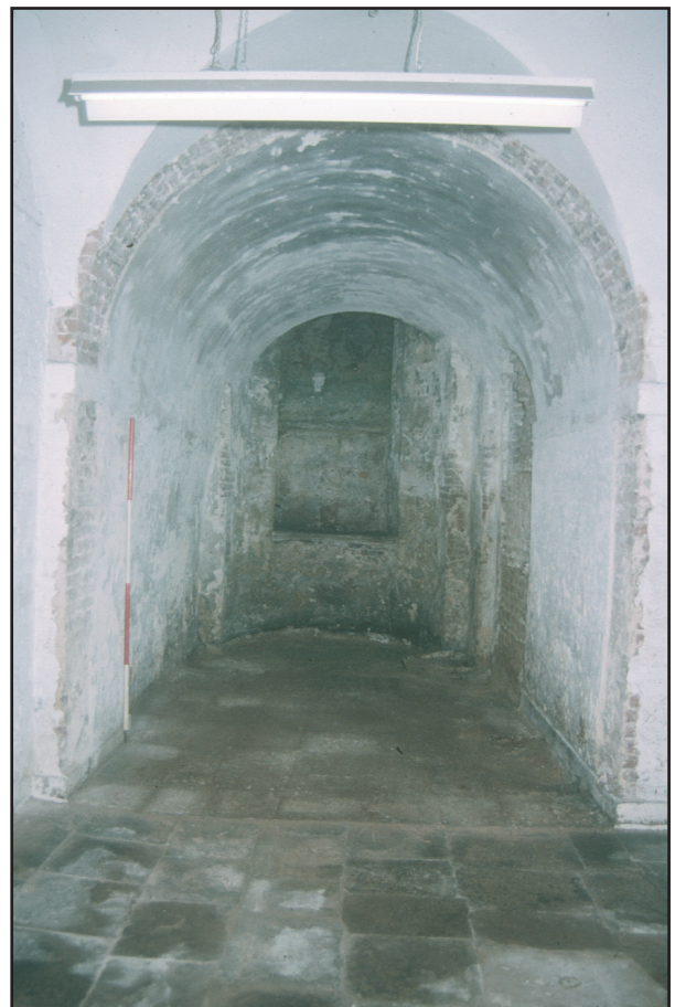
Plate 2.16: Vault 4 looking east
