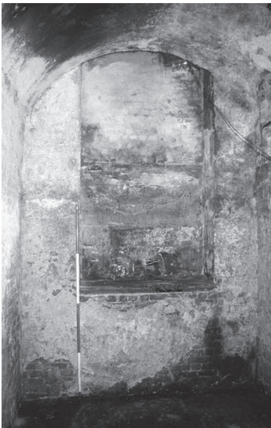
Plate 2.7 Vault 2 looking E, showing recess with raised sill and blocked window
