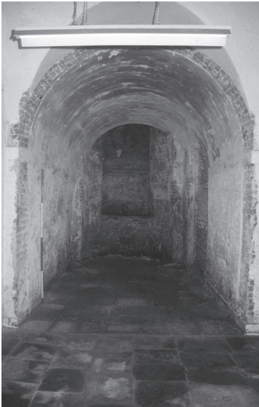
Plate 2.12 Vault 4 looking W. The skewed window recess in the apse at the end of the vault is clear
