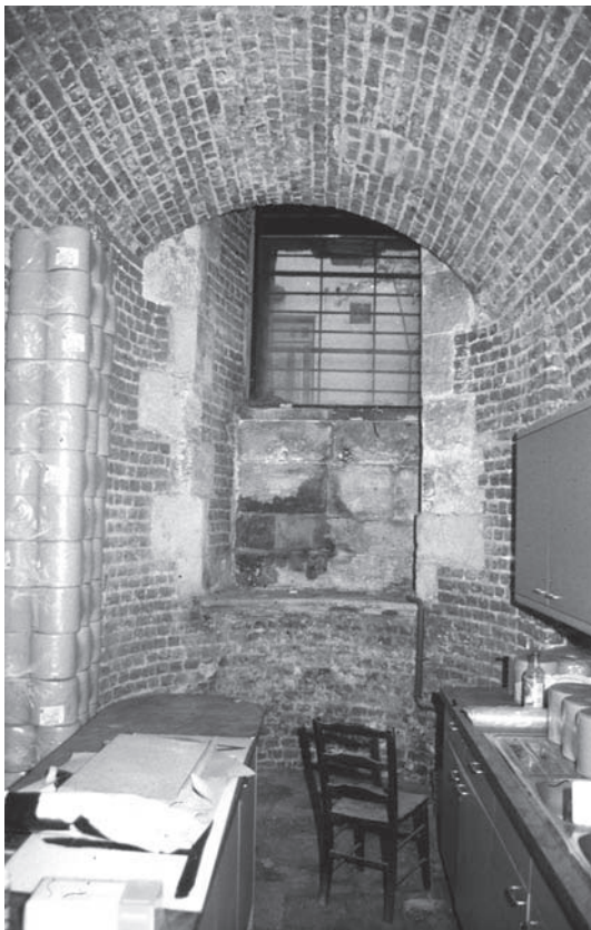
Plate 2.19 Vault 8 containing kitchen. View looking W. Note the apsidal end and skewed window opening
