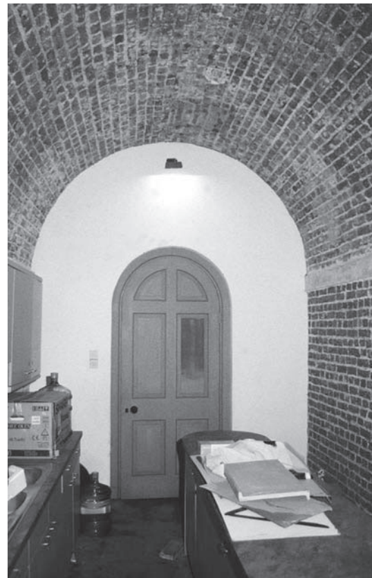
Plate 2.20 Vault 8 looking E.
