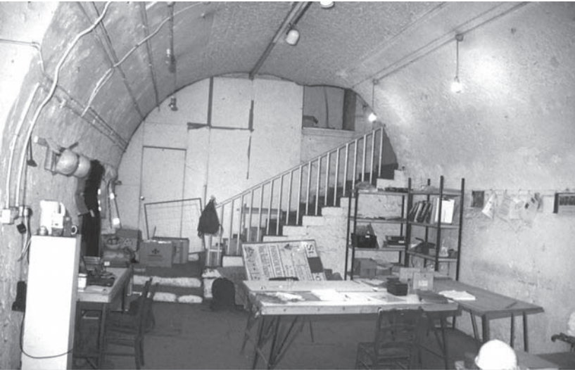
Plate 2.2 E-W Vault to the S of the main central vault of the crypt, showing one of the main stairways at the E end of the vault
