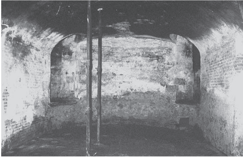
Plate 2.4 Vault 1 looking E. Note the two cast iron uprights originally designed to support the racking for coffins.
