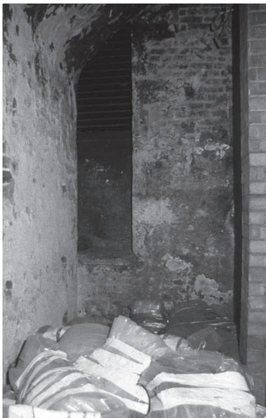
Plate 2.17 Vault 7 looking N. The original wall and vault to the left are primary, the wall to the right is a 20th-century insertion. The awkward positioning of the window at the north end of the vault is clear
