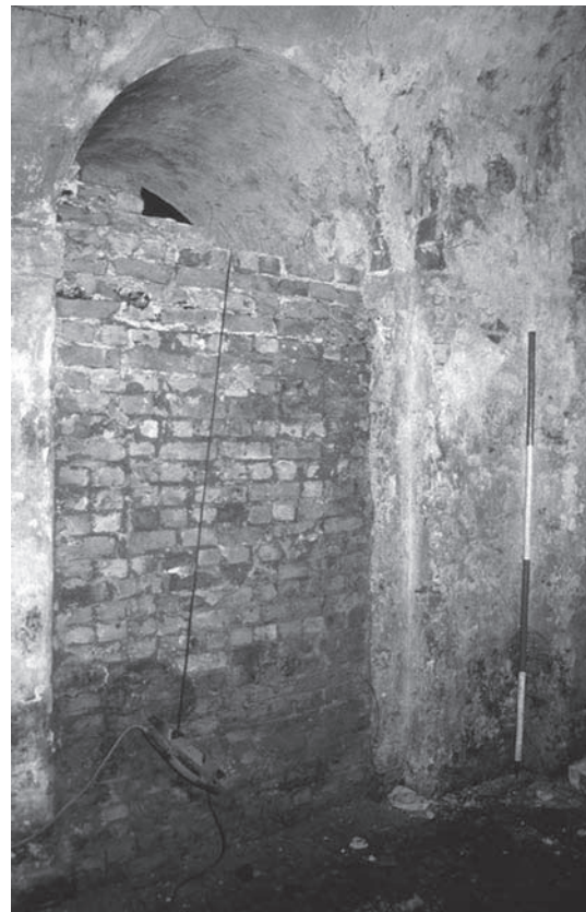
Plate 2.11 Vault 3 looking N, showing brick blocking between Vault 3 and Vault 2
