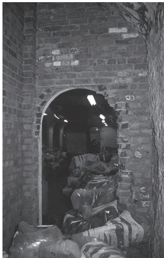
Plate 2.18 Vault 7 looking S. The S wall is built of 19th-century bricks, the E wall to the left is built of 20th-century bricks
