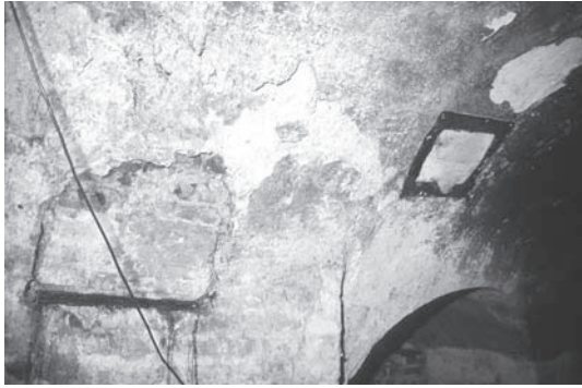
Plate 2.9 Vault 2, later features: to the left an iron bar supporting inserted brickwork, and to the right is a blocked rectilinear opening with an iron lining
