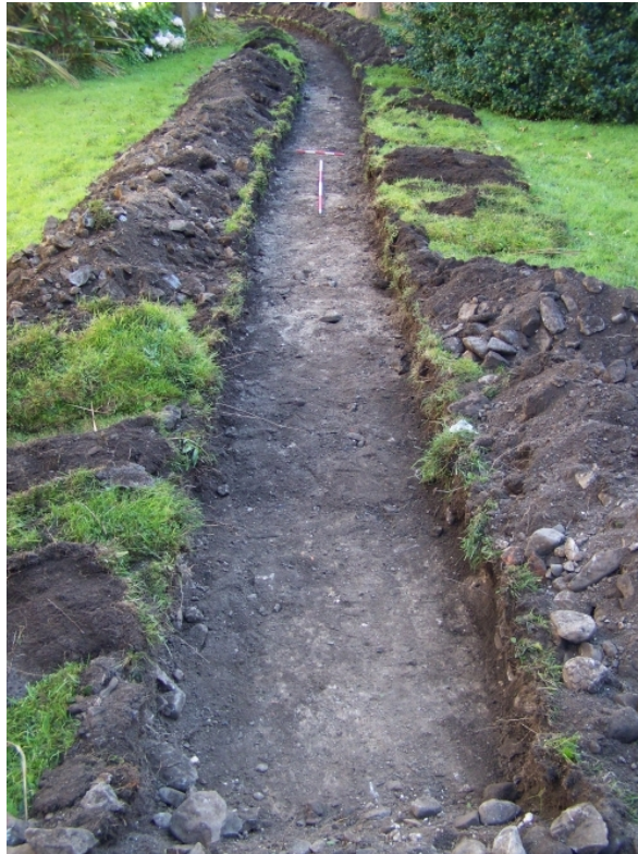
Plate 6: The north-east/south-west-aligned part of Trench 4, looking north-east
