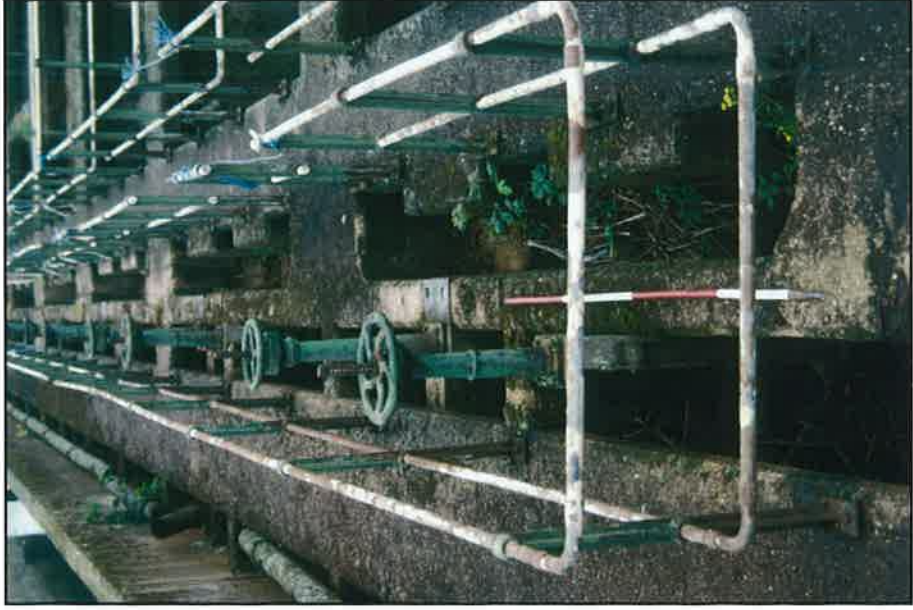
Plate 22: South view of penstocks at east
