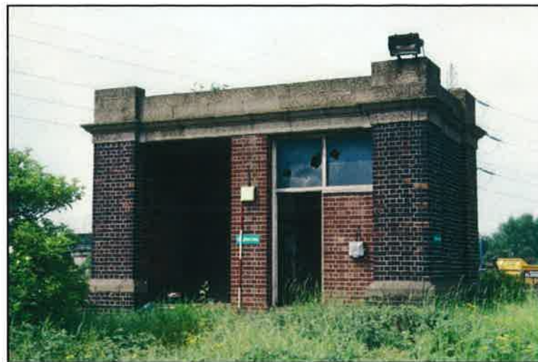
Plate 39: South-west view of Penstock Controller House
