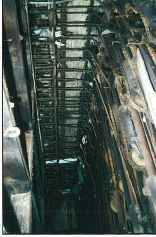
Plate 31: Internal north-east view showing the Valve House basement
