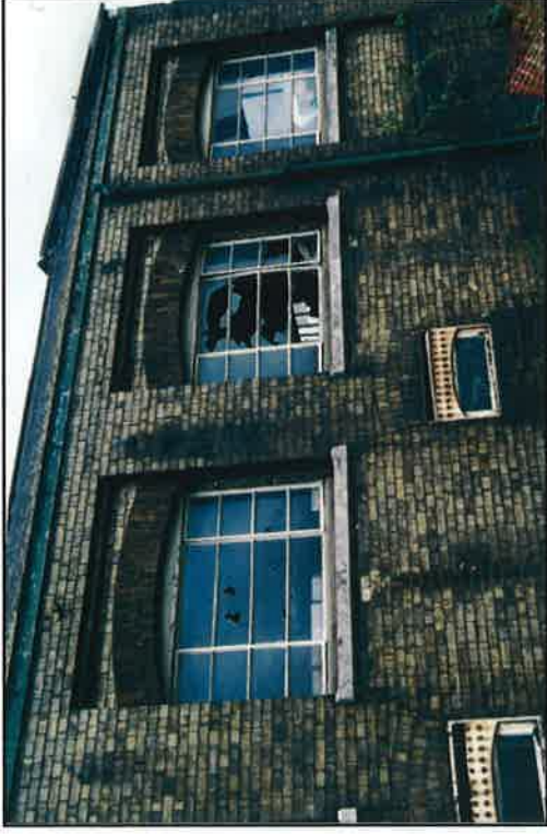
Plate 29: Valve House windows, south-west elevation
