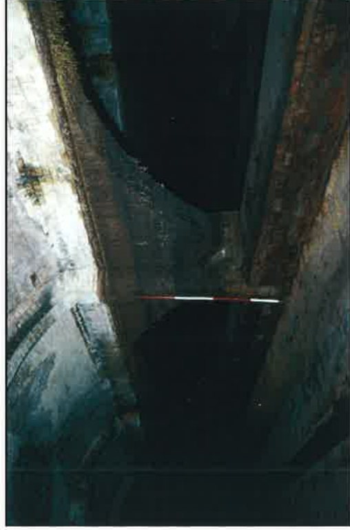
Plate 8: Internal north view of open arches dividing precipitation lanes
