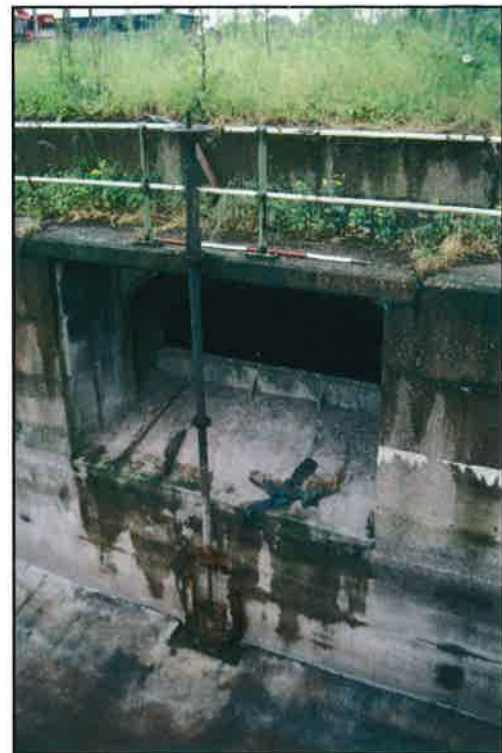
Plate 12: South-west view of weir chamber penstock
