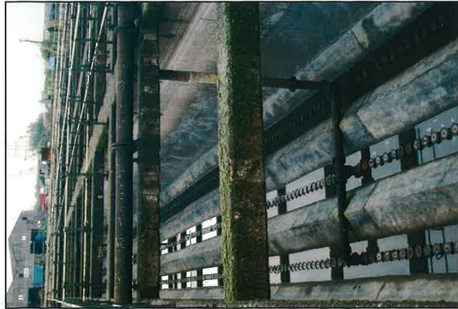
Plate 21: East view showing base of re-aeration lanes
