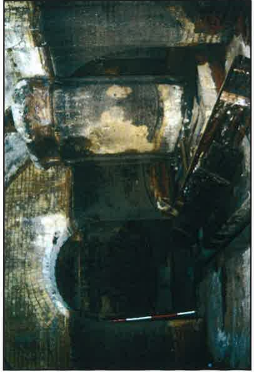
Plate 15: Box weir located at south-west termination of precipitation lanes
