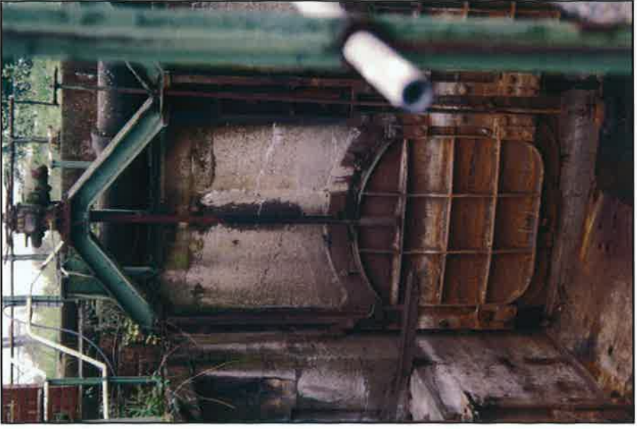
Plate 23 North view showing weir chamber penstocks
