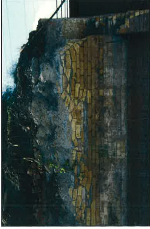
Plate 6: North view showing construction of precipitation lanes
