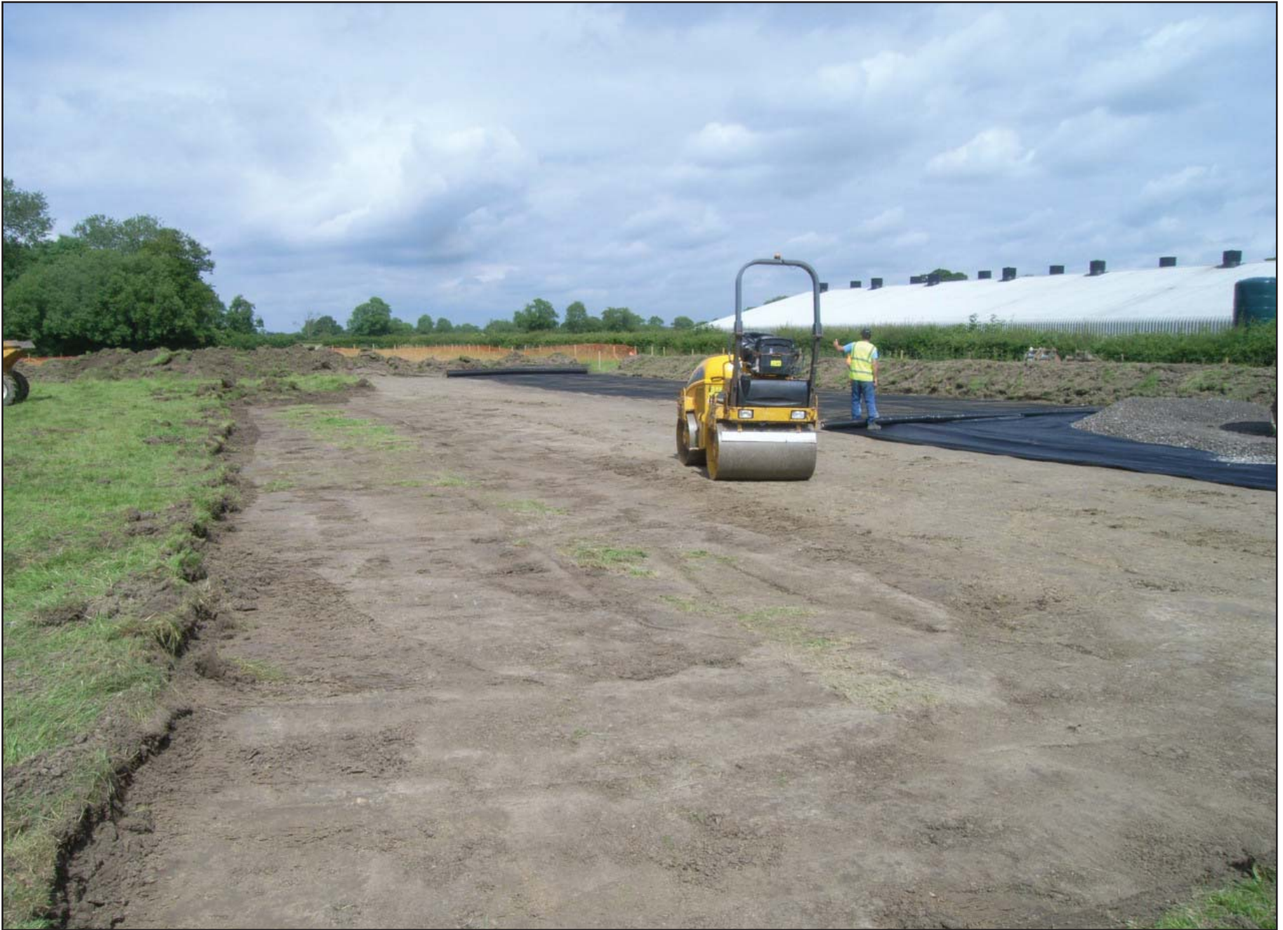
Plate 1: Compound area after stripping
