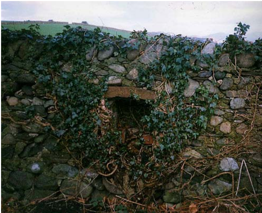
Plate 3: A Bee Bole in the garden wall at Fellgate, Strands
