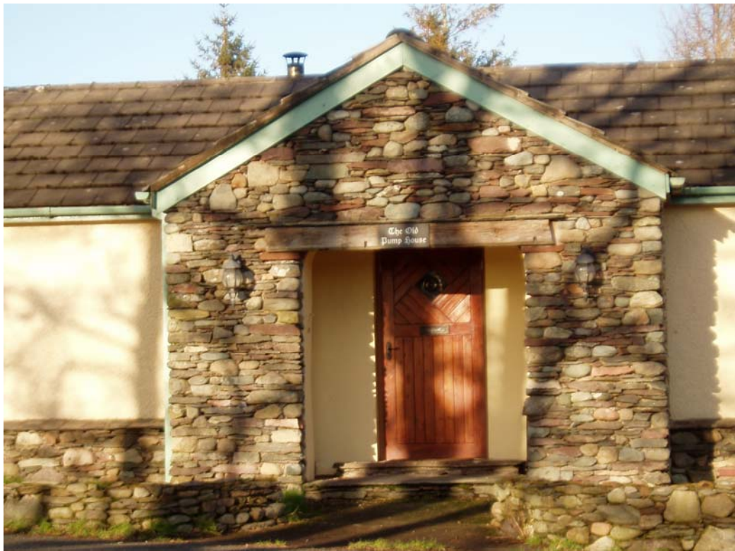
Plate 14: Residential building with slate plaque engraved “Pump House”, facing north-east.
