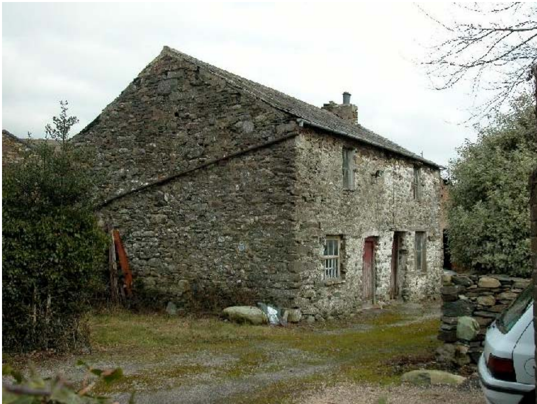
Plate 4: The workers cottages, Hallthwaites
