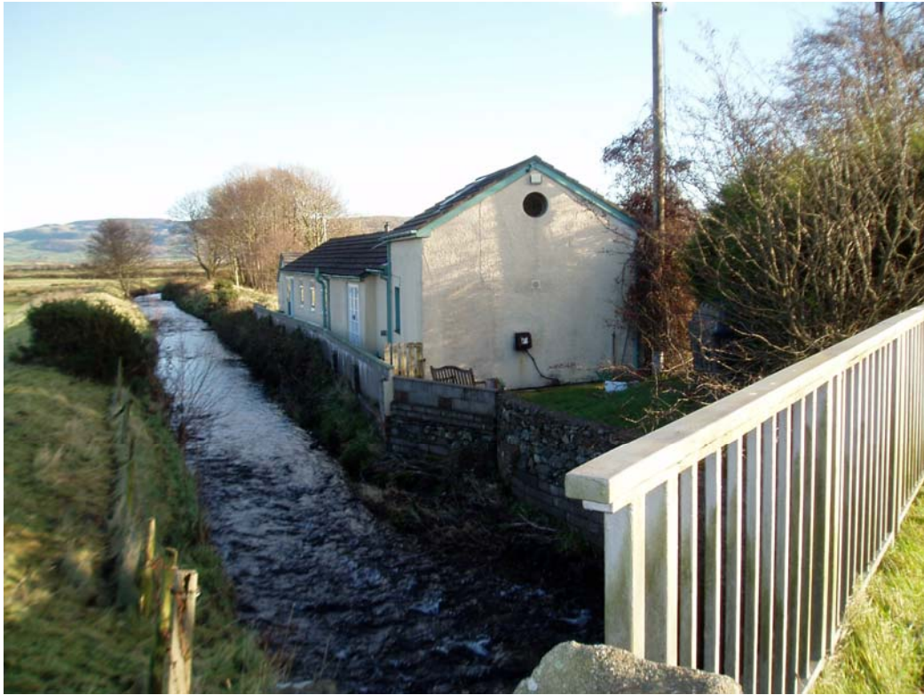
Plate 13: Probable location of Pump House (Site 14 ), facing east.
