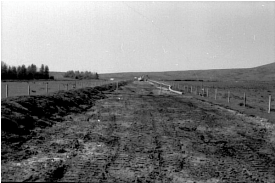
Plate 1: View of pipeline easement looking north-west
