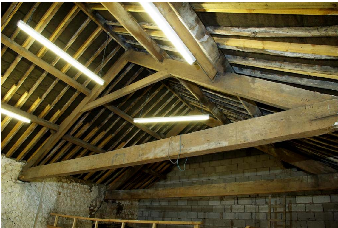
Plate 12: The roof as viewed from Room 4
