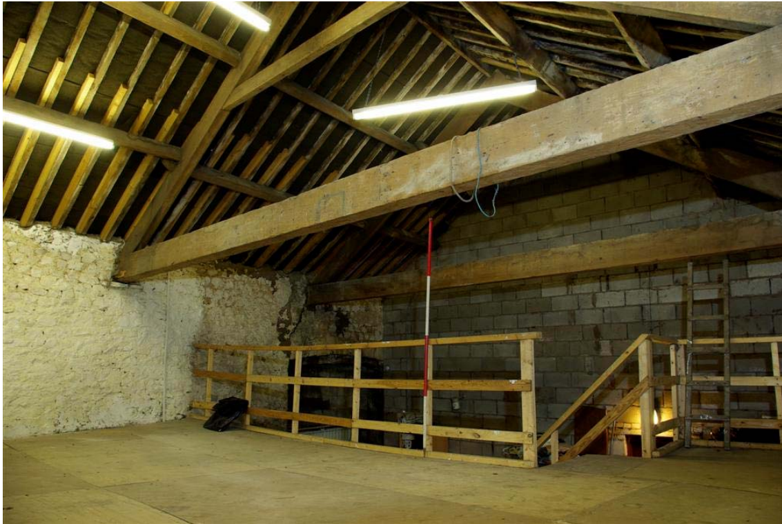
Plate 11: View of Room 4 facing west towards Room 1
