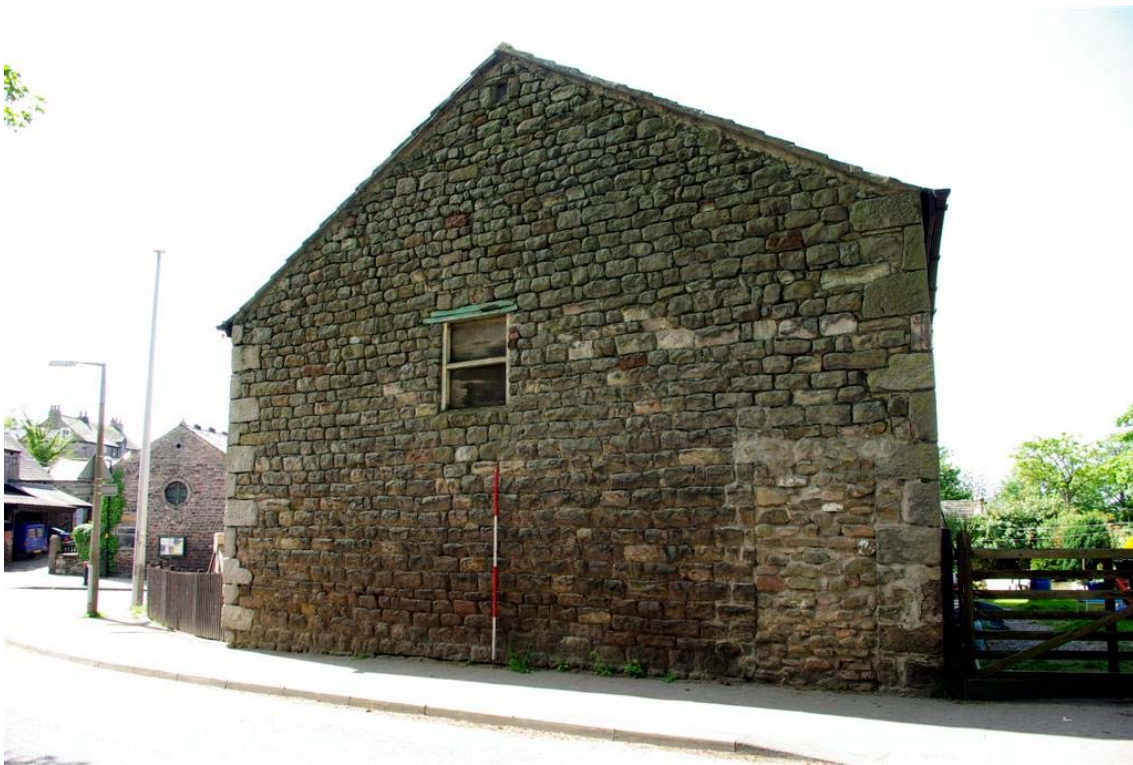
Plate 4: The east gable elevation of the barn
