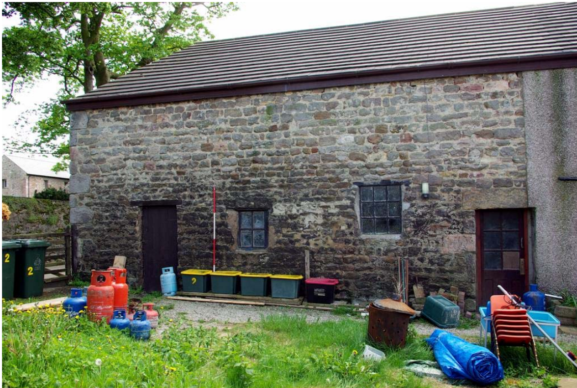
Plate 3: The north elevation of the barn
