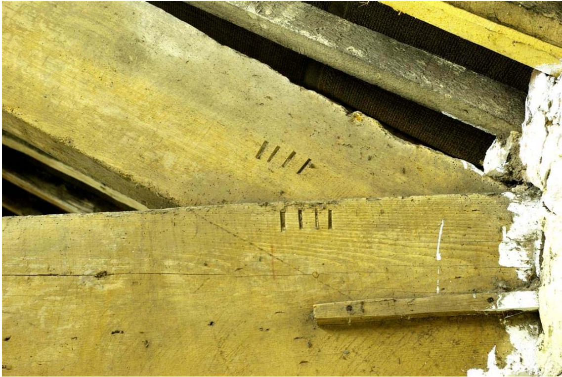
Plate 13: Example of the carpenter's marks
