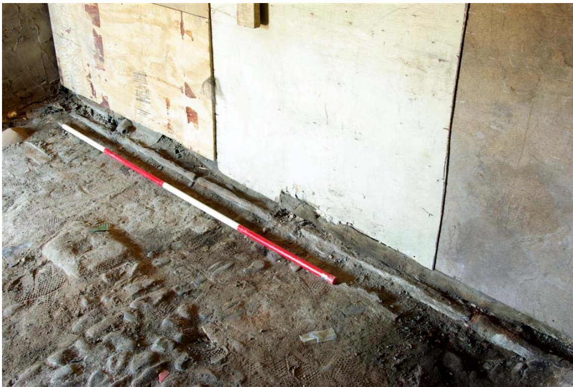
Plate 10: The stone gully in Room 2
