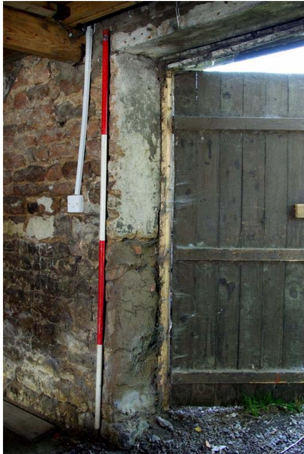
Plate 6: Doorway into Room 3 showing modified lower jambs
