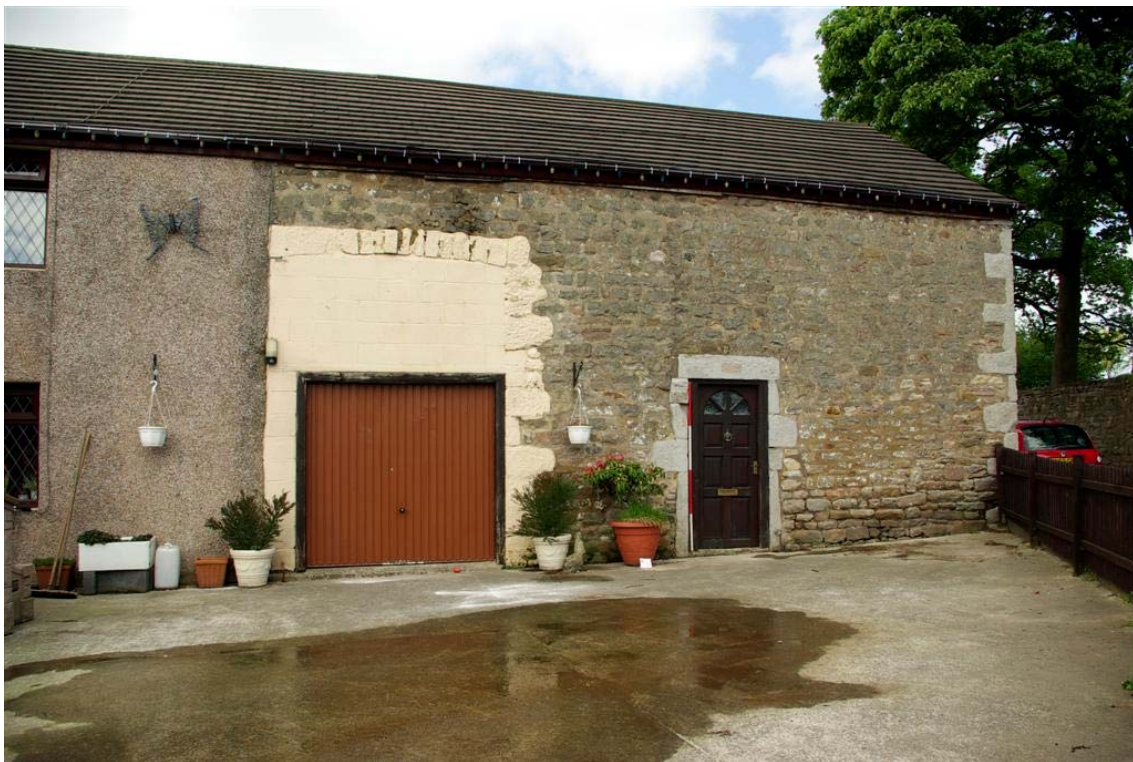
Plate 2: The south elevation of the barn
