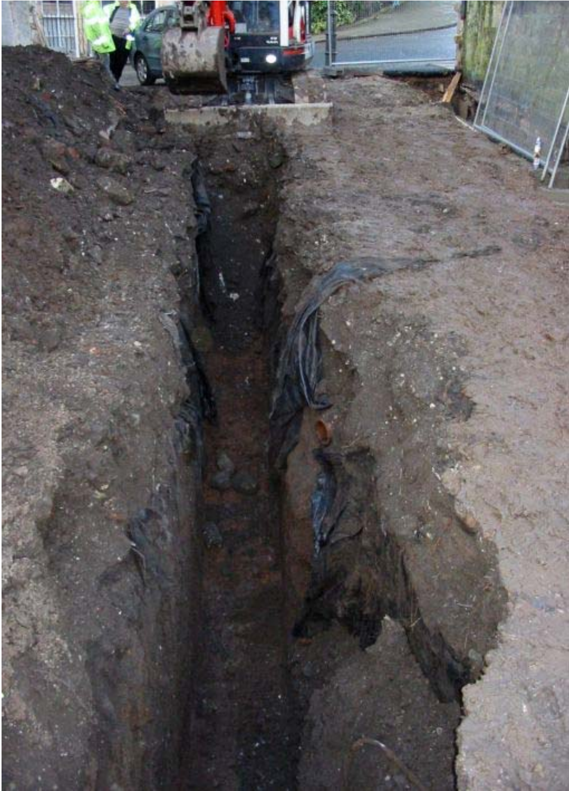
Plate 3: General shot of Foundation Trench 2, facing west
