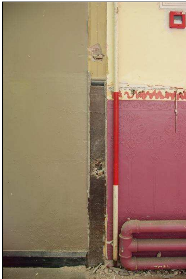
Plate 16: Original decoration revealed in the ground floor main hall
