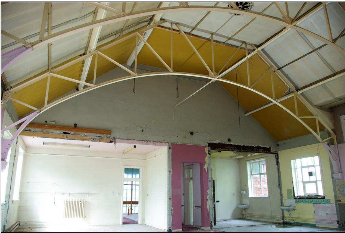
Plate 20: Example of a truss in the main hall on the first floor
