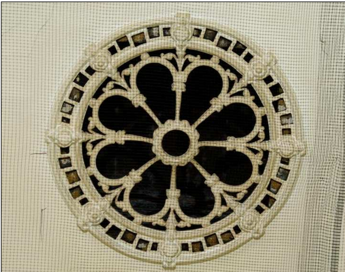
Plate 22: Decorative ceiling vent in the first floor hall
