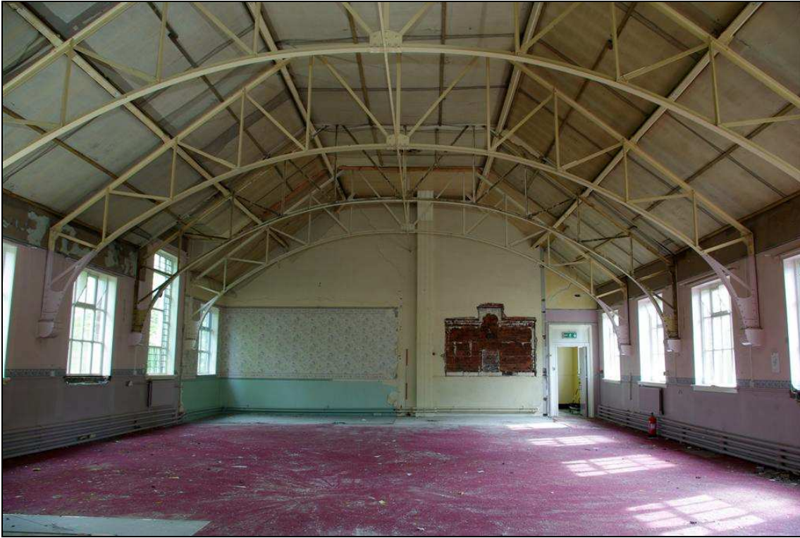
Plate 19: General view of the main hall on the first floor
