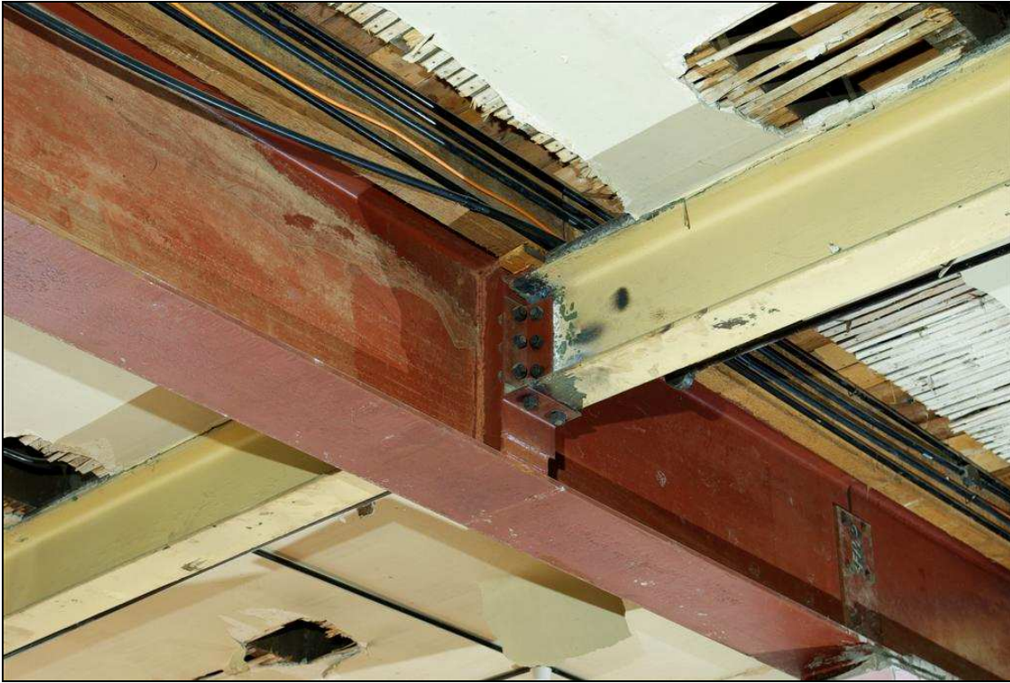
Plate 15: Evidence of beam modification in the ground floor main hall
