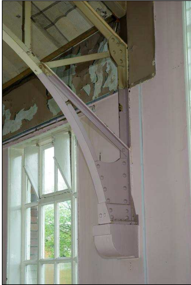
Plate 21: Example of a corbel supporting a truss on the first floor
