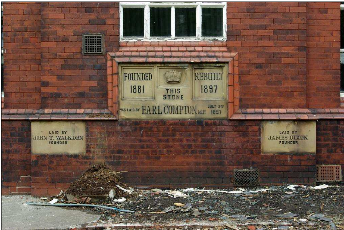
Plate 13: The Foundation stones on the main building
