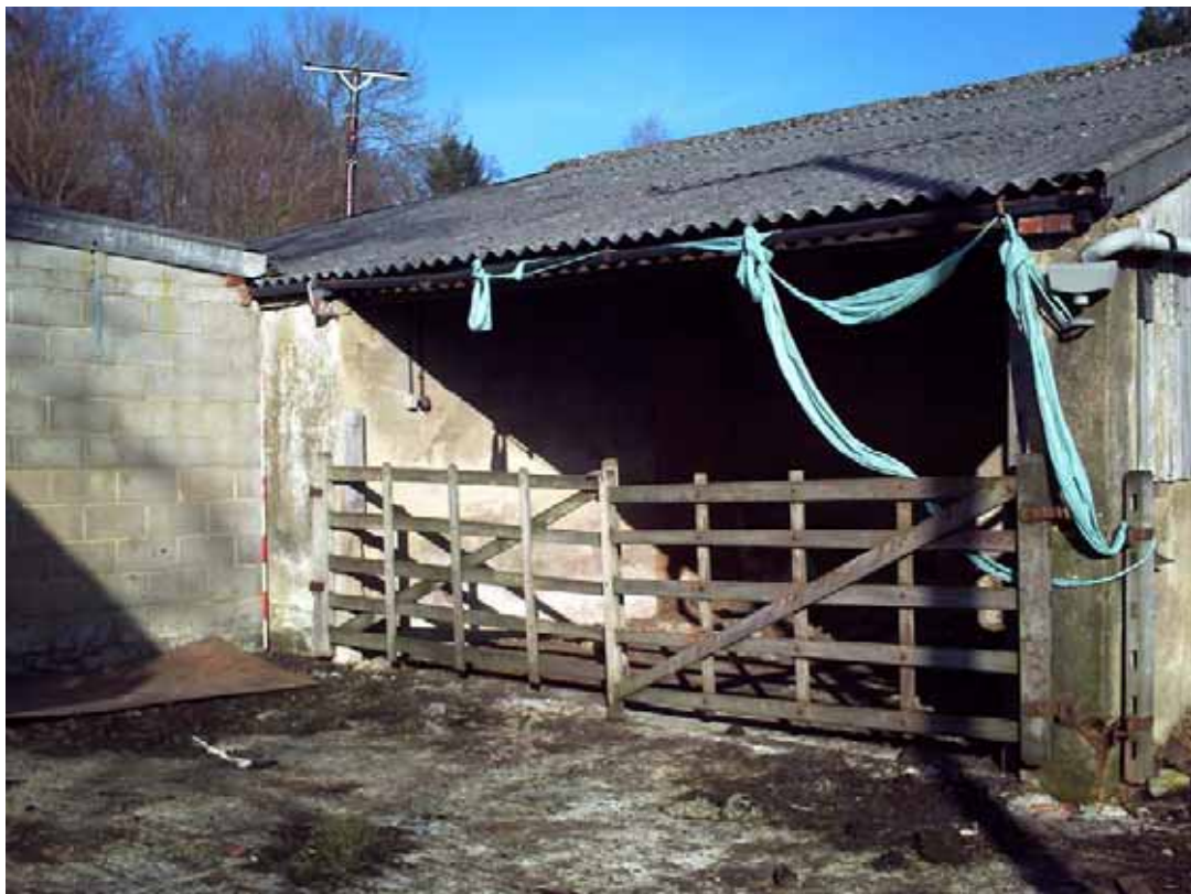
Plate 12: South entrance to Building 3
