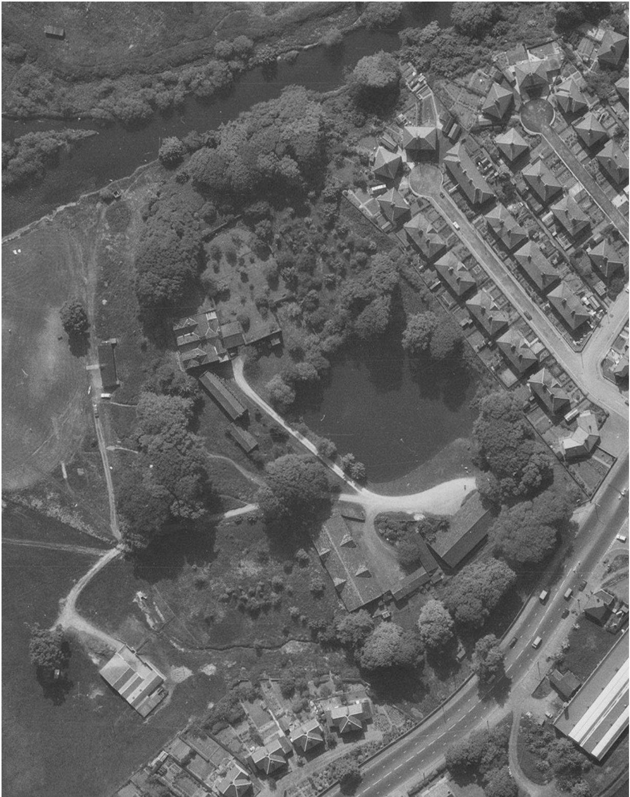
Plate 17: Aerial Photograph of East Riddlesden Hall 1969 (OS/69245-27)
