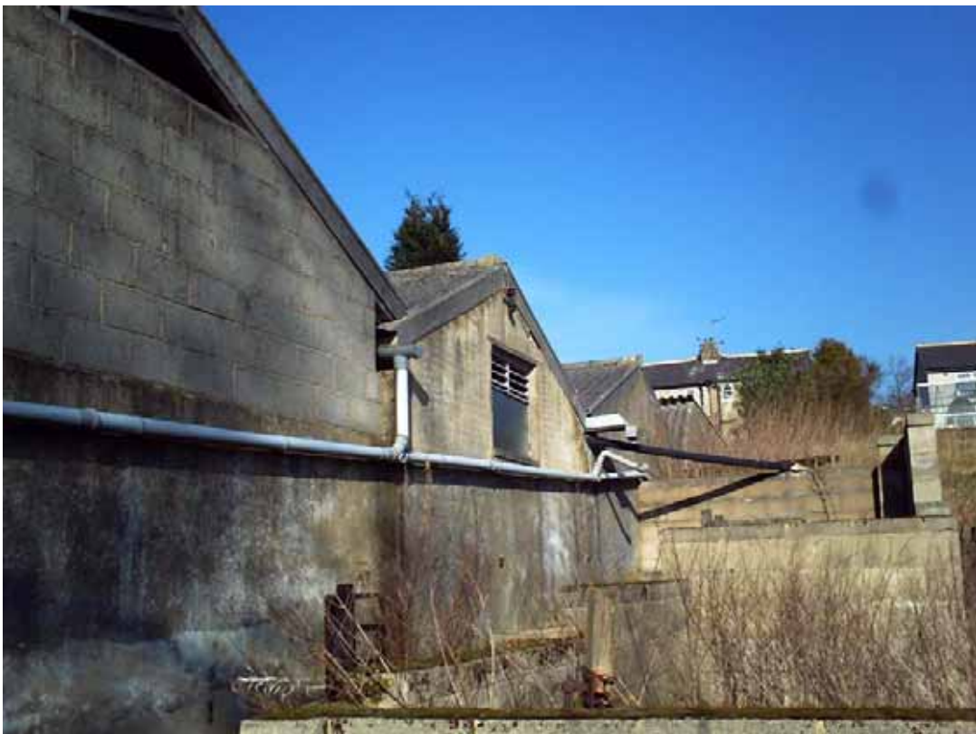
Plate 14: East elevation of Buildings 4 and 5
