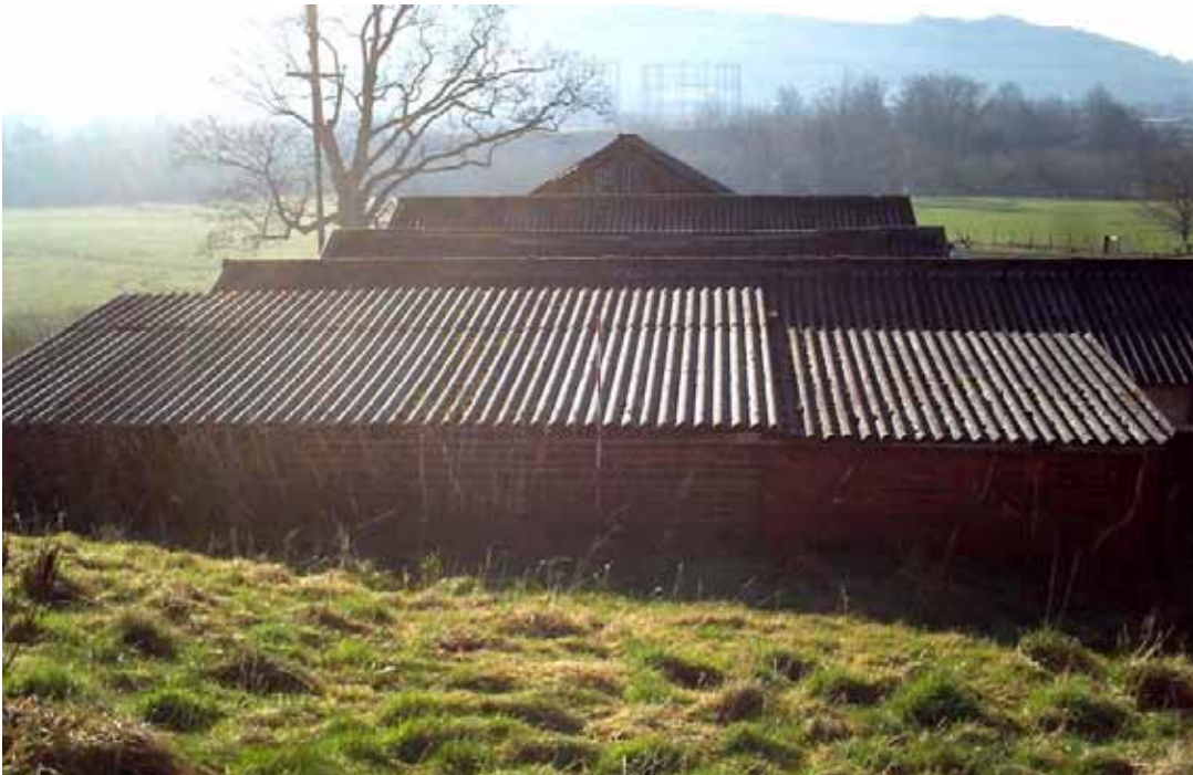
Plate 16: North elevation of Building 6
