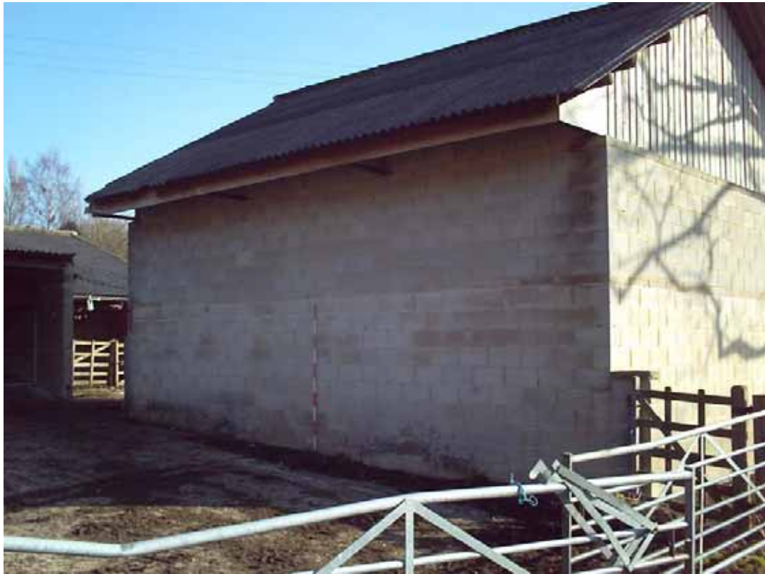
Plate 9: West elevation of the modern barn ( Building 1 )
