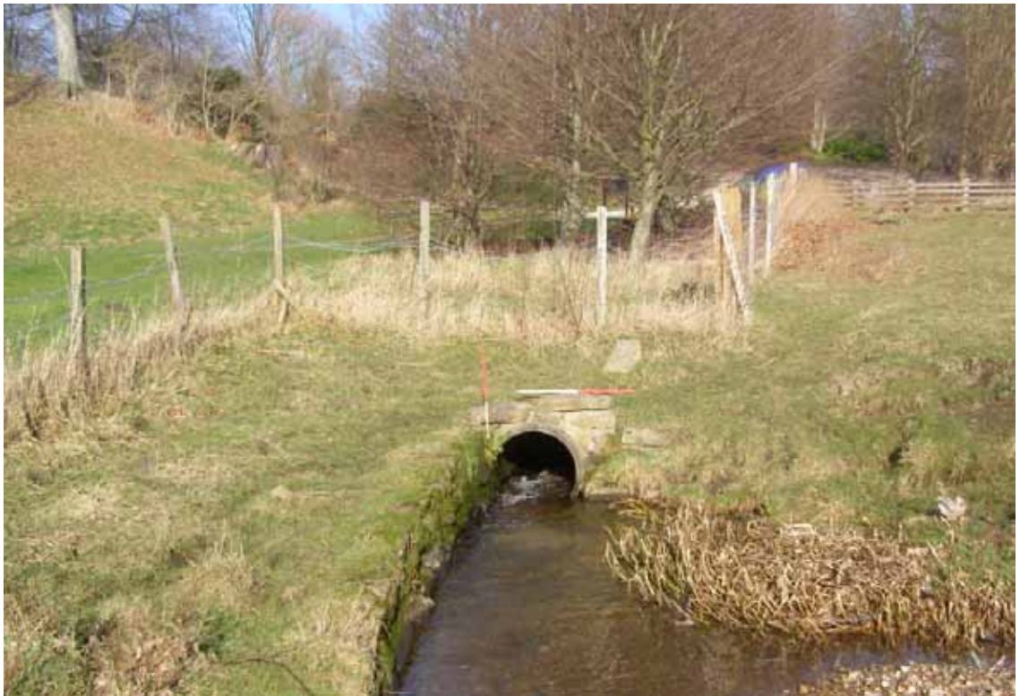
Plate 4: Site 35 - culvert looking north
