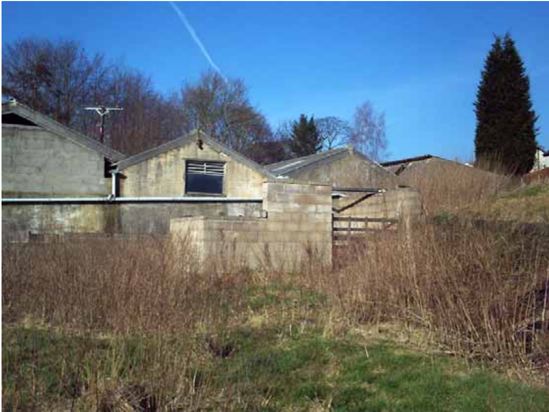
Plate 15: East elevation of Buildings 3-6 (from left to right)
