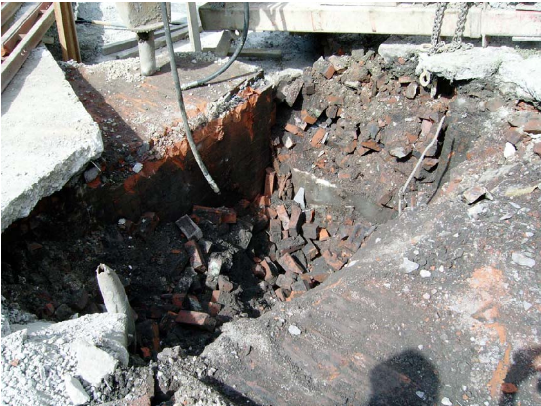
Plate 3: The engine base at the east end of the pipe trench
