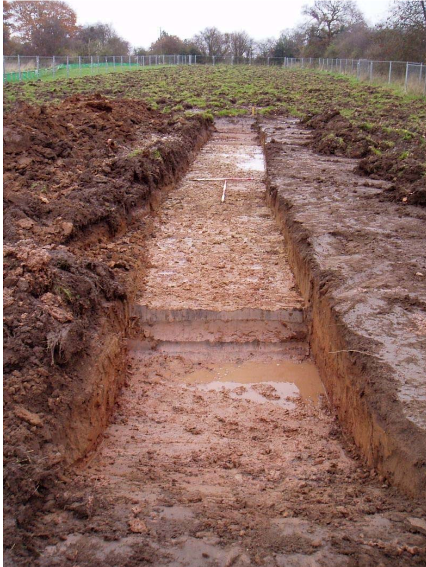
Plate 4: View of Trench 1, looking north
