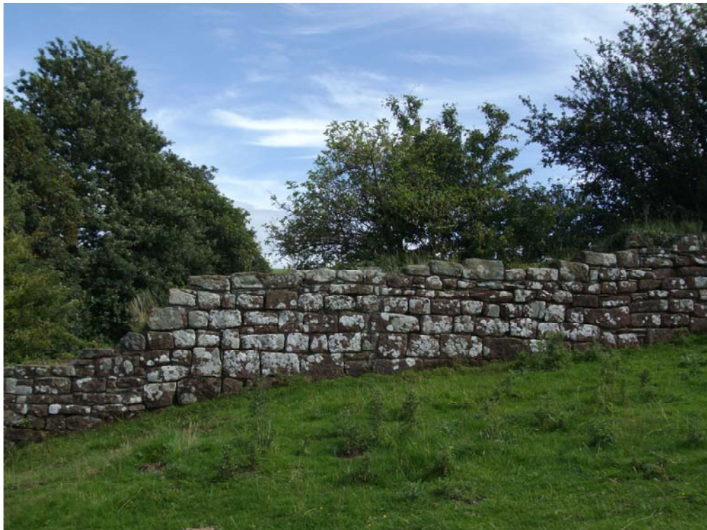
Plate 2: North view of the Abbey Precinct Wall
