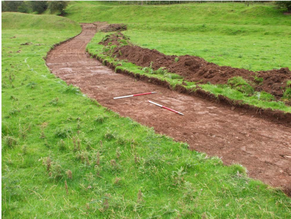
Plate 5: South-eastern view of a stripped section of the greenway, from north of the central section of the area under watching brief
