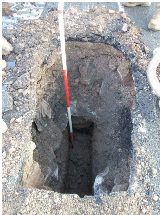
Plate 6: TP302, Old London Road garage site, facing east
