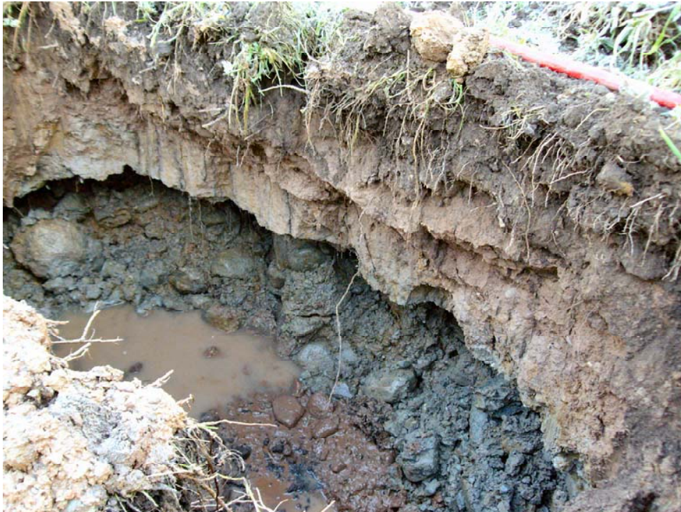
Plate 1: South-west facing section of TP201, Storage pond site, showing unstable ground conditions
