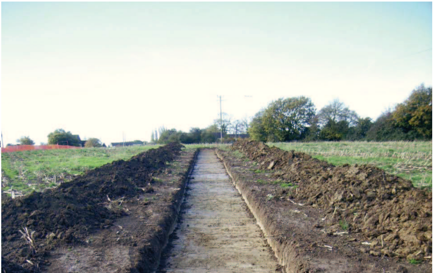
Plate 3: Trench 6, general view showing ridge-and-furrow traces
