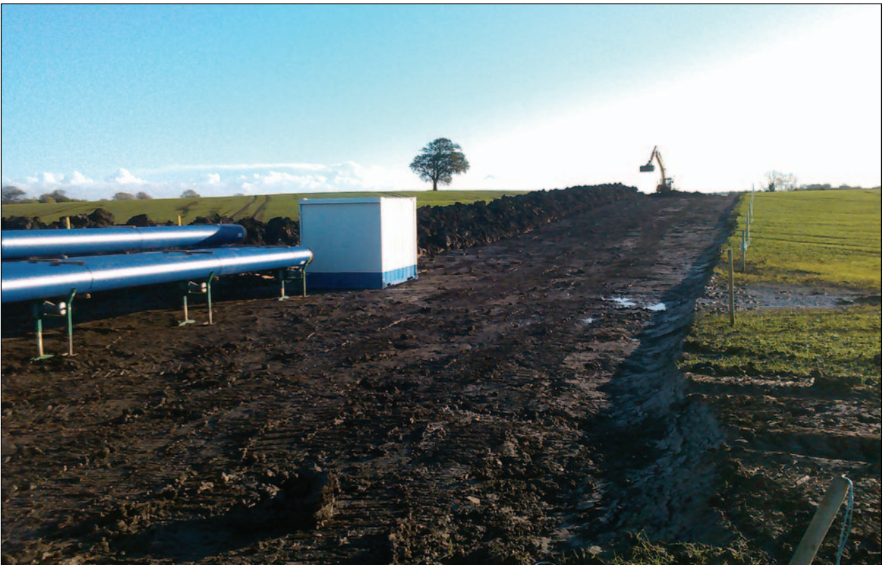
Plate 4: Top Soil excavation
