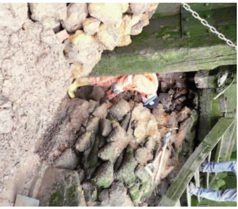
Plate 2: Working in TP01
