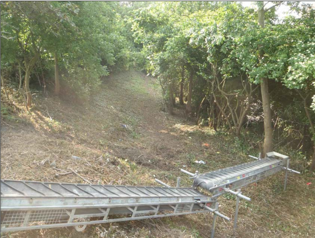
Plate 1: Pre excavation of access ramp to site
