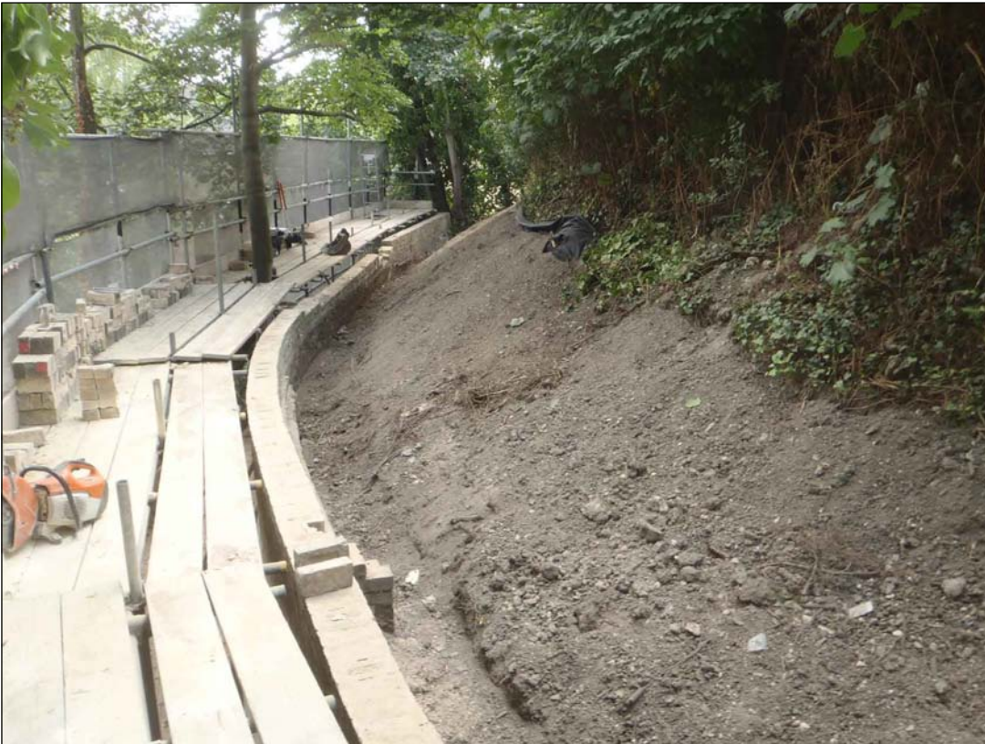
Plate 15: Reinstated section of mound base
