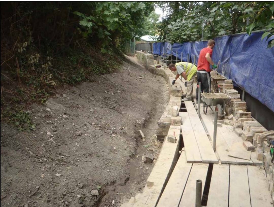
Plate 14: Reinstatement of mound base and wall consolidation.
