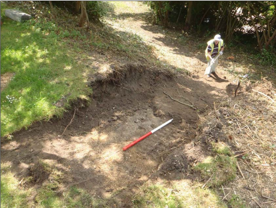
Plate 5: Access ramp to site
