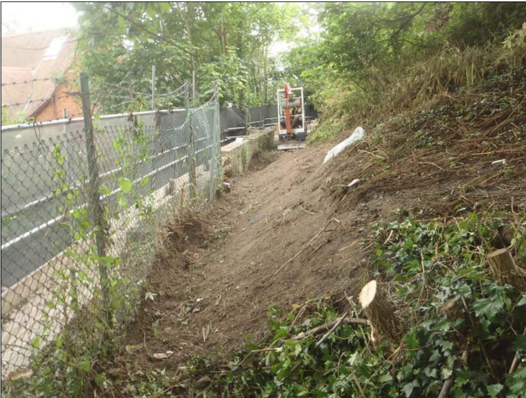
Plate 12: Digging out footing along base of wall during mound reinstatement.
