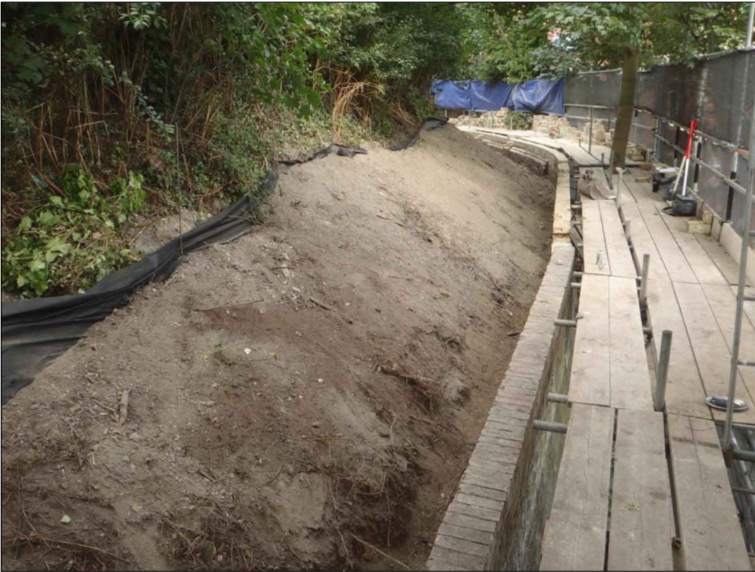
Plate 13: Reinstated section of mound base
