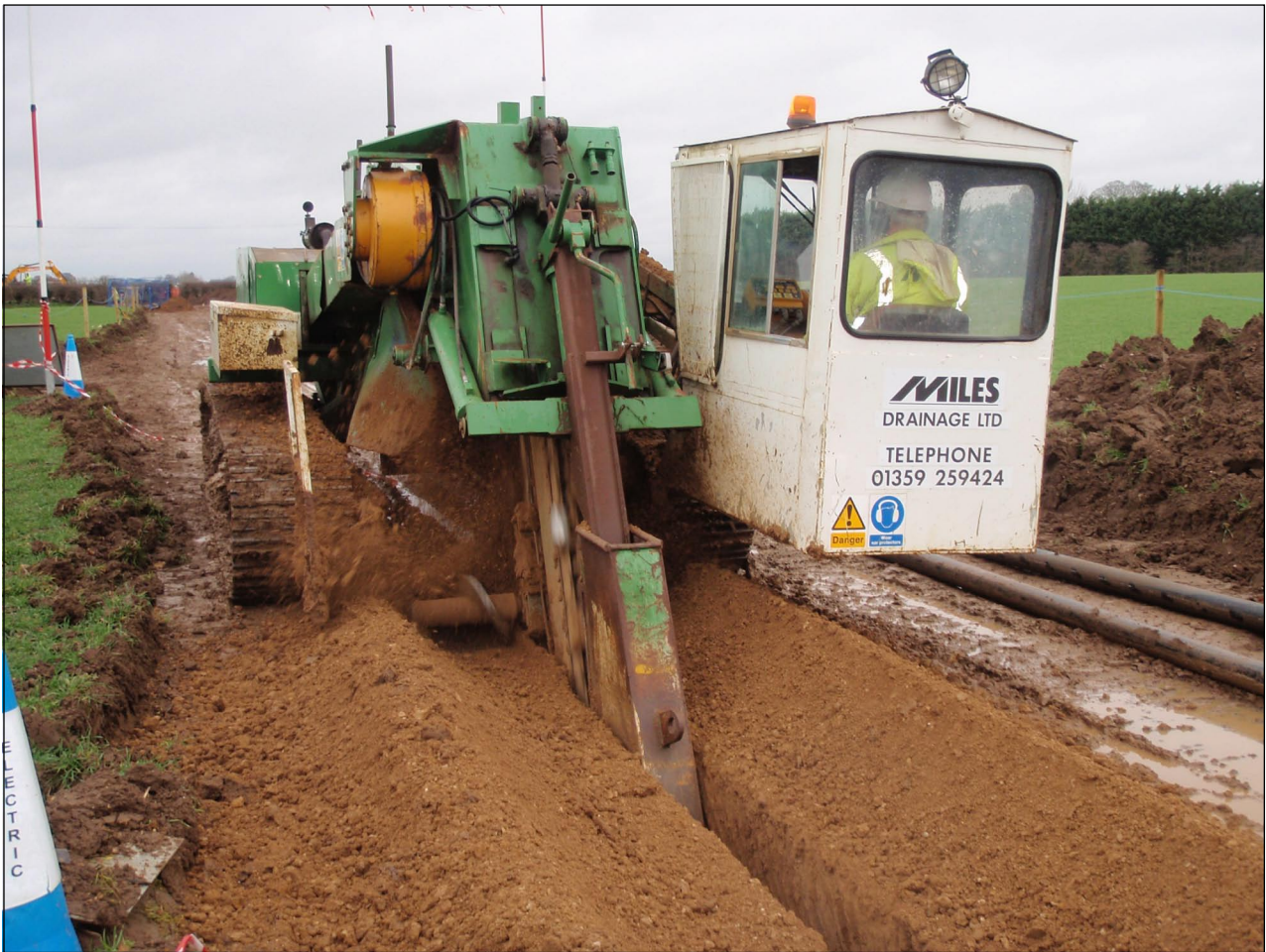
Plate 1: Trenching machine and trench cut, looking south
