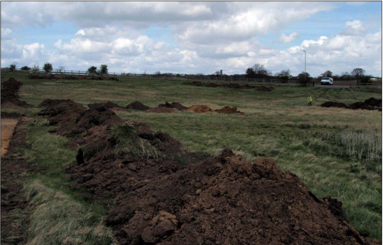
Plate 1: Working shot of site looking north
