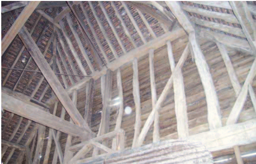
Plate 16: Secondary west end of barn
