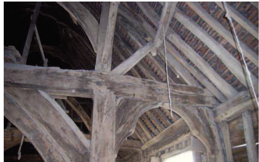
Plate 11: Detail of framing in Frame 3
