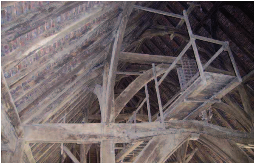
Plate 8: Roof in east half of barn
