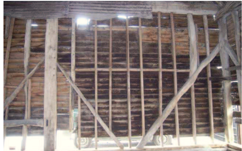
Plate 15: Secondary frame at W end of barn
