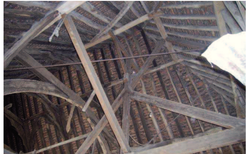
Plate 17: Secondary west end of barn
