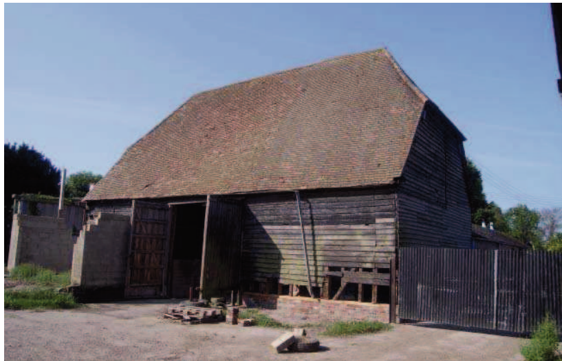
Plate 4: Exterior of barn from NW
