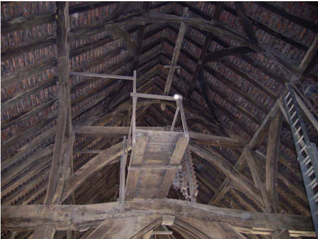
Plate 7: Roof in east half of barn
