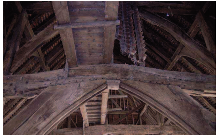
Plate 9: Detail of Frame 2 and 20th-century gantry
