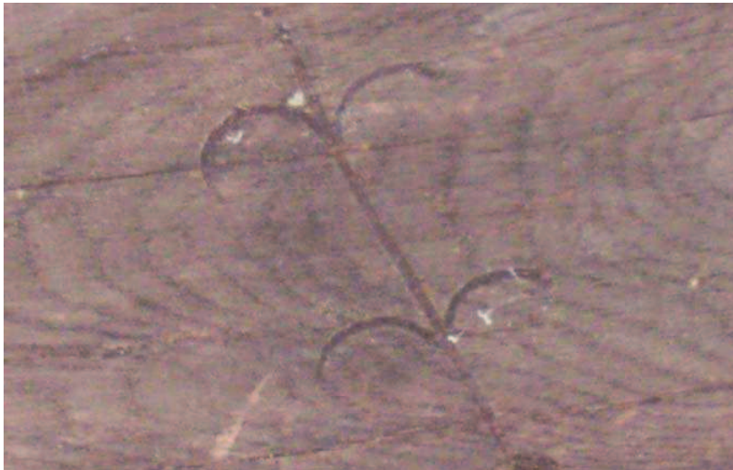
Plate 20: Carpenters mark on Frame 3 (W central)
