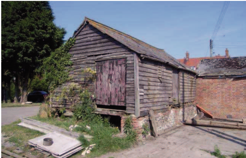
Plate 24: Granary from east
