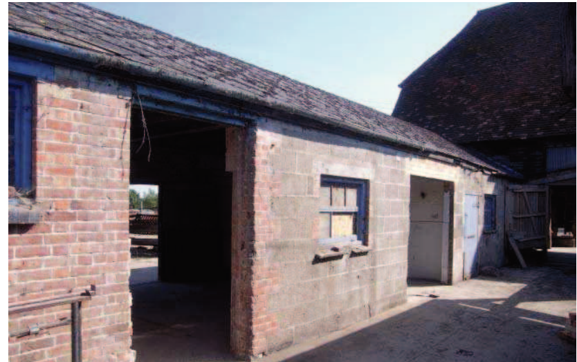
Plate 25: East wall of stables. Right side formerly open fronted
