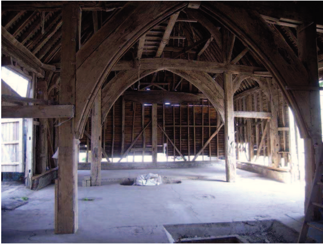
Plate 6: General internal view of barn from east
