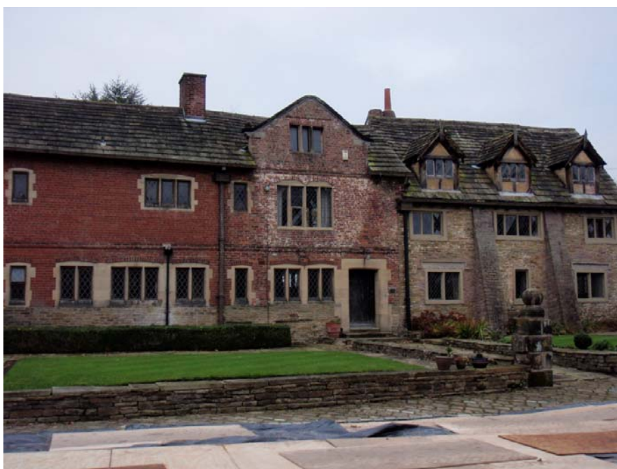
Plate 1: View of the facade of Willot Hall, showing the varying phases of construction
