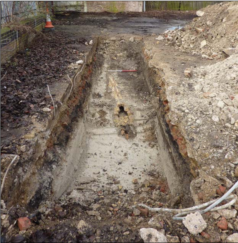
Plate 5: Trench 3, looking west (1m scale)
