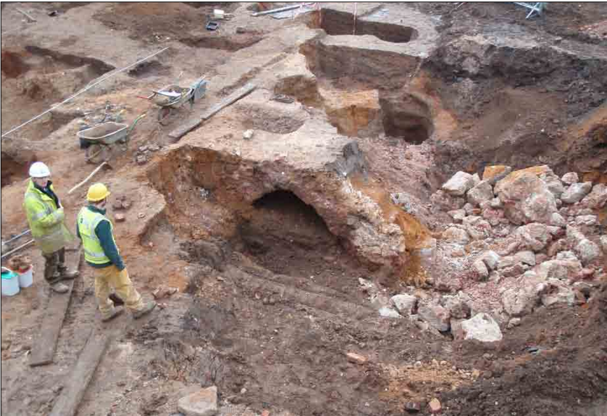
Plate 14: Working shot showing the removal of concrete from within the basement structure.
