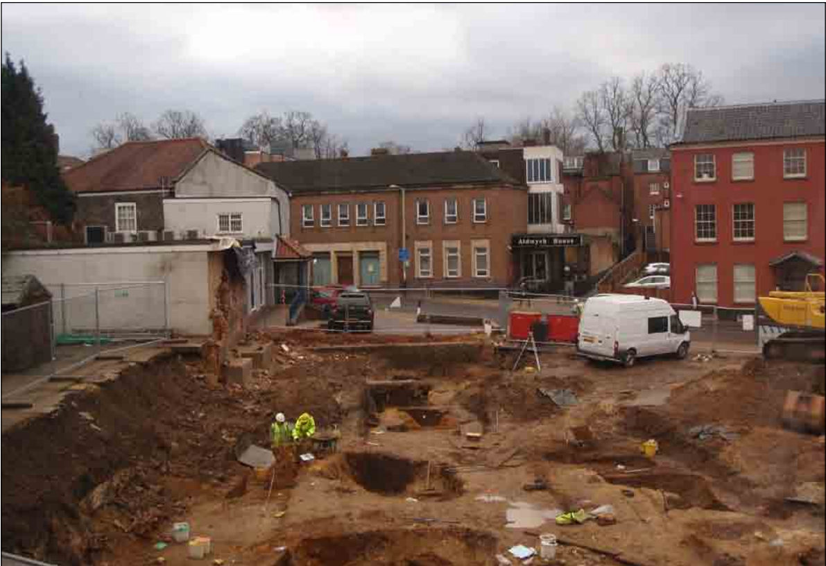
Plate 8: Working shot showing southern half of the excavation area showing pitting, taken from the north.
