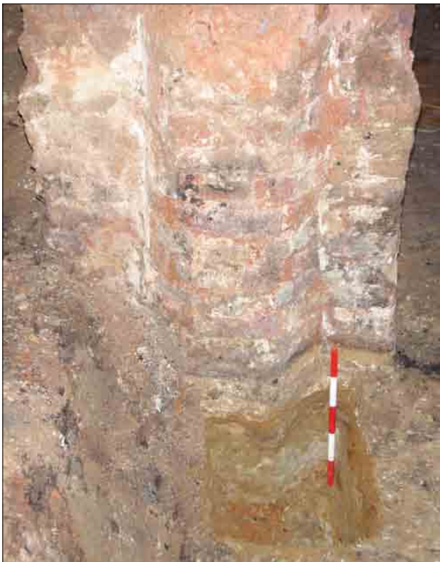
Plate 18: Shot of undercroft pillar footings, taken from the north.
