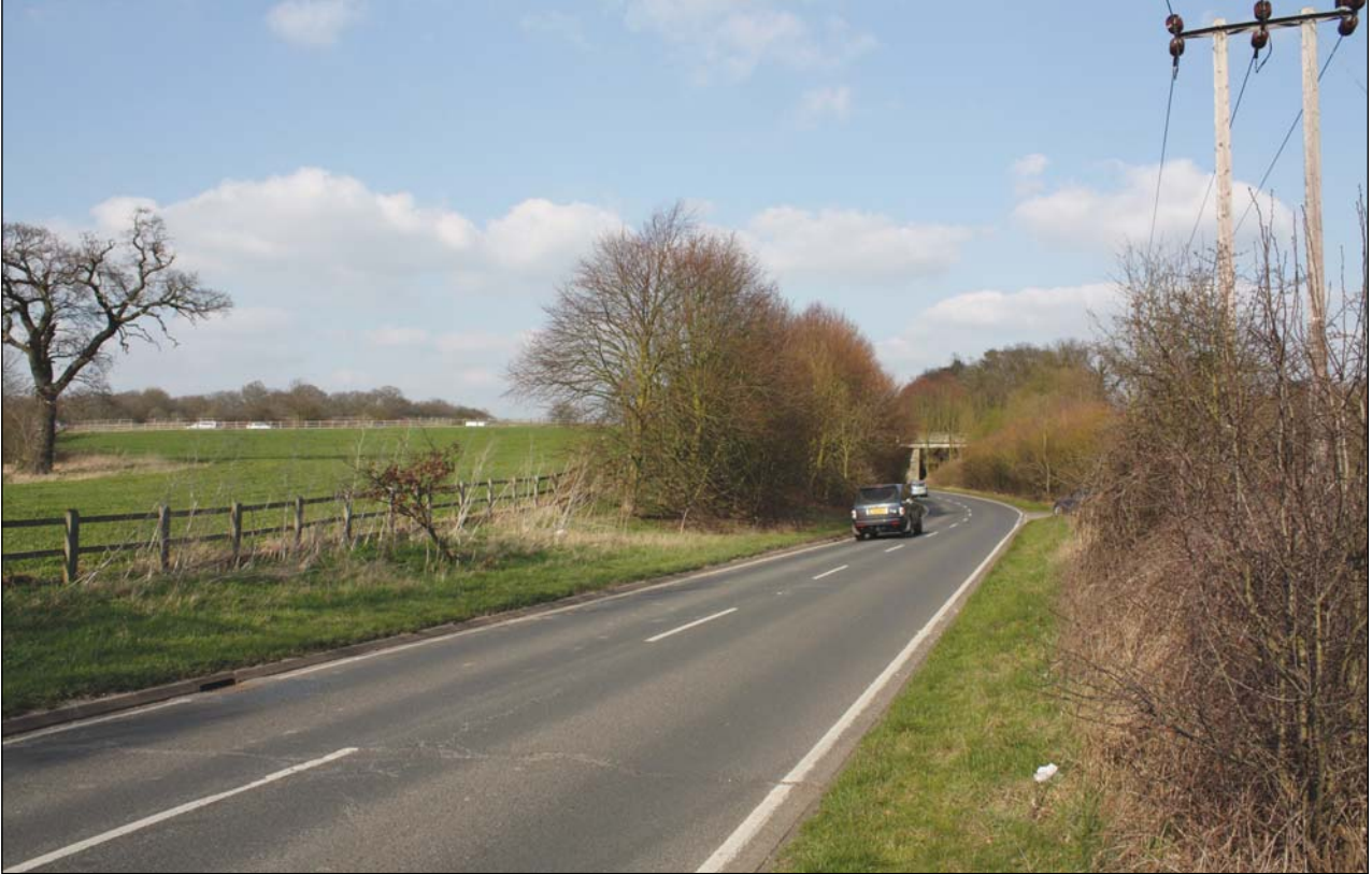
Plate 1: View of A120 flyover with study areas to east and west, taken from Hazelend Rd
