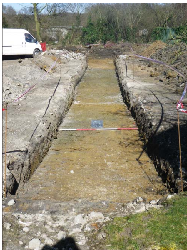
Plate 1: Trench 19 view north east
