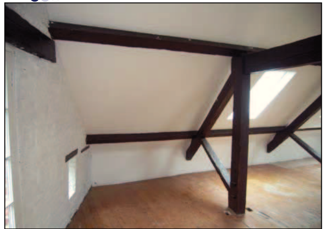
Plate 46: West end of north slope of roof
