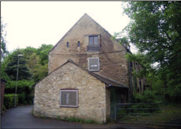
Plate 5: General view from east
