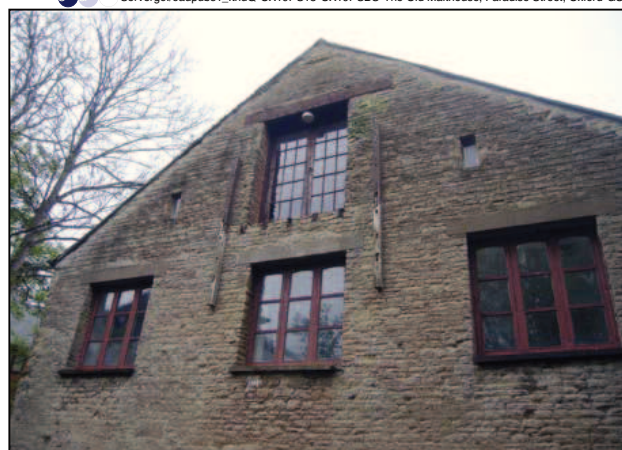
Plate 14: Upper part of west elevation
