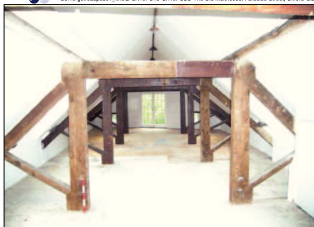
Plate 34: General view of roof structure looking west
