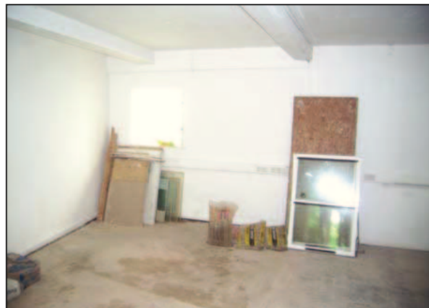
Plate 16: Ground floor, south-east corner
