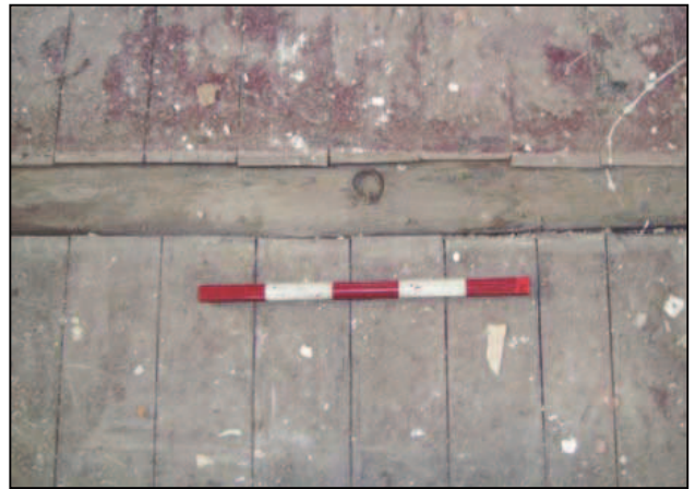
Plate 32: Loop exposed in floor at first floor level
