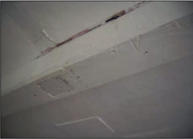
Plate 21: Marks in underside of joist at ground floor level
