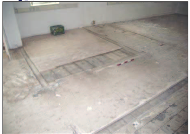
Plate 30: Visible sections of older floor at first floor
