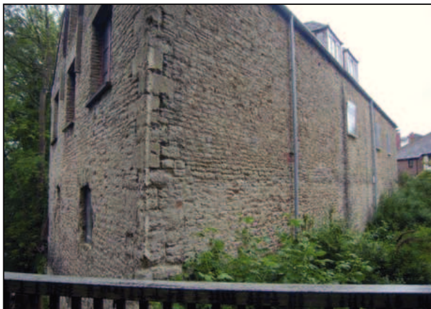
Plate 11: Oblique south-west corner of building
