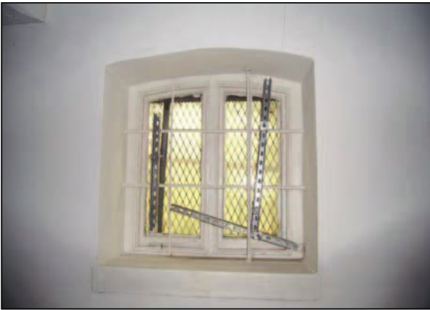
Plate 19: Ground floor window
