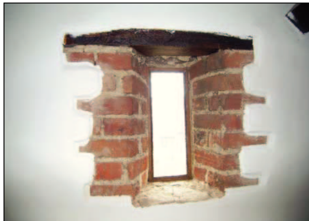
Plate 52: Detail of window at east end
