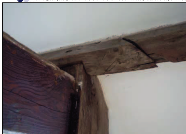
Plate 50: Purlin scarf detail
