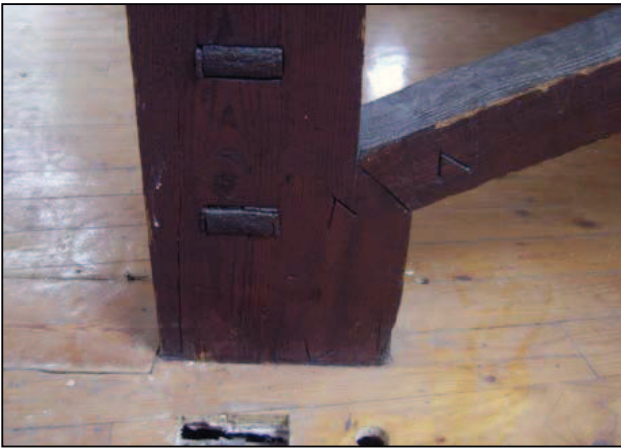
Plate 43: Roman numeral carpenter's marks at base of queen post
