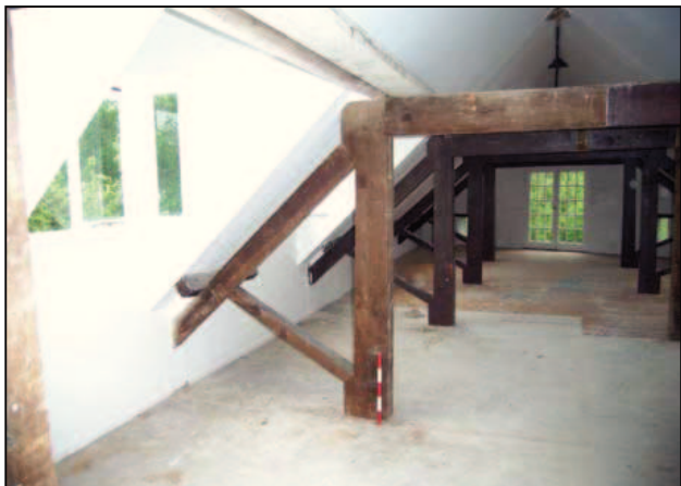
Plate 35: General view of roof towards west
