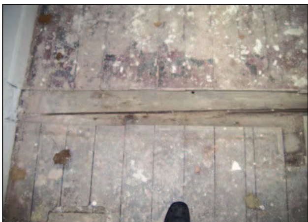
Plate 33: Exposed beam at first floor
