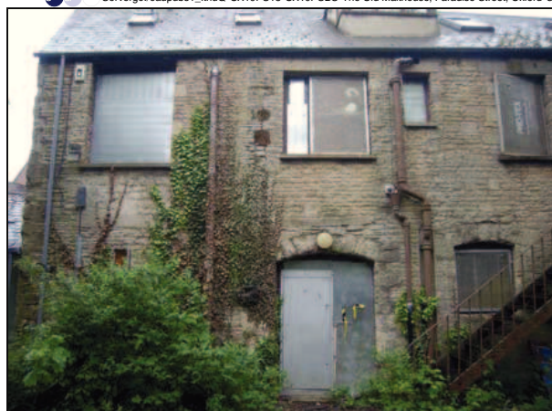
Plate 2: East half of north elevation
