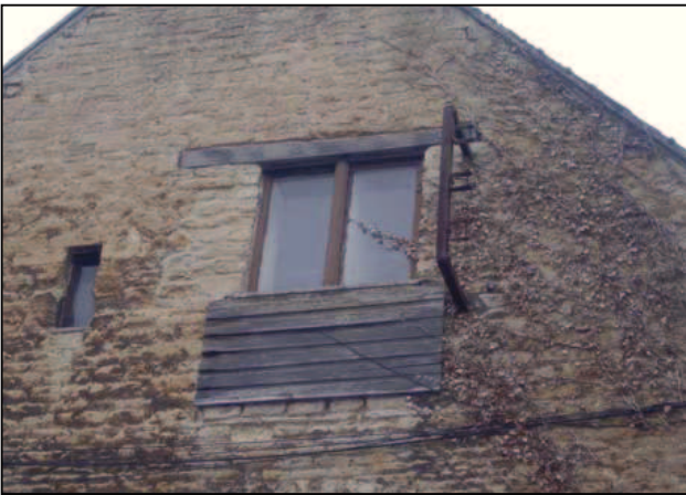
Plate 7: Loading door in east elevation converted to window
