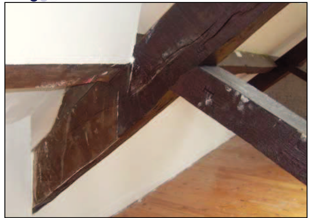
Plate 42: Roof detail – raking strut to purlin
