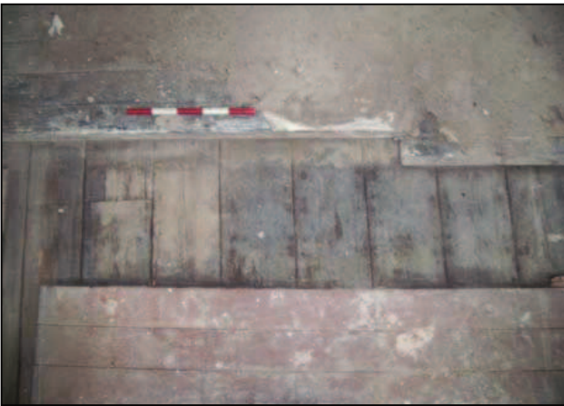
Plate 31: Older floorboards visible at first floor
