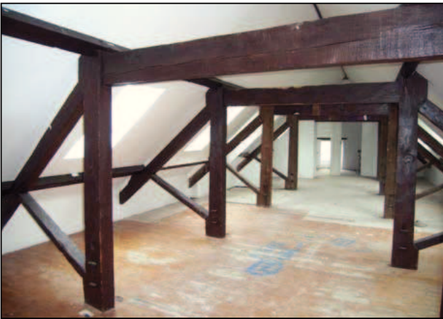
Plate 47: General view of roof from west
