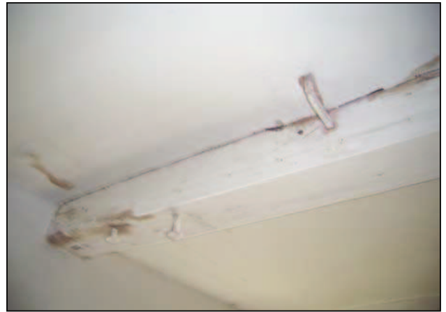
Plate 20: Third principal joist from east at ground floor
