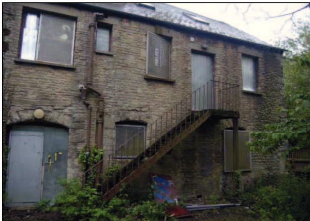
Plate 3: West half of north elevation
