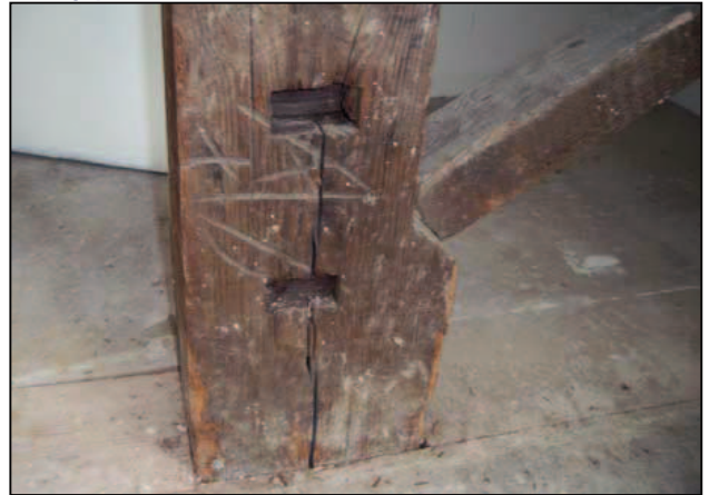
Plate 38: Importers marks on the post at the eastern end
