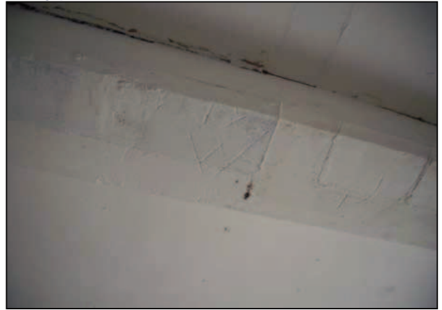
Plate 22: Importers marks in underside of joist at ground floor
