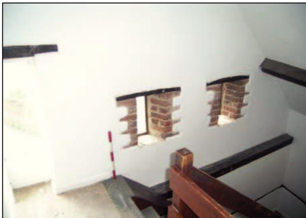
Plate 51: East end at second floor level
