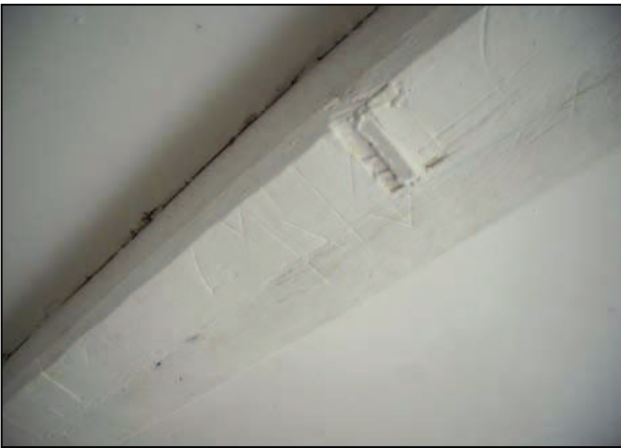
Plate 23: Importers marks in underside of joist at ground floor
