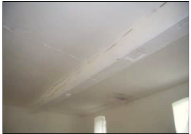
Plate 24: Westernmost joist at ground floor with imprint from former posts
