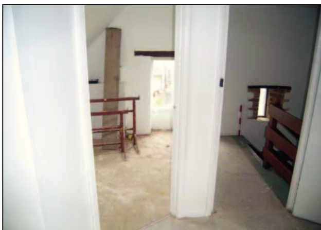
Plate 49: General view of east end of building
