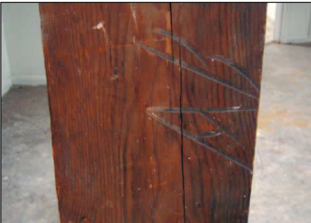
Plate 39: Importers marks on the post in the second truss from the east
