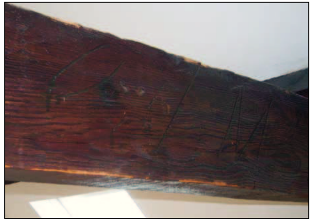
Plate 48: Importers marks on side of collar
