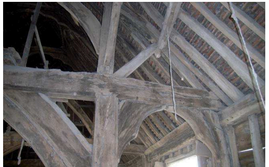
Plate 11: Detail of framing in Frame 3
