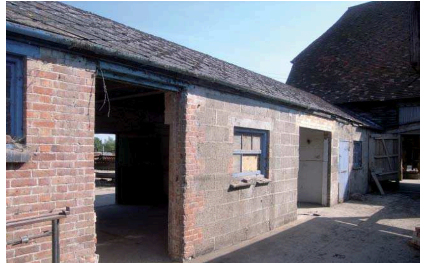
Plate 25: East wall of stables. Right side formerly open fronted
