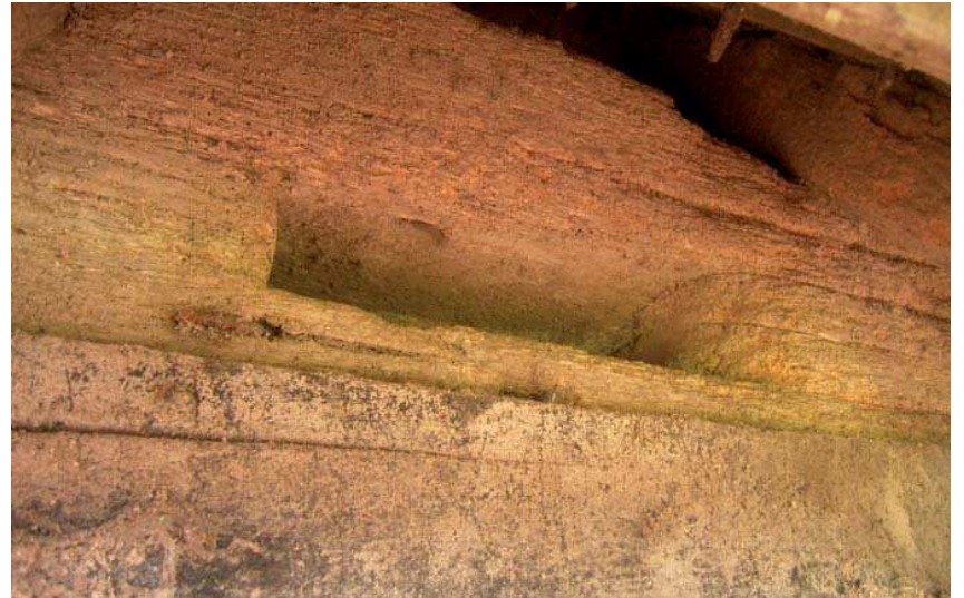
Plate 21: Chase mortise in face of wall plate, under eaves, from former projecting oriel
