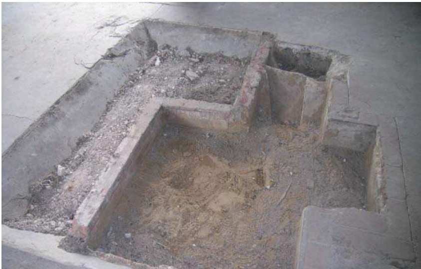
Plate 18: Modern trough/chute in floor of barn
