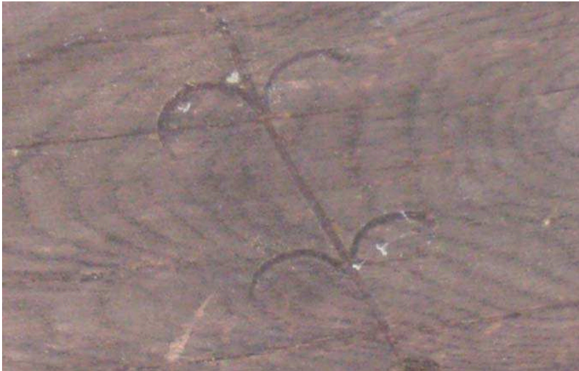
Plate 20: Carpenters mark on Frame 3 (W central)
