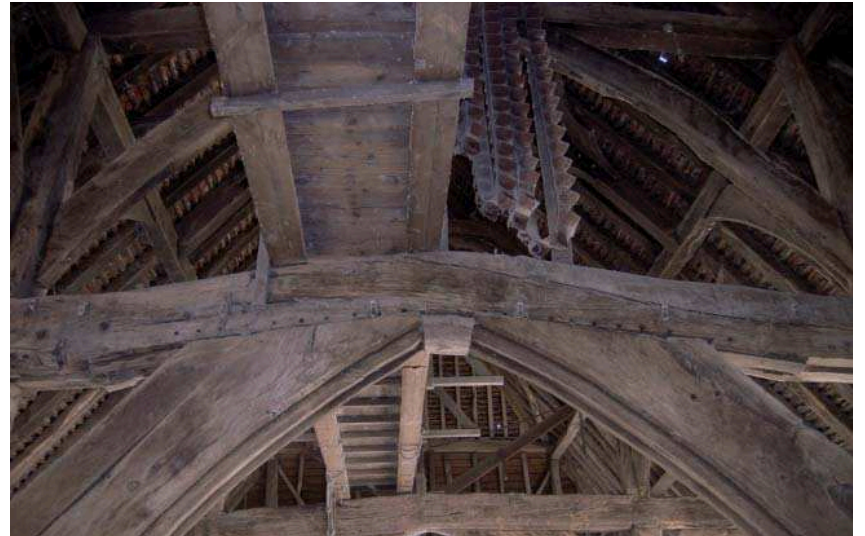
Plate 9: Detail of Frame 2 and 20th-century gantry
