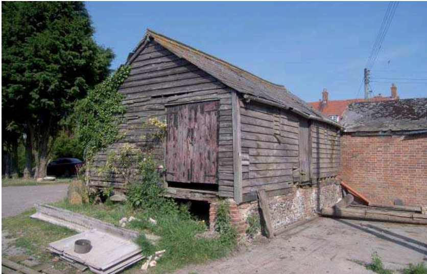
Plate 24: Granary from east
