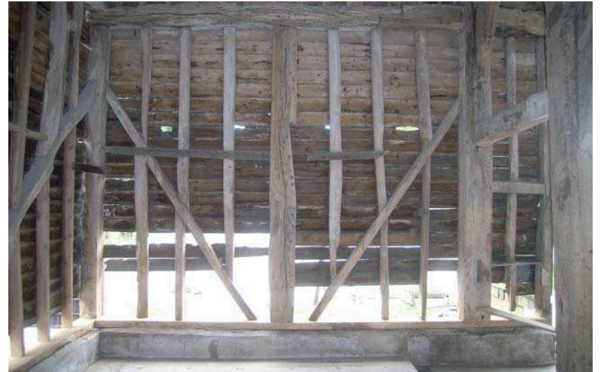
Plate 13: Secondary framing and possibly reused tie at W end of N wall
