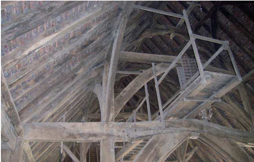
Plate 8: Roof in east half of barn
