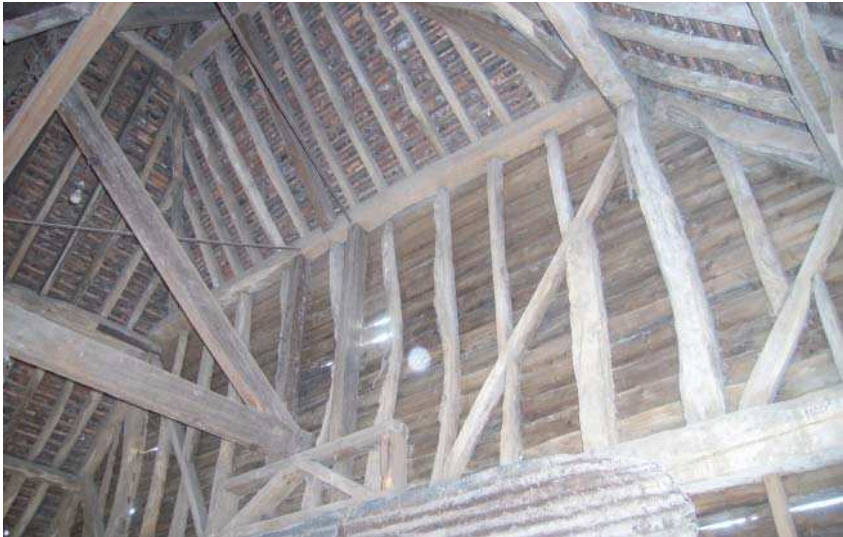
Plate 16: Secondary west end of barn
