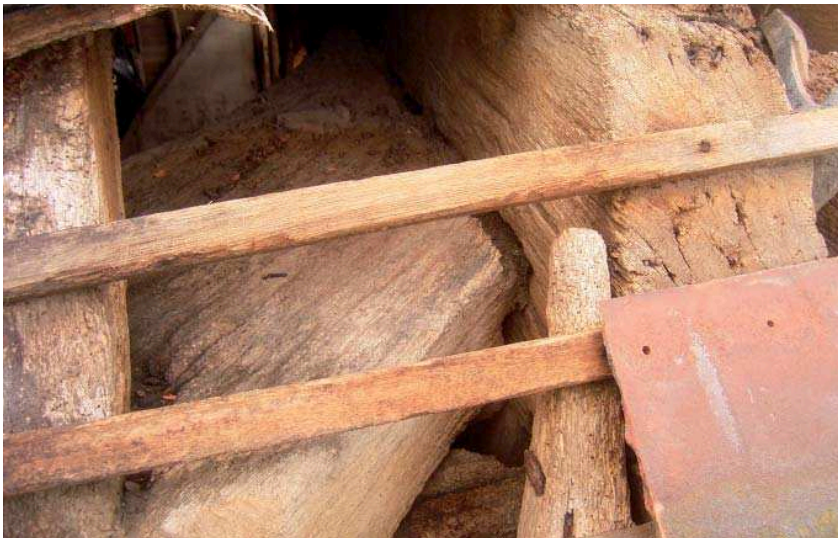
Plate 22: Curved corner brace and end of tie beam at E end of barn
