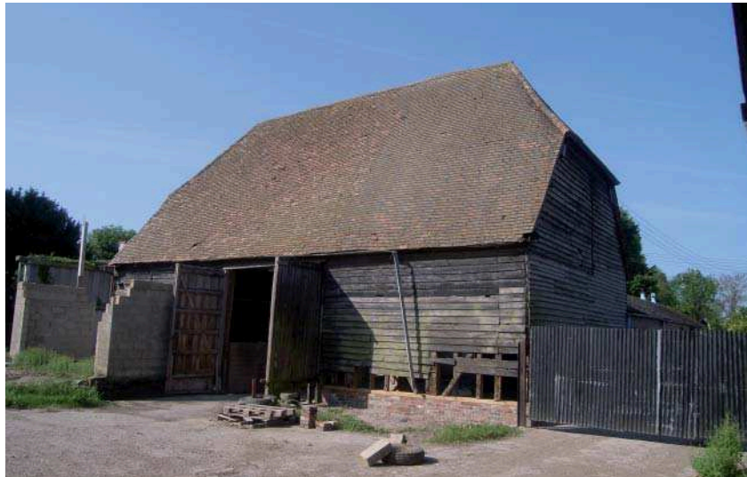
Plate 4: Exterior of barn from NW
