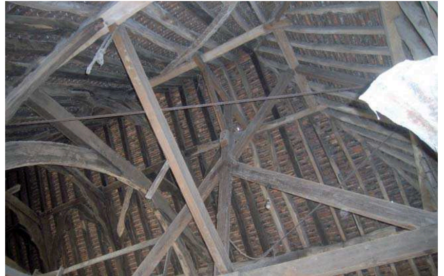
Plate 17: Secondary west end of barn
