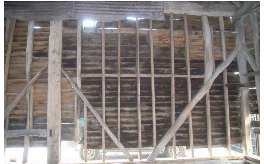
Plate 15: Secondary frame at W end of barn
