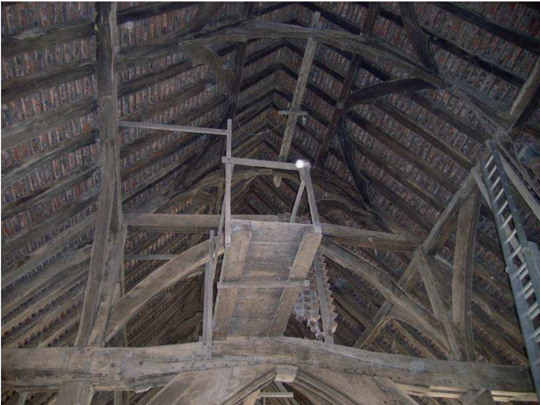
Plate 7: Roof in east half of barn
