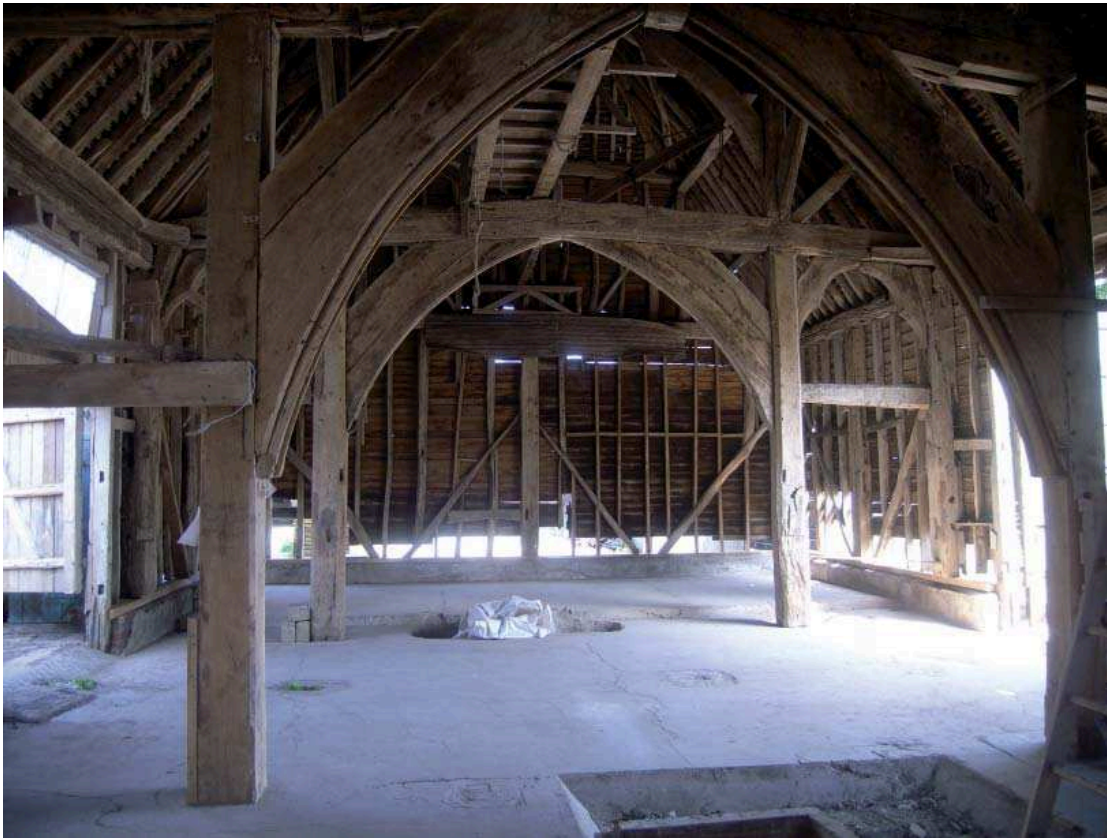
Plate 6: General internal view of barn from east
