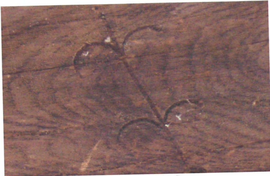
Plate 20: Carpenters mark on Frame 3 (W central)
