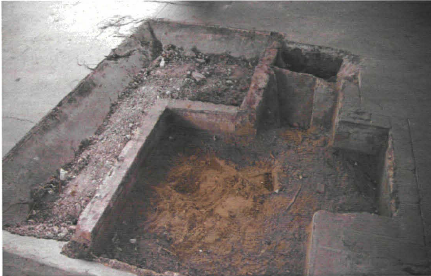
Plate 18: Modern trough/chute in floor of barn
