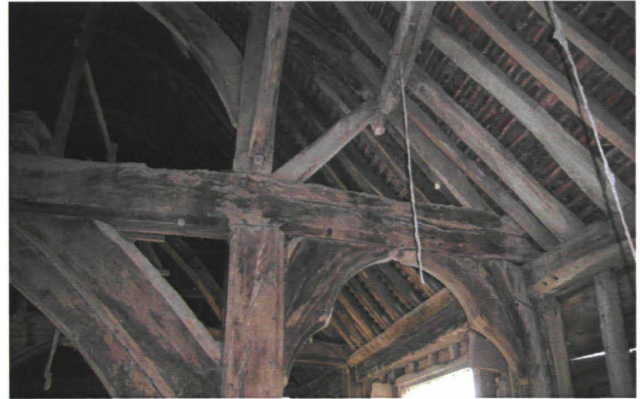
Plate 11: Detail of framing in Frame 3
