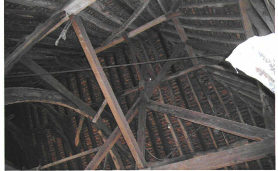
Plate 17: Secondary west end of barn
