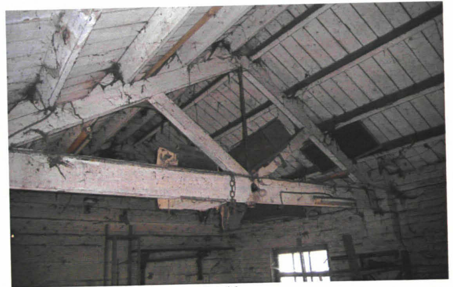
Plate 27: Interior of north room of stable range
