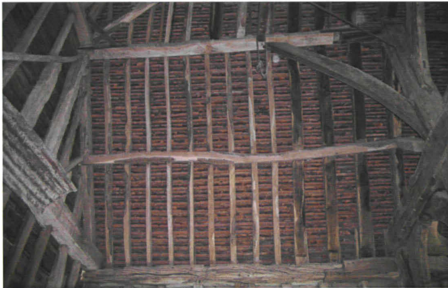
Plate 14: Roof at W end. Rafters to left secondary. Primary smoke blackened rafters to right
