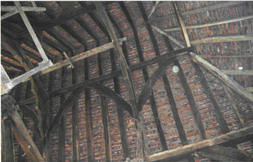
Plate 10: View of roof at east end of barn
