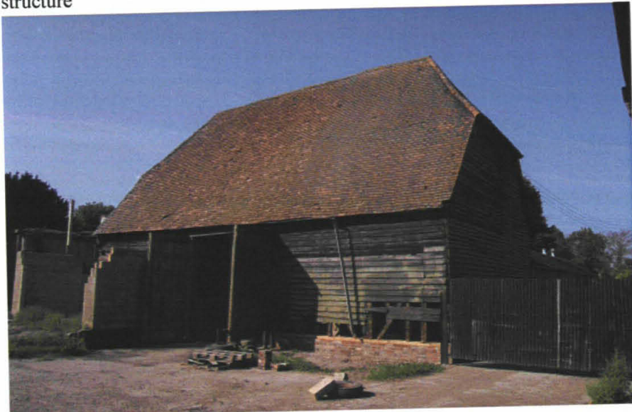
Plate 4: Exterior of barn from NW
