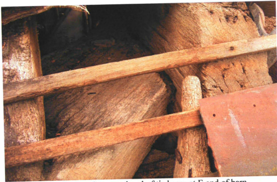
Plate 22: Curved corner brace and end of tie beam at E end of barn
