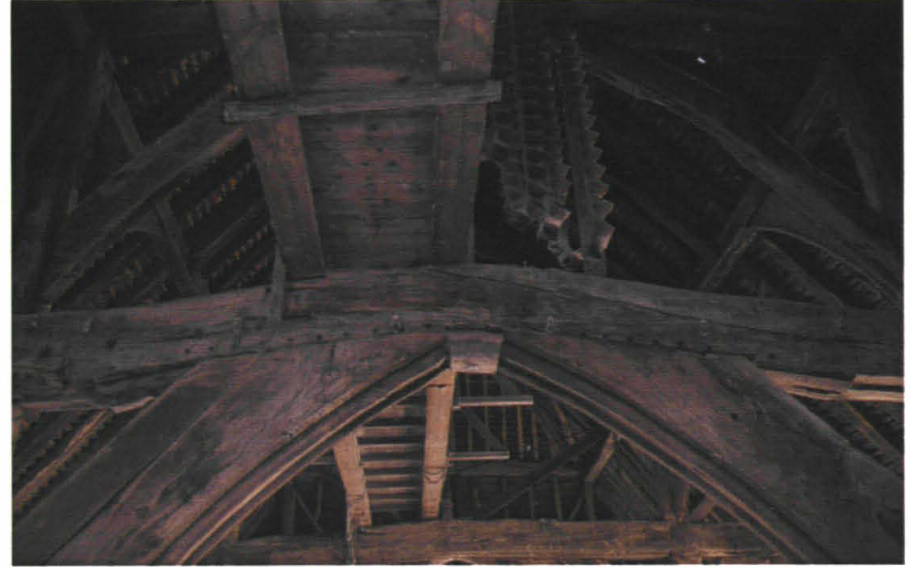
Plate 9: Detail of Frame 2 and 20th-century gantry
