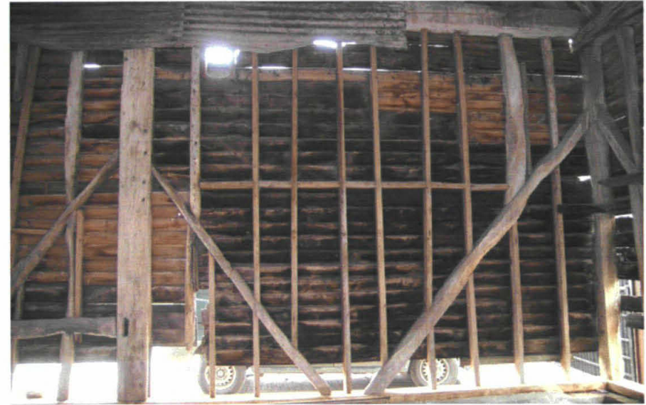
Plate 15: Secondary frame at W end of barn
