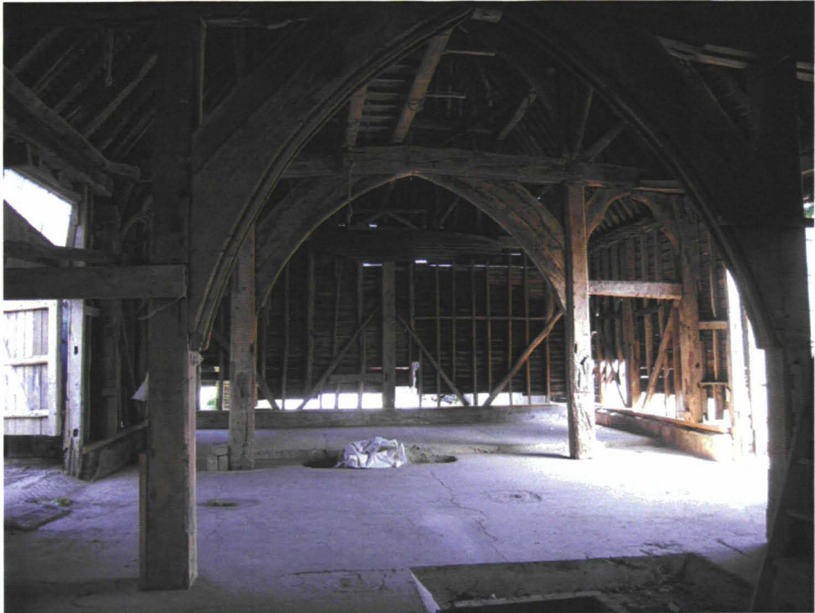
Plate 6: General internal view of barn from east
