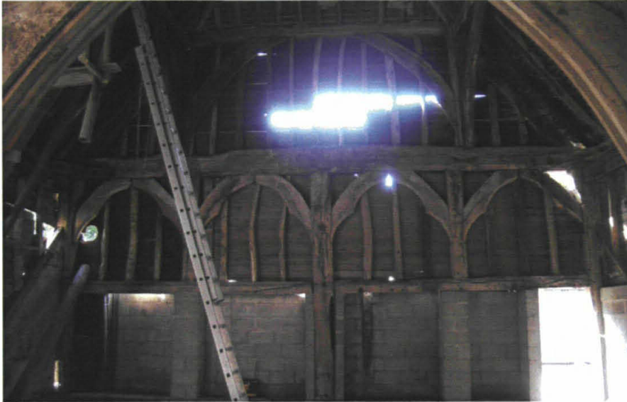
Plate 12: East end of barn (Frame 1)
