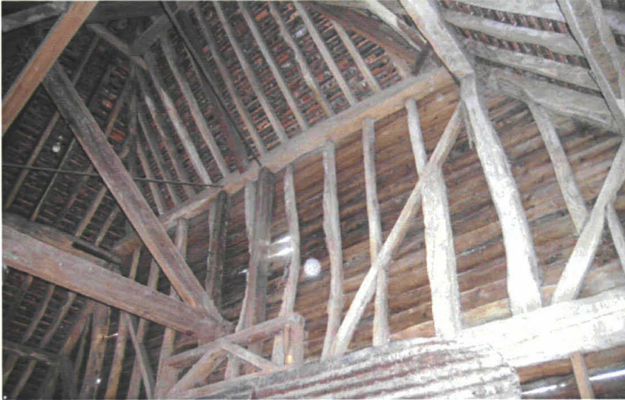
Plate 16: Secondary west end of barn
