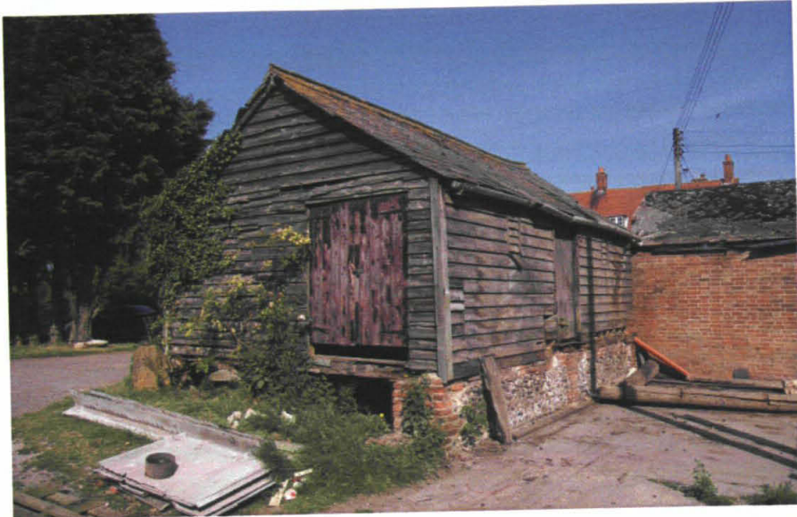
Plate 24: Granary from east
