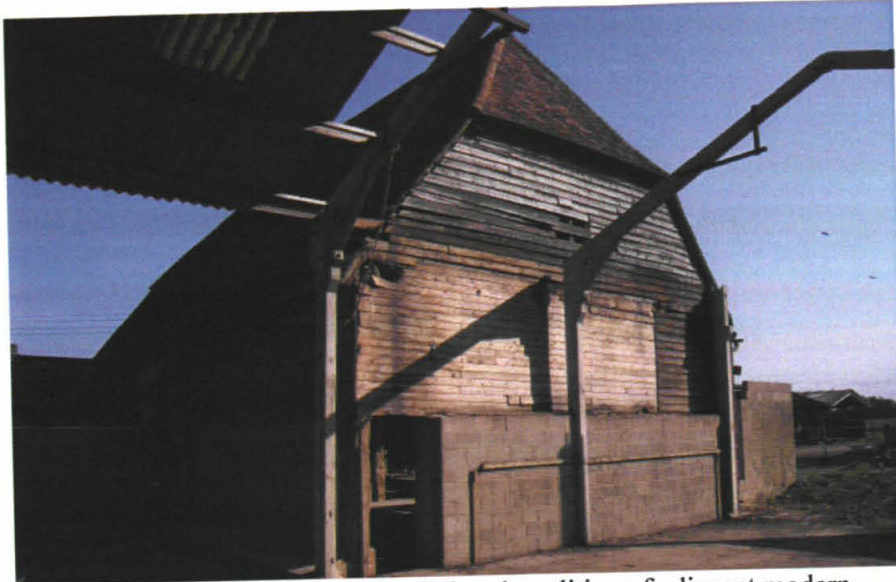
Plate 3: Exterior of barn from SE during demolition of adjacent modern structure
