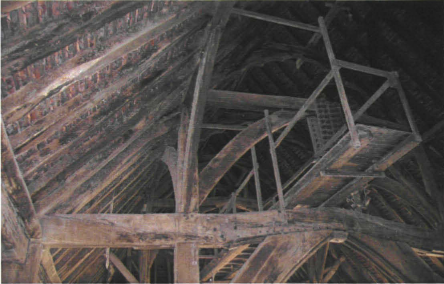
Plate 8: Roof in east half of barn
