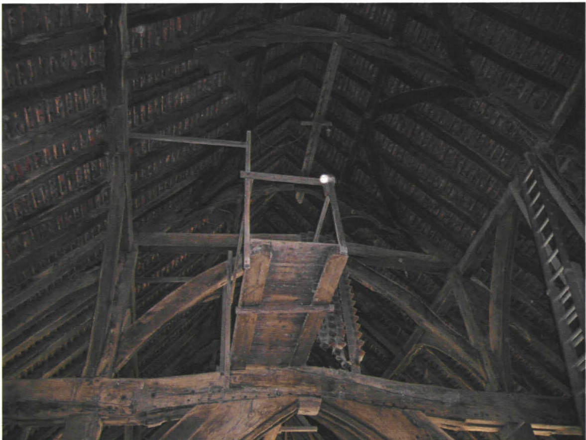
Plate 7: Roof in east half of barn
