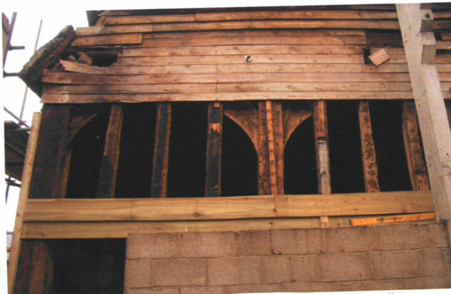
Plate 5: Detail of east elevation during removal of weather boarding
