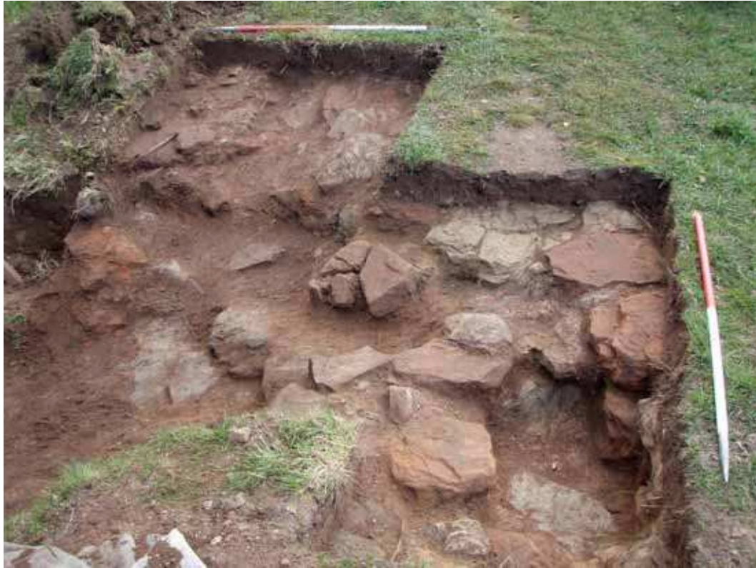
Plate 1: The foundation of the stone phase of Hadrian's Wall ( 101 ) in Trench 1, looking south-east (1m scales)
