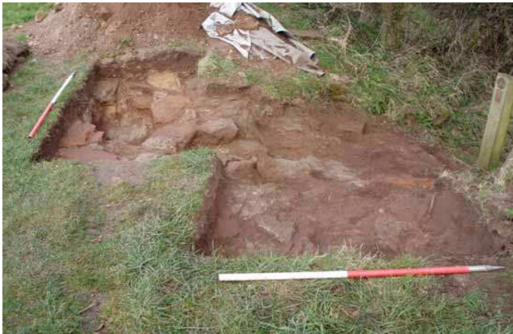
Plate 2: The foundation of the stone phase of Hadrian's Wall ( 101 ), on the edge of the scarp slope, looking north-west (1m scale)
