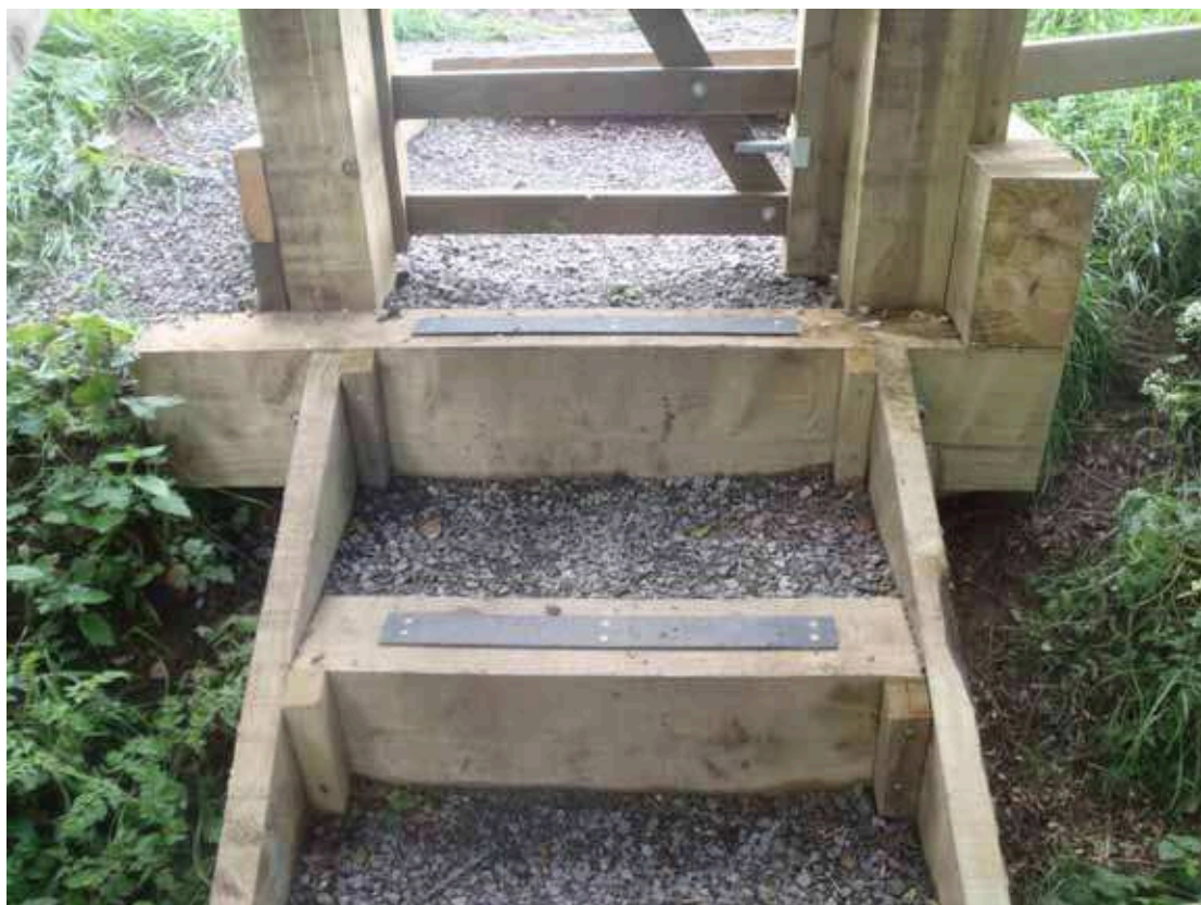
Plate 7: The gate as installed, over the foundations of Hadrian's Wall
