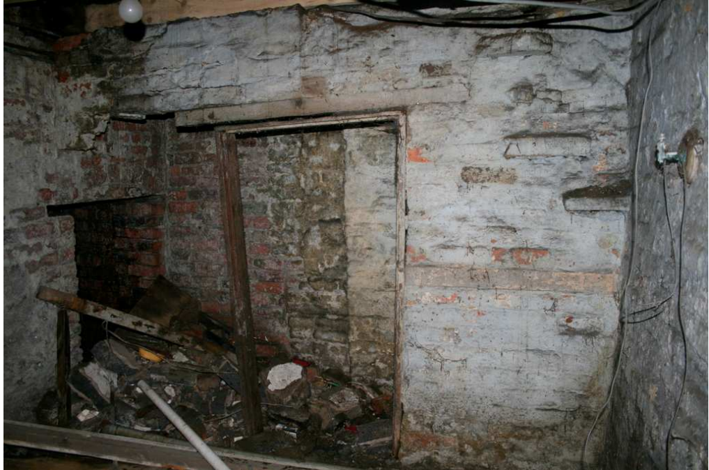
Plate 32: Stair wall and possible coal store, cellar, 7 Greengate
