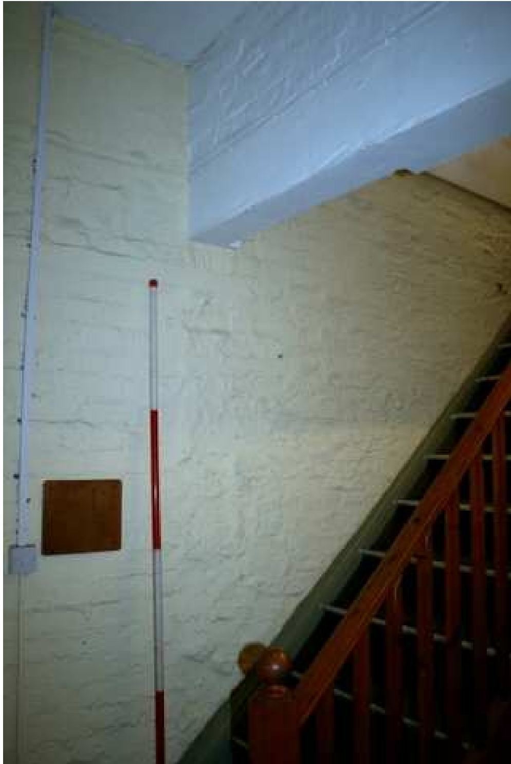
Plate 7: Original external wall carried over late staircase, with associated wall scar
