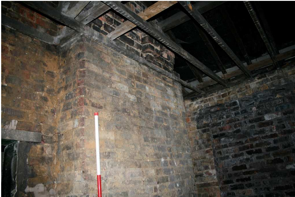
Plate 29: Blocked window in west wall, and corbelling to purlin, second floor, 7 Greengate
