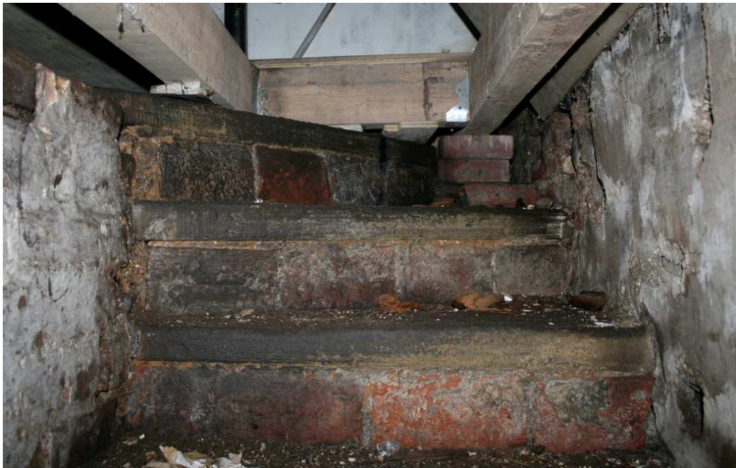
Plate 31: Edge-set brick risers, and flagstone steps, cellar, 7 Greengate
