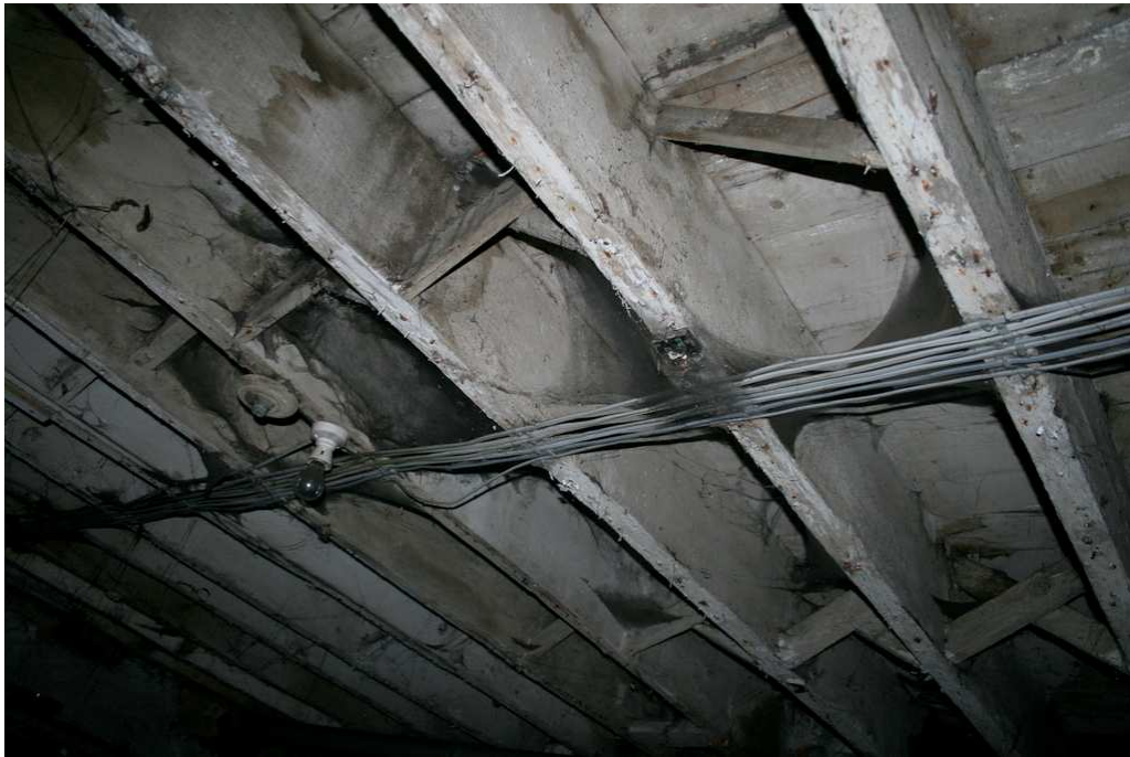
Plate 22: Detail of ceiling joist construction in cellar, 5 Greengate
