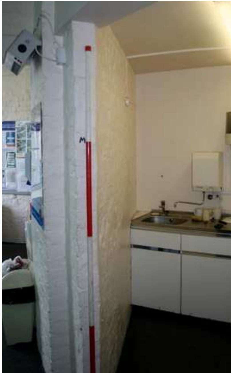
Plate 16: Chimney breast within partition wall, 1-3 Greengate
