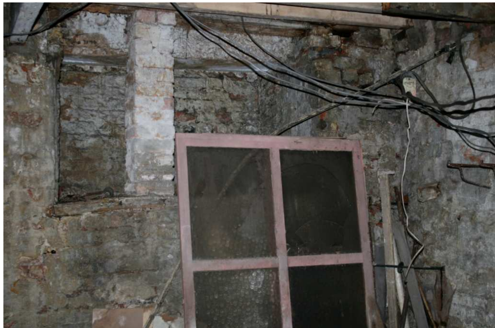
Plate 33: Cellar-light window, with supporting brick column, 7 Greengate
