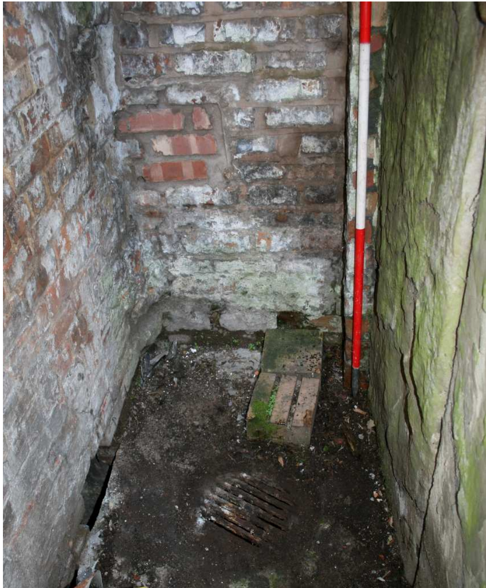
Plate 36: Drain in yard behind 5 Greengate, draining into cellar
