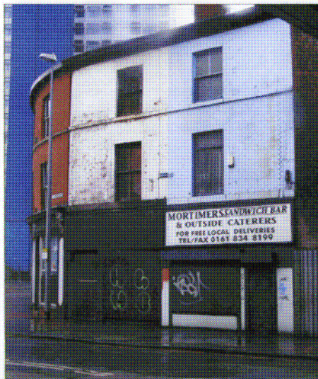
Figure 30 The Exchange, Greengate, Salford: Nos. 5 and 7 Greengate (40)
