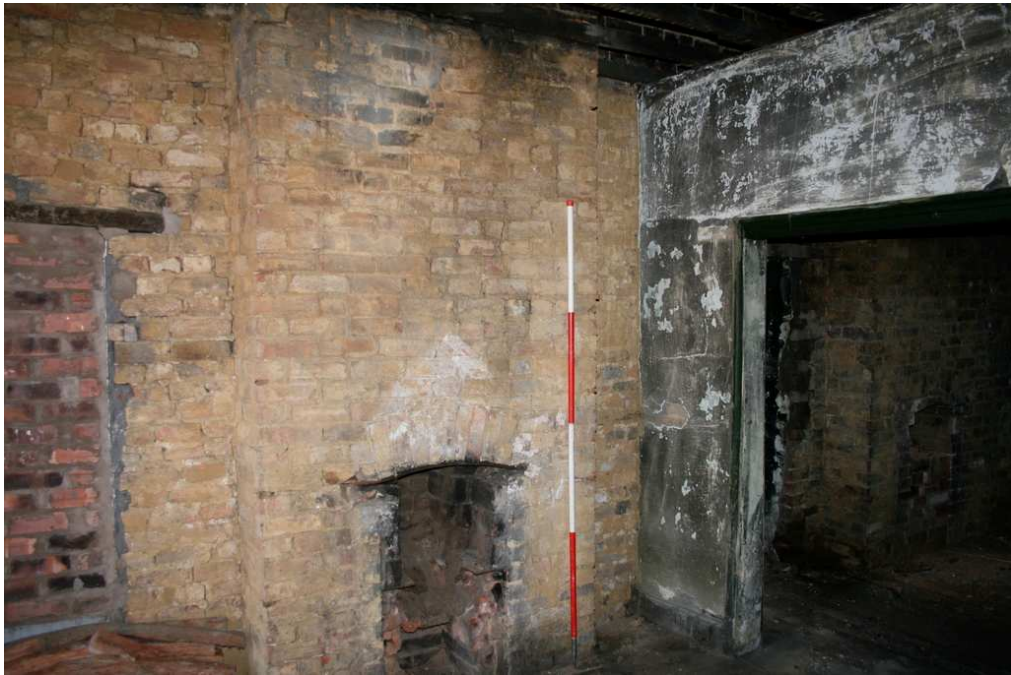
Plate 27: Remodelled fireplaces, blocked and inserted doorways, second floor, 7 Greengate
