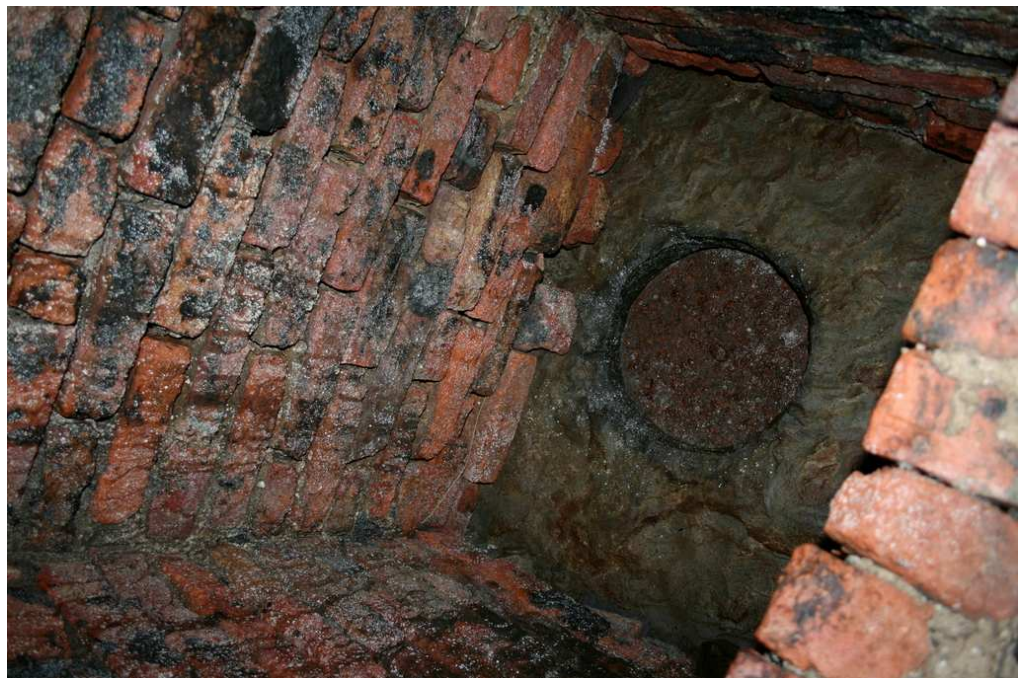
Plate 35: Circular aperture in yard floor into rear chamber of cellar, 7 Greengate
