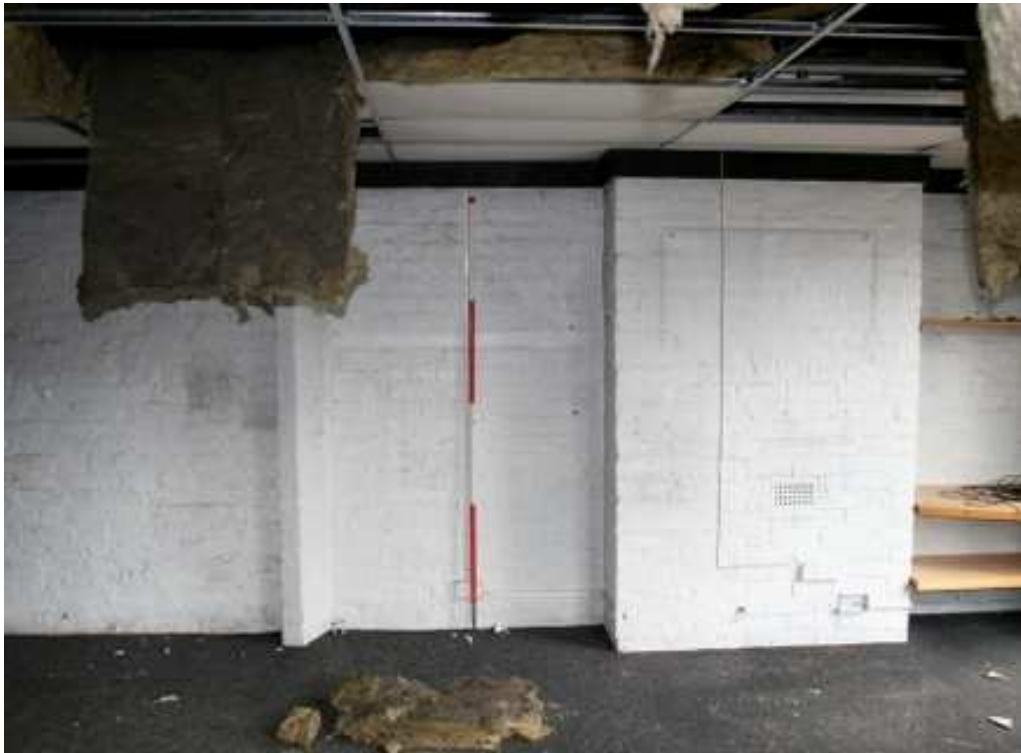
Plate 18: Blocked fireplace and stub of internal partition wall, second floor, 3 Greengate
