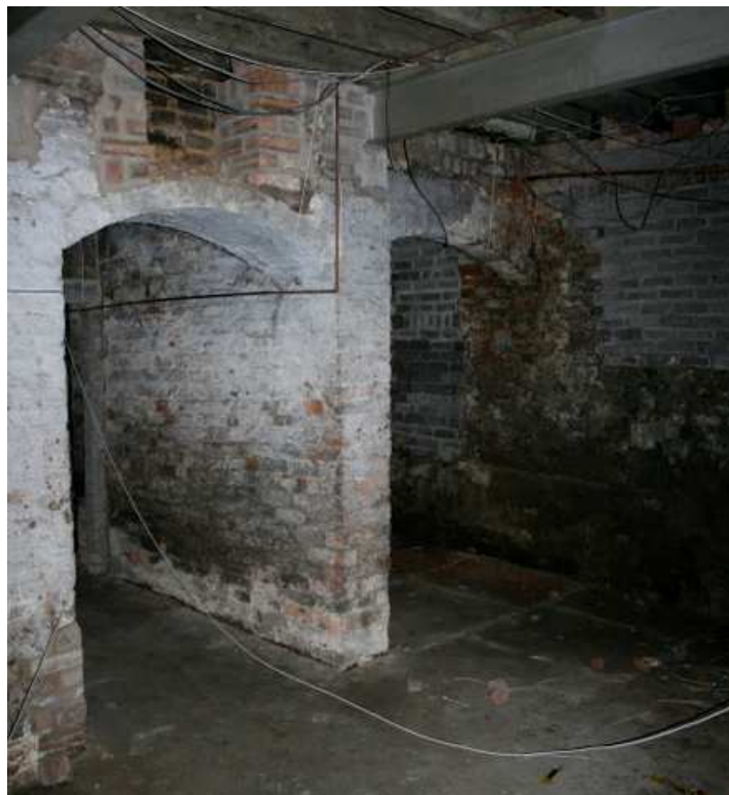
Plate 15: Vaulted alcoves within Cellar below 12-14 Chapel Street and 1-3 Greengate
