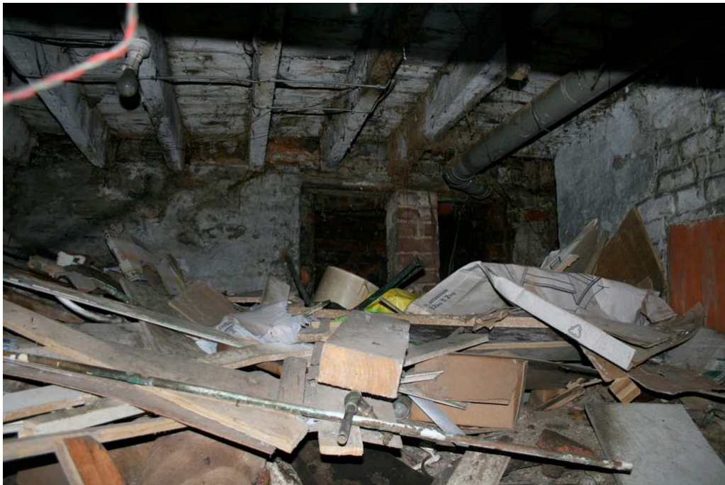
Plate 23: Rear cellar of 5 Greengate, filled with debris
