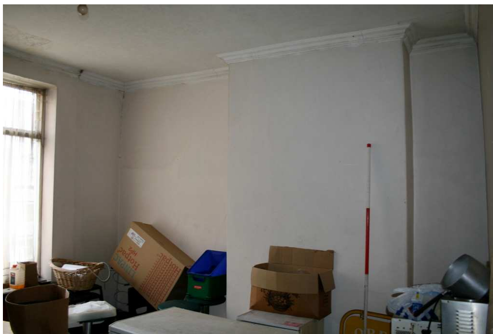
Plate 24: Blocked fireplace and decorative cornice, first floor, 7 Greengate
