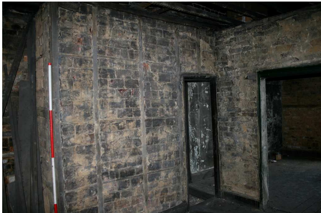
Plate 30: Edge-set brick nogging within timber panelled wall, second floor, 7 Greengate
