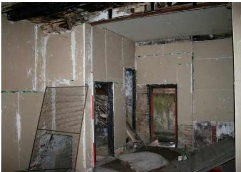
Plate 21: Original staircase, badly damaged by fire, then re-faced, 5 Greengate
