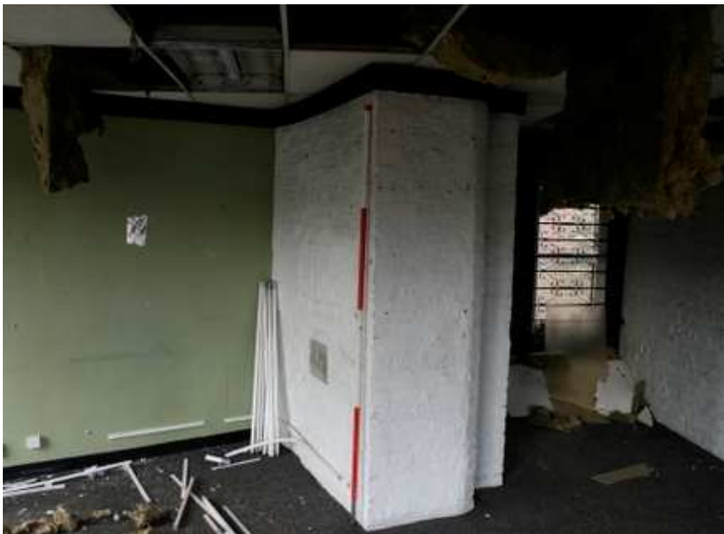
Plate 19: Blocked fireplace/flue within partition wall, second floor, 3 Greengate
