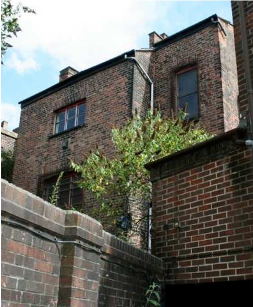
Plate 8: Extension to rear of 12-14 Chapel Street, constructed in English Garden Wall bond
