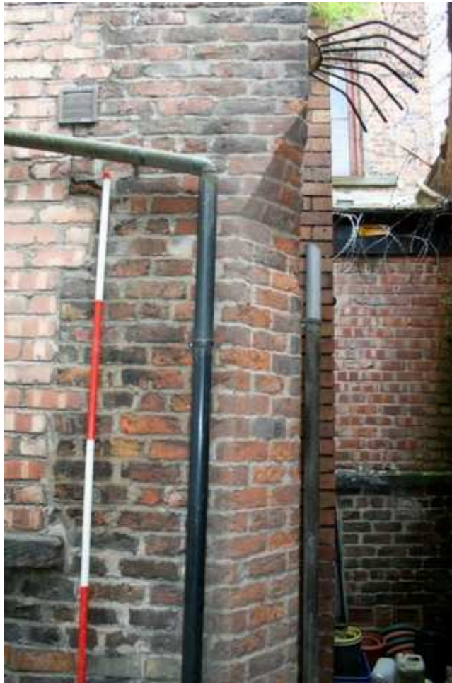
Plate 11: Chamfered return of extension to 12-14 Chapel Street
