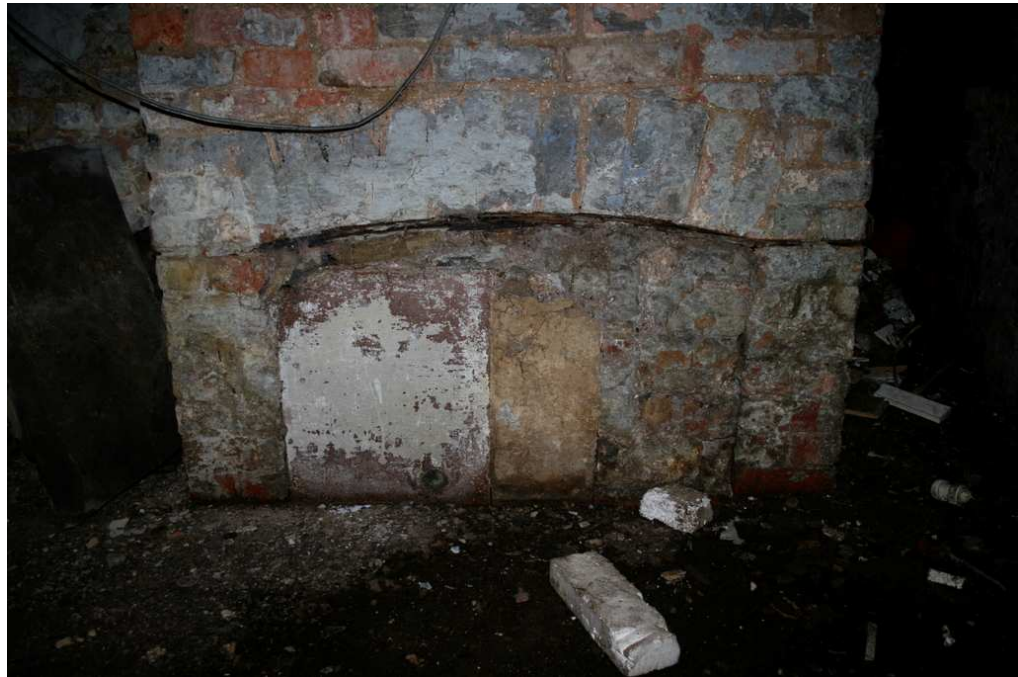
Plate 34: Blocked fireplace with iron-bar lintel, cellar, 7 Greengate
