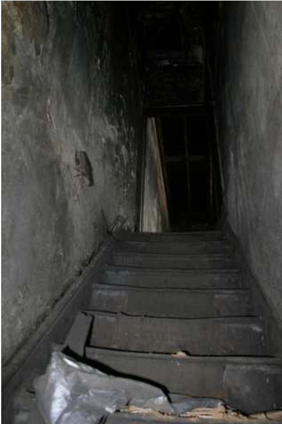
Plate 26: Detail of stairs to second floor, 7 Greengate
