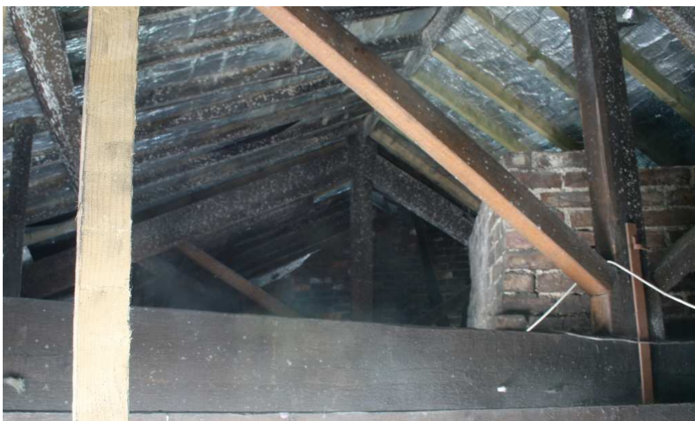
Plate 20: Detail; of roof trusses, 3 Greengate
