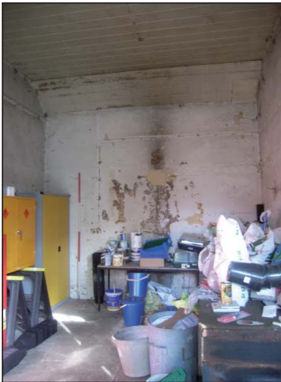
Plate 23: Interior view of area 6
