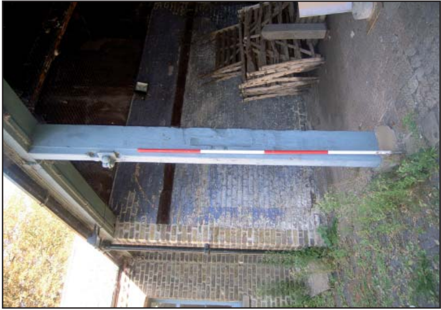
Plate 25: Detail of carriage door post in area 9
