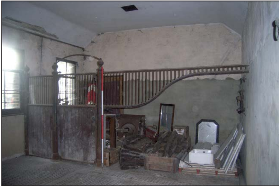
Plate 21: Later 19th century loose box divide in area 5
