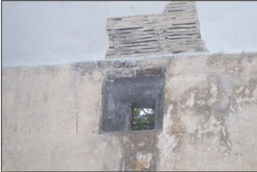
Plate 17: Detail of wall vent within area 3
