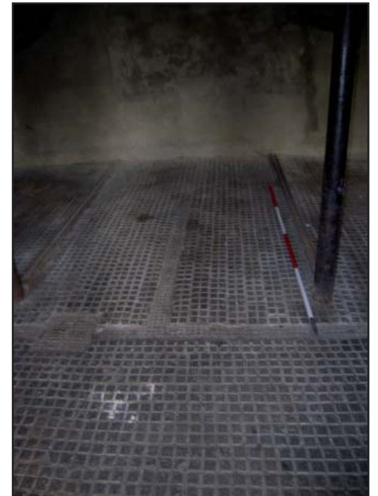
Plate 20: Detail of floor and drainage in stalls of area 5
