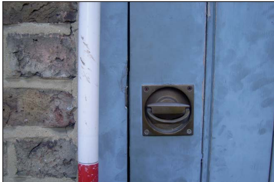
Plate 15: Detail of door fitting
