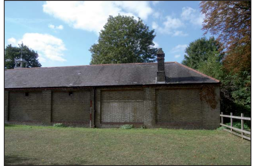
Plate 6: Detail of external elevation showing location of removed extension
