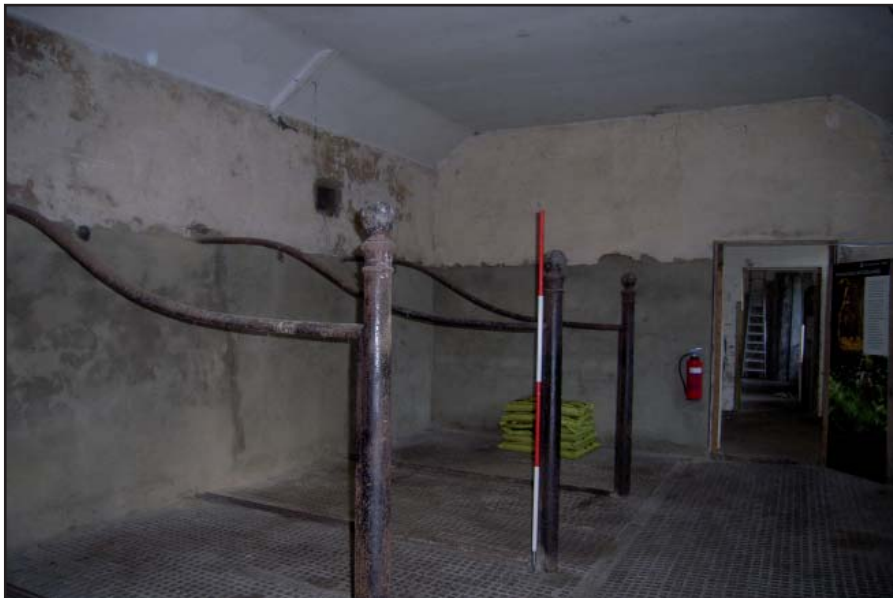
Plate 19: Cast Iron hind posts in-situ in area 5
