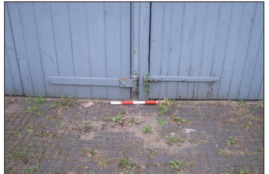
Plate 12: Detail of door hinges to area 2
