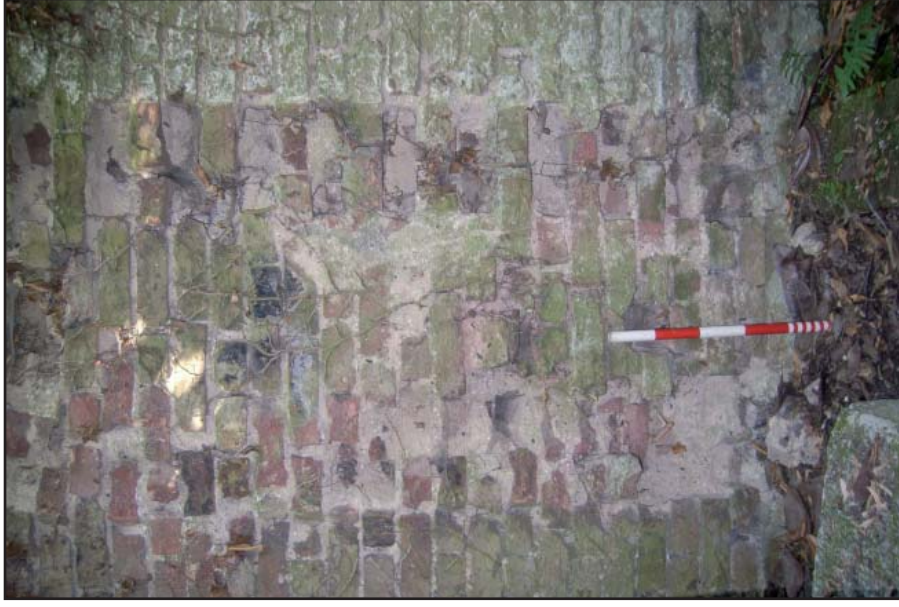
Plate 30: Detail of removed brick feature in former scullery
