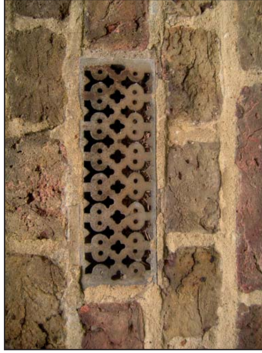
Plate 32: Detail of wall vent in external north elevation
