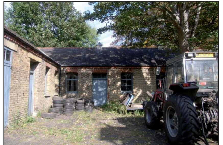
Plate 8: View of north west stable courtyard
