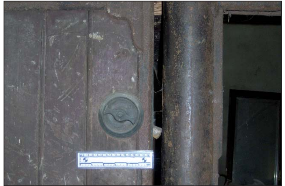
Plate 22: Detail of door fitting to loose box in area 5
