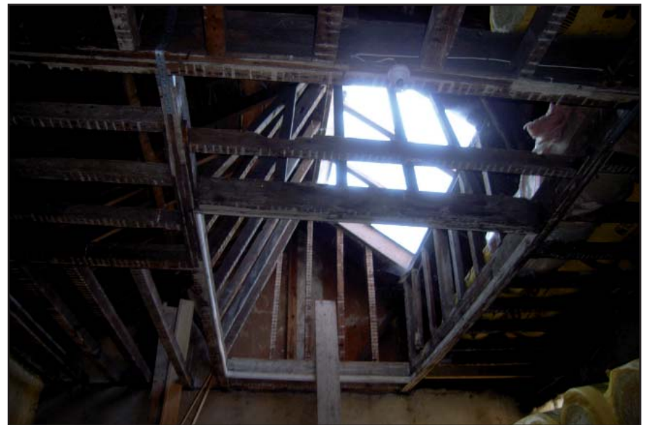
Plate 24: View of lantern and ceiling within area 8
