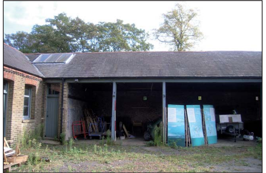
Plate 10: View of east range of stable courtyard
