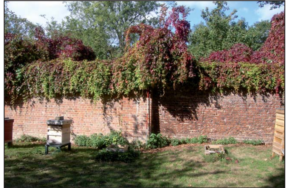
Plate 34: Detail of south facing elevation of orchard and apiary wall
