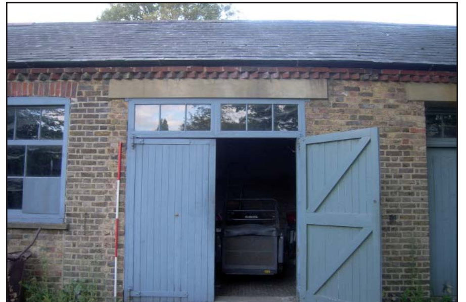
Plate 16: Blocked doorway and adjacent enlarged doorway in area 3
