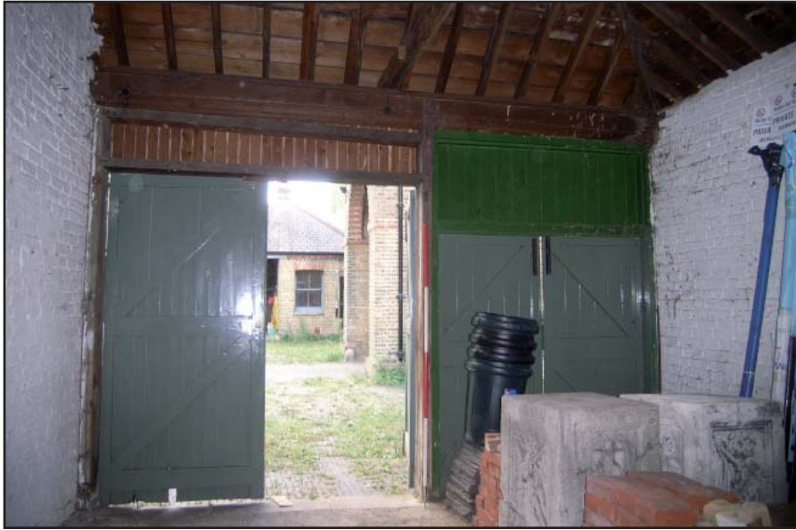
Plate 13 Interior view of area 2 showing construction of doors
