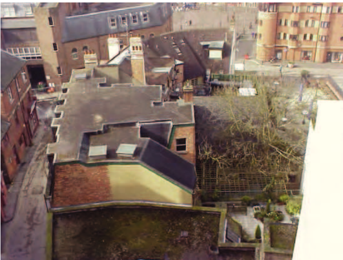
Flat roof seen from Debenhams building
