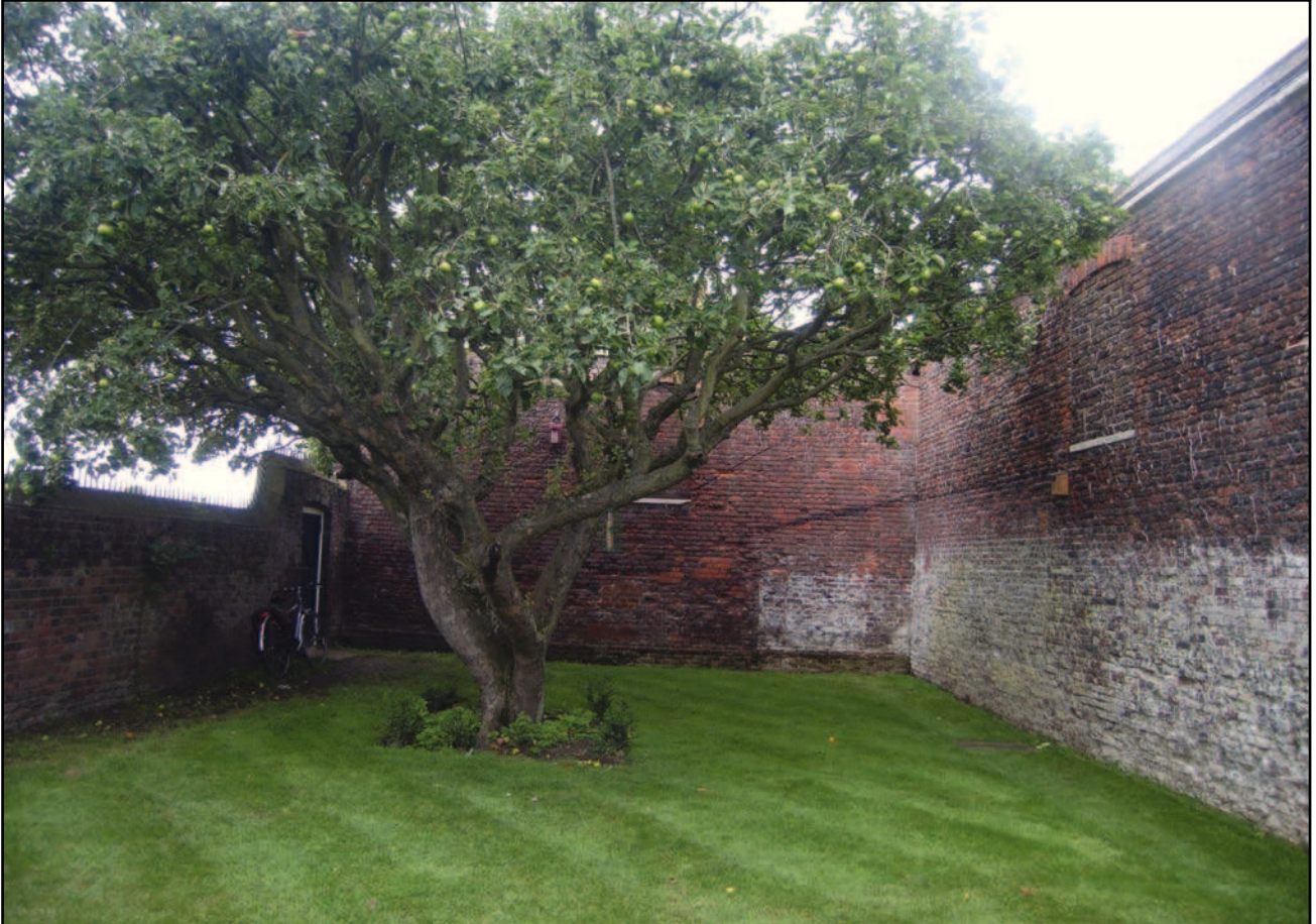
Plate 18: View of north elevation of garden wall showing extent of former lean to
