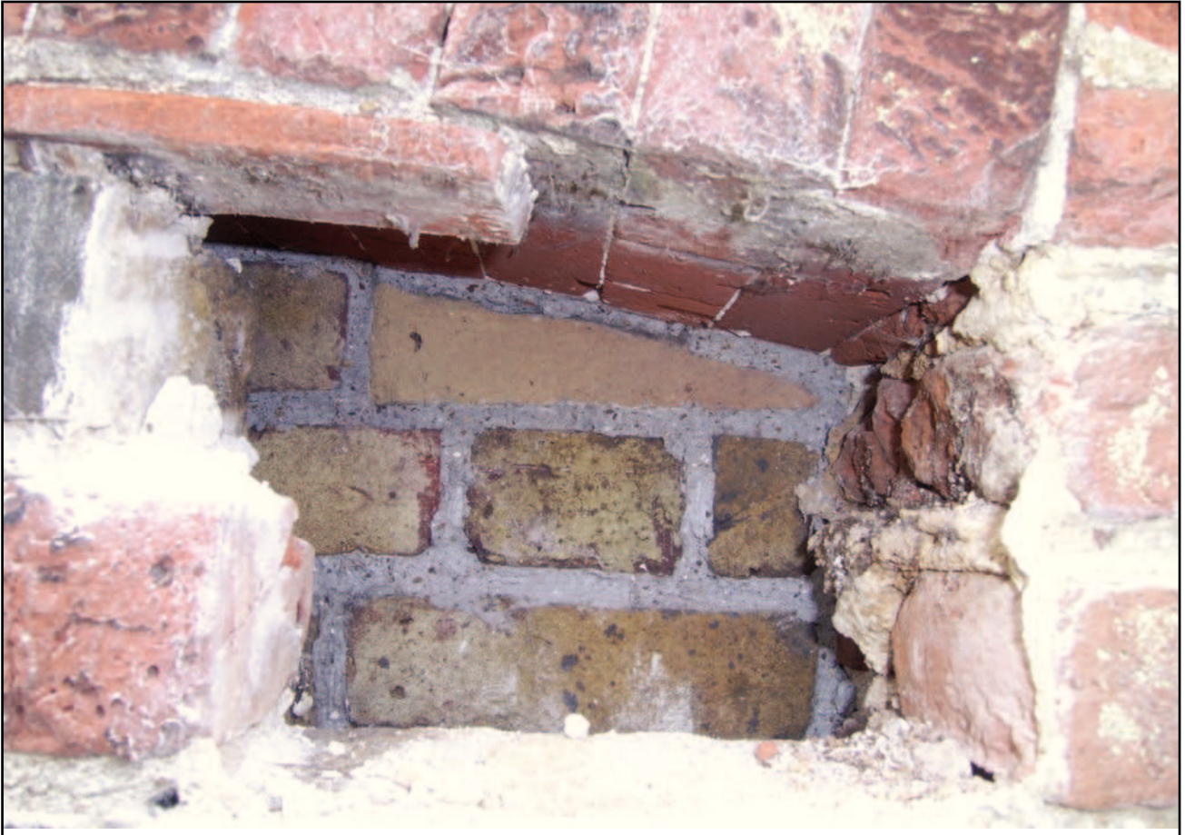
Plate 25: Opening up of upper infill brickwork on north west elevation
