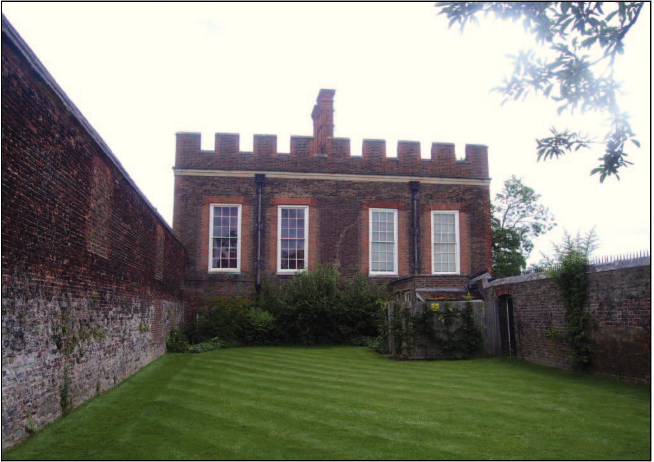
Plate 17: View of south elevation of Banqueting House
