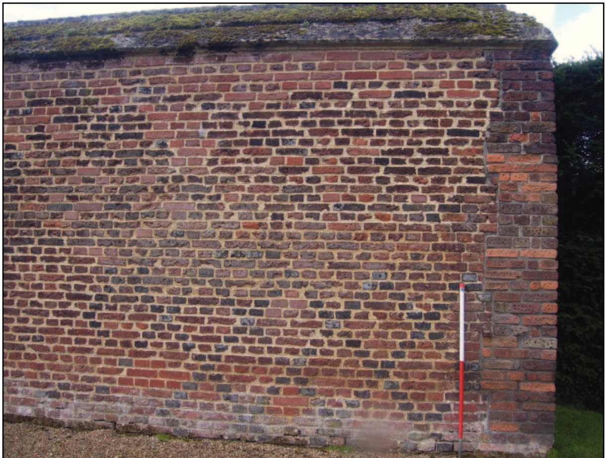
Plate 12: Tudor diaperwork and later rebuilt corner on north west end of wall
