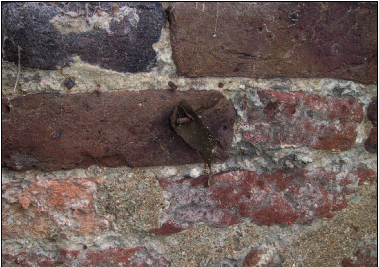
Plate 22: Detail of leather strap plant fixing on south east elevation
