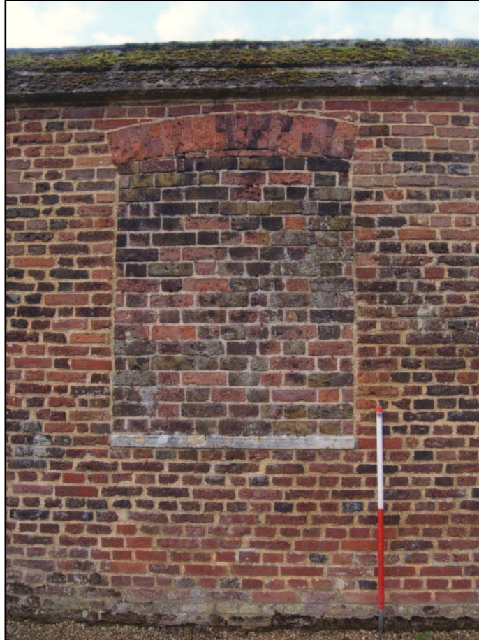
Plate 10: Infilled window opening with stone sill on north west elevation of wall
