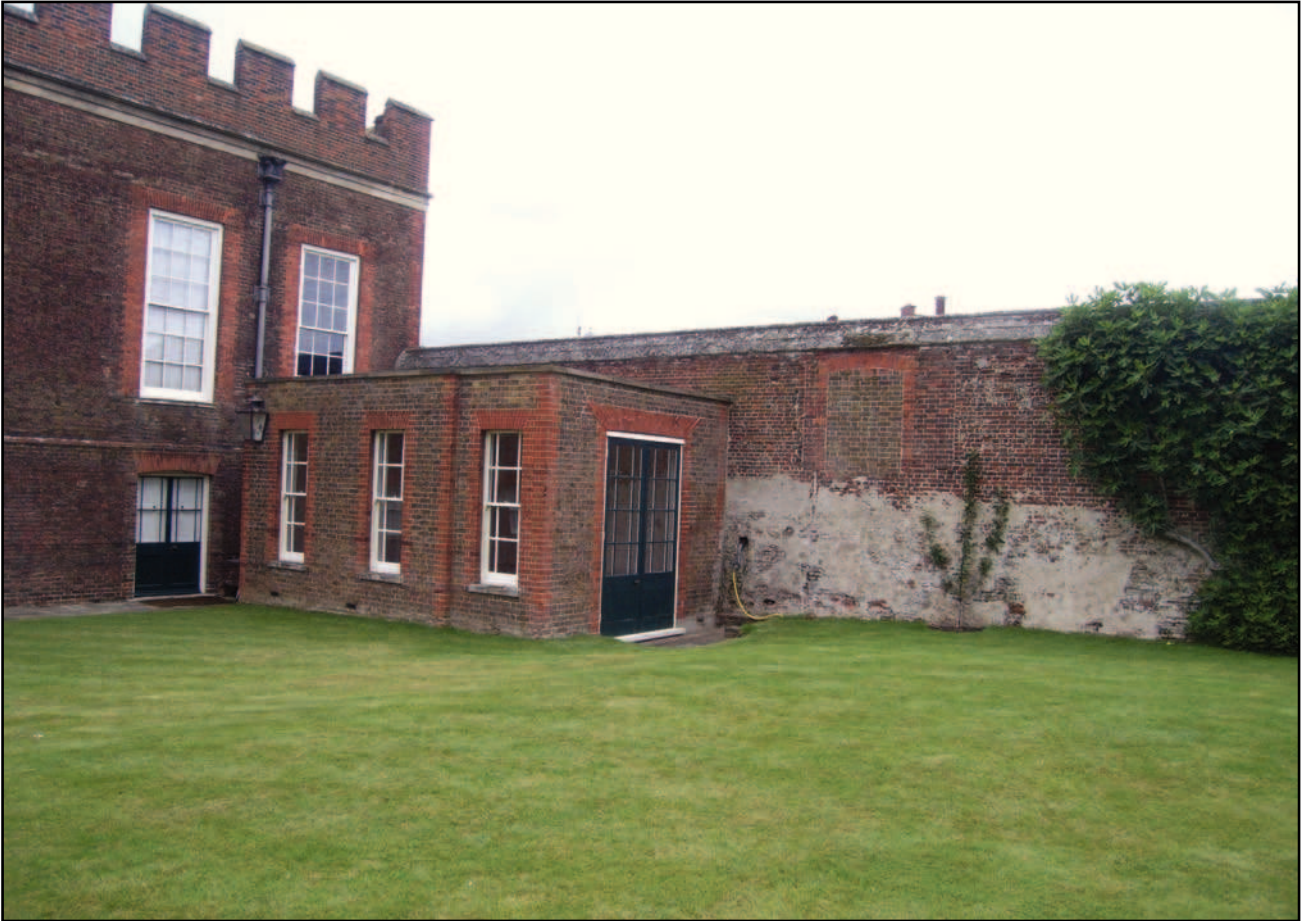
Plate 19: View of south east elevation
