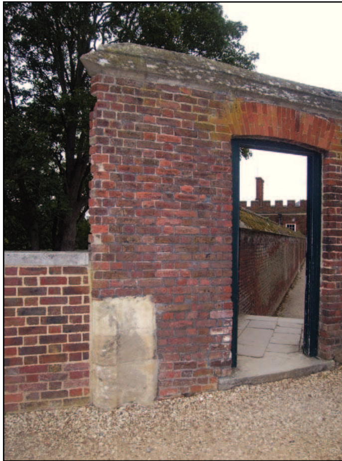
Plate 11: Moulded stone quoins on south garden wall
