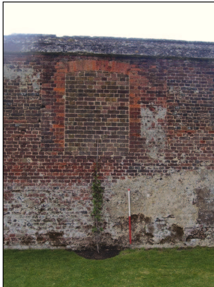
Plate 20: South east elevation detail of infilled window
