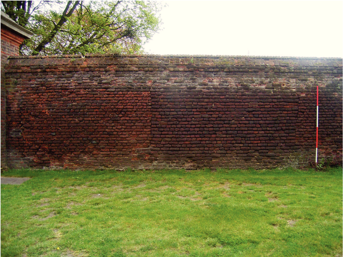
Plate 13: East elevation of west boundary wall showing 17th century infill
