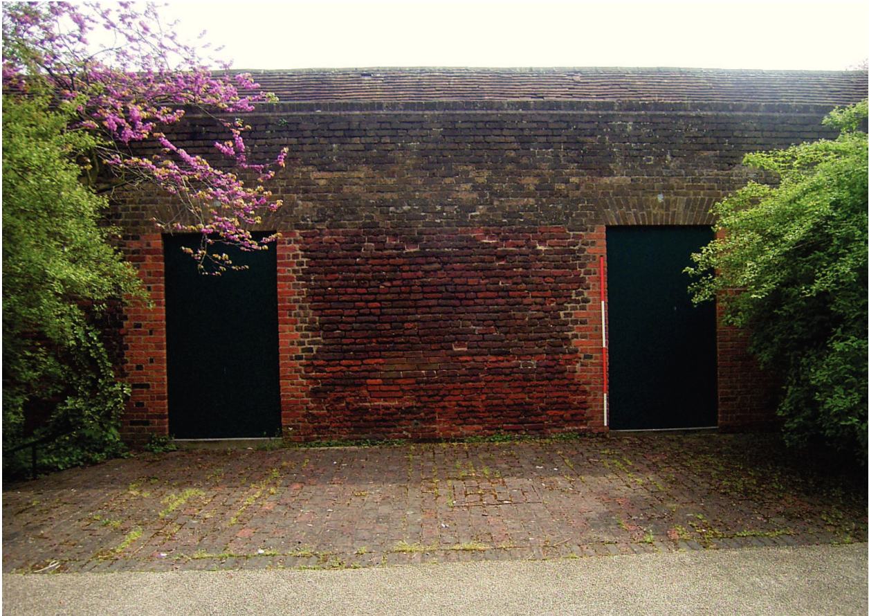
Plate 17: Inserted doorways within the Vrow Walk wall leading into the conveniences in the former putting green
