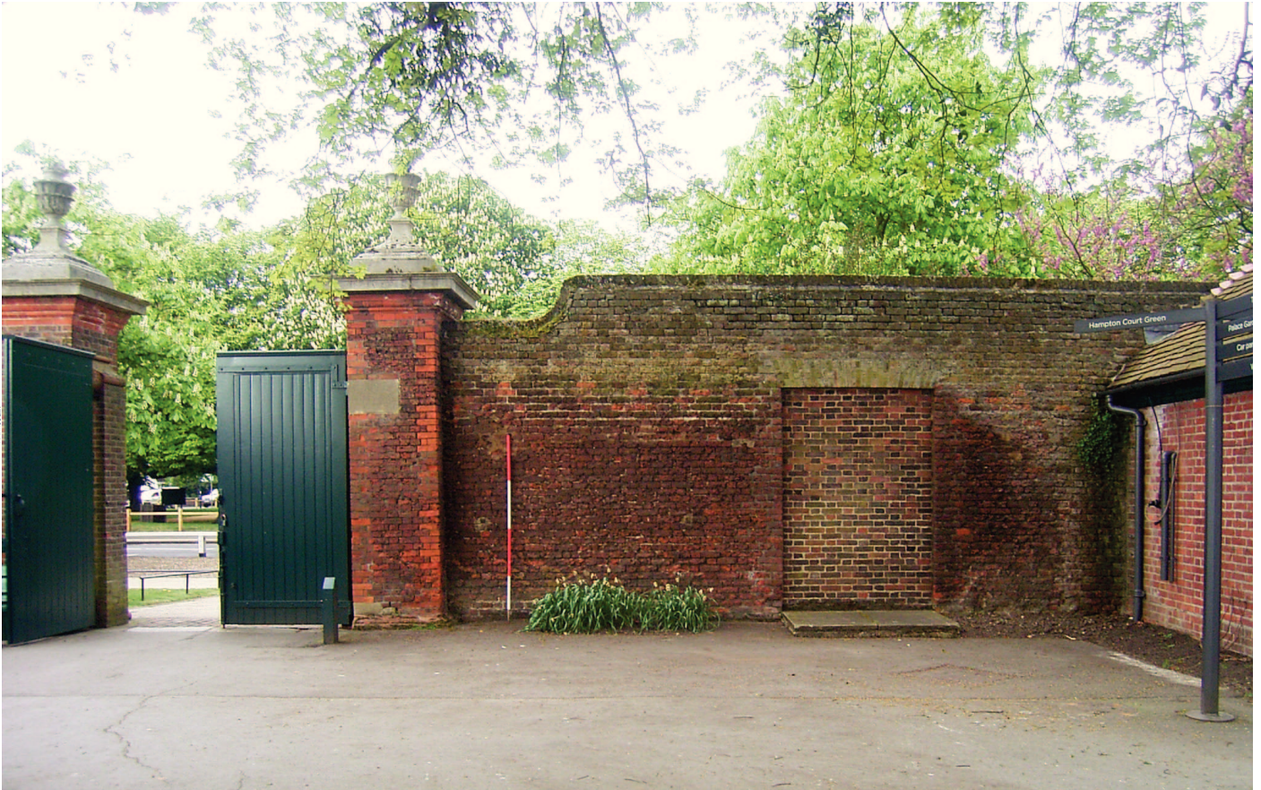
Plate 15: Gate leading onto the Vrow Walk and blocked 20th century turnstile entrance
