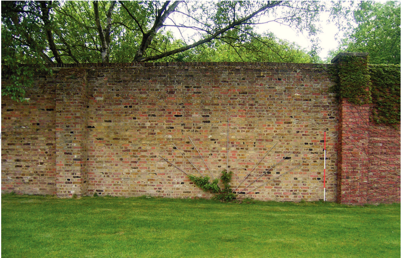
Plate 19: West elevation of west boundary wall with former tennis court showing modern refacing and darker brickwork belonging to the 18th century
