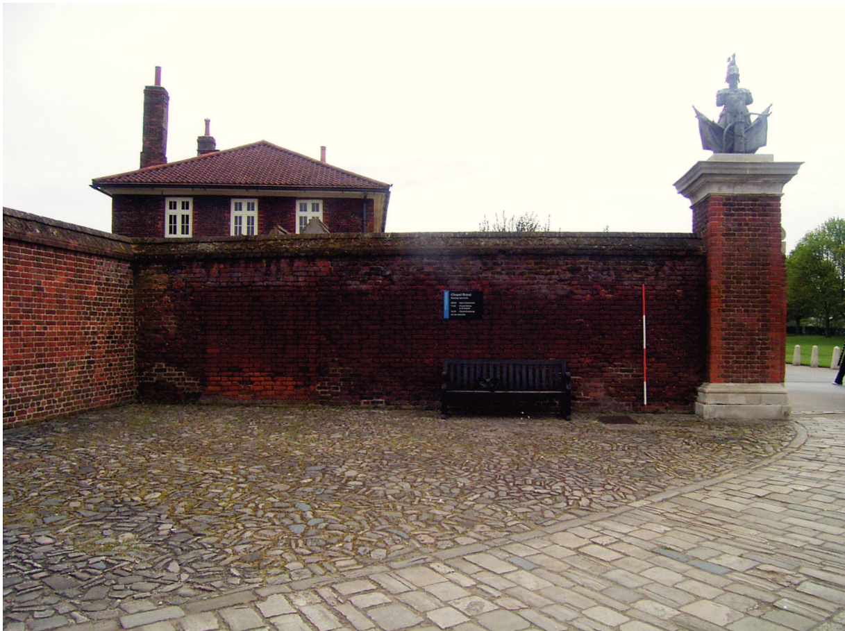
Plate 10: View of wall beside Trophy gate showing 19th and 20th century blocking in and rebuilding
