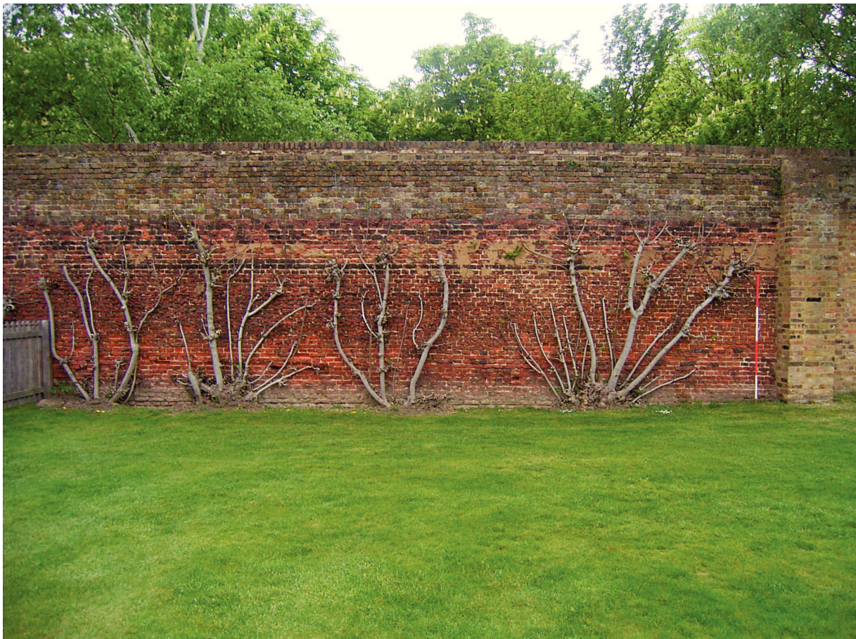
Plate 18: West Elevation of west boundary wall with former tennis court
