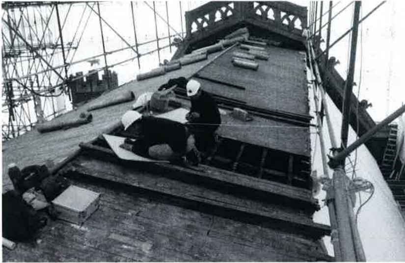
Figure 12: General view of roof from south-west
