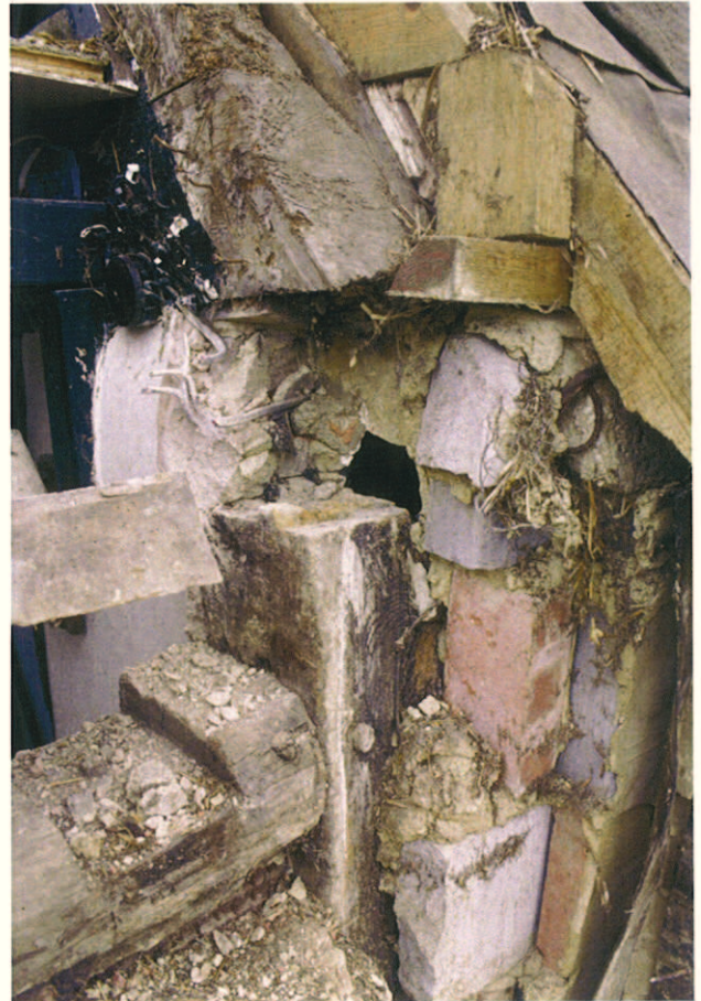
Plate 12 : Primary wall plate, post and tie at West corner of house
