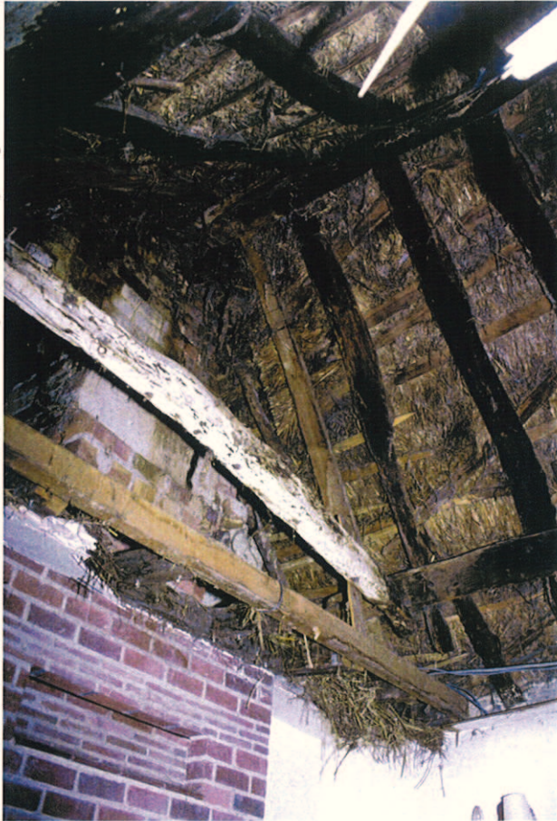
Plate 9 : Rafters on the South East slope at North East end
