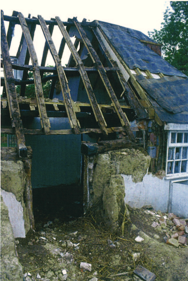
Plate 11 : Doorway in North East elevation
