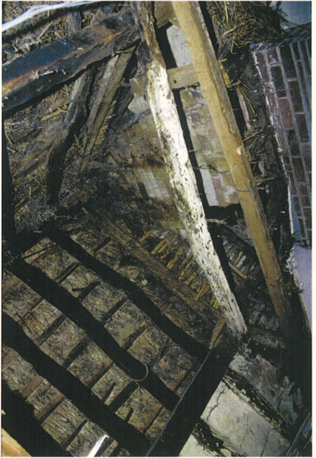
Plate 3 : Roof space and chimney stack at the North East end
