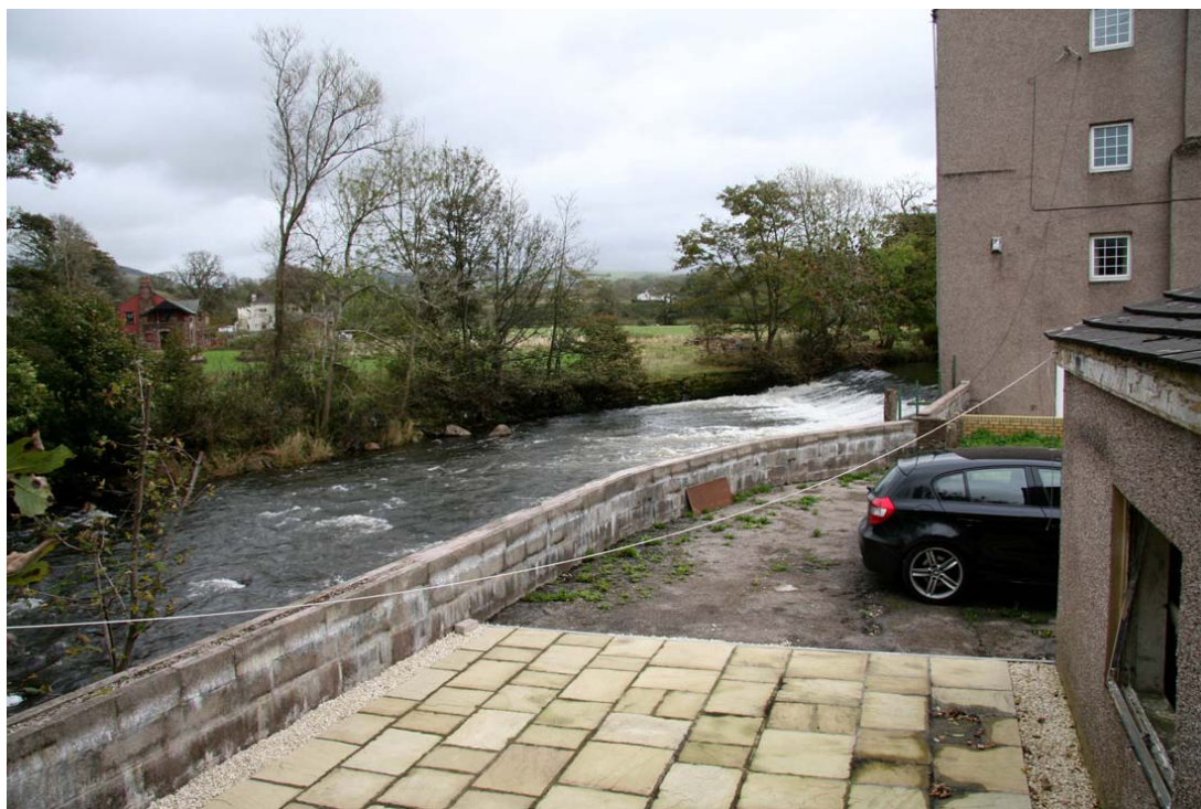
Plate 18: Weir associated with Bridge End Tannery
