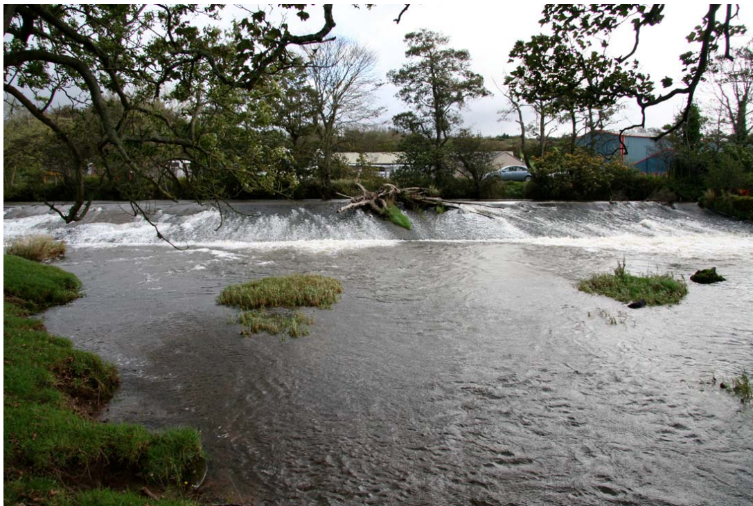
Plate 10: Looking south-east to Ennerdale Mill weir
