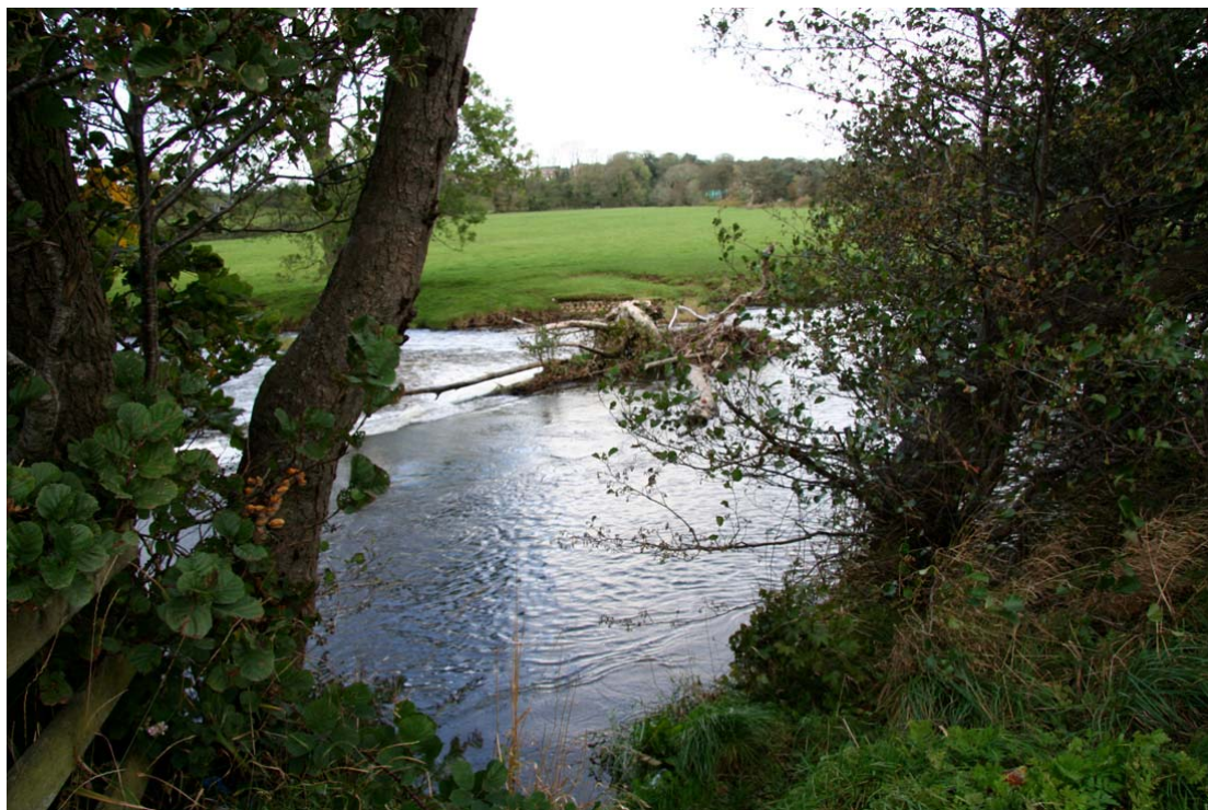
Plate 4: Looking north-west across the river Ehen to the wall on the north-west bank just below the weir
