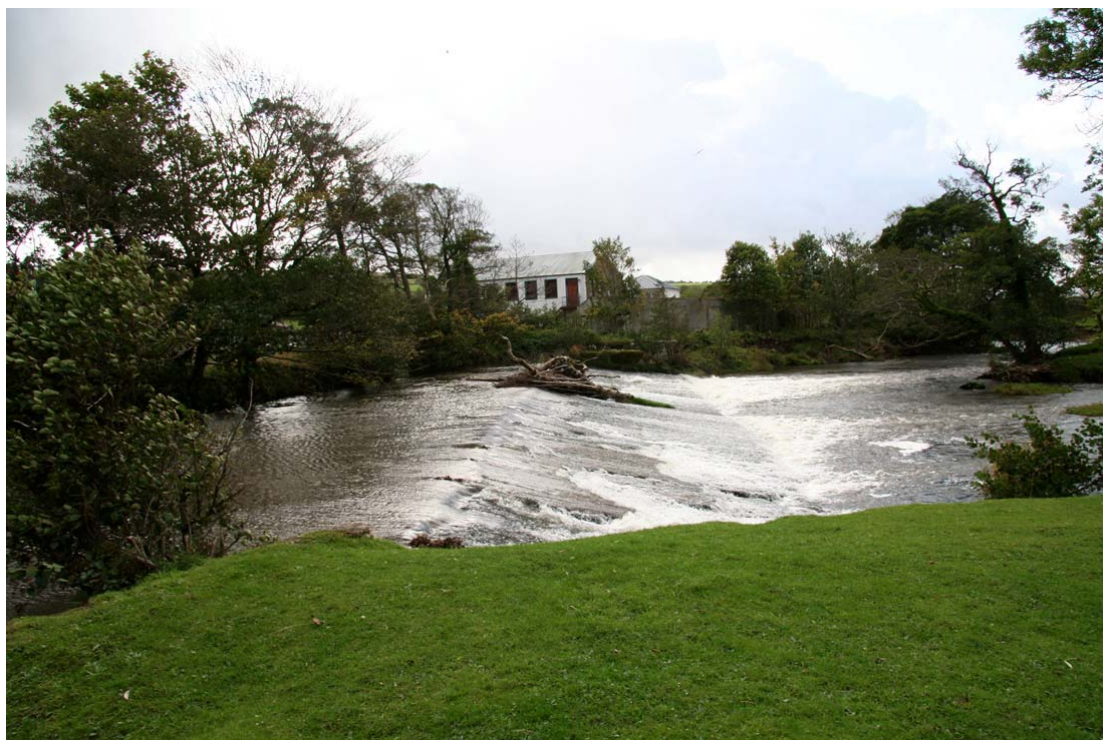
Plate 7: Looking south across Ennerdale Mill weir
