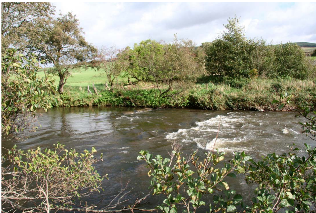
Plate 16: Brisco Mill weir from downstream
