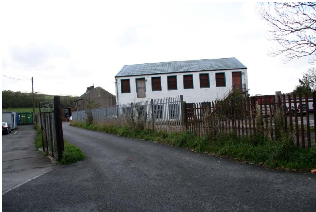
Plate 12: Possible nineteenth century Ennerdale Mill building, looking south. The road is located over the central mill race
