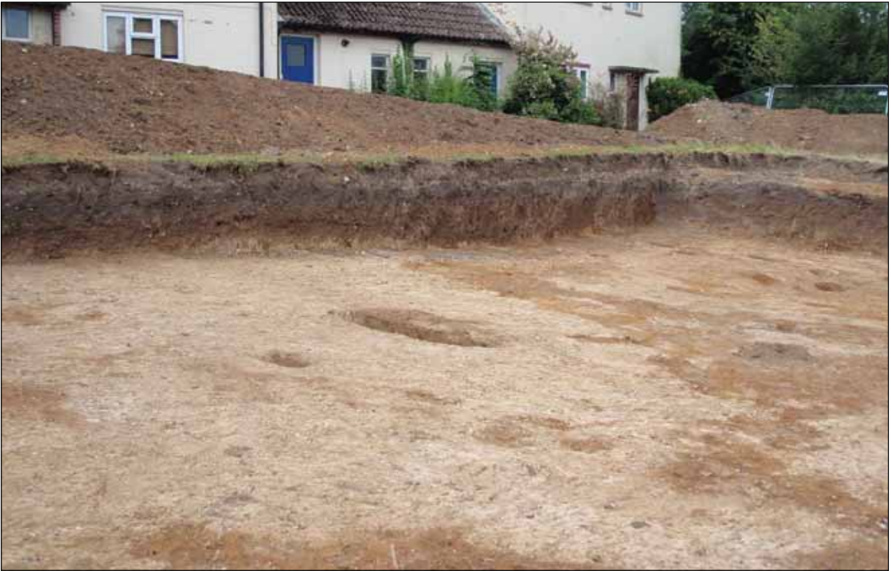
Plate 9: Terrace cut in western edge of excavation area
