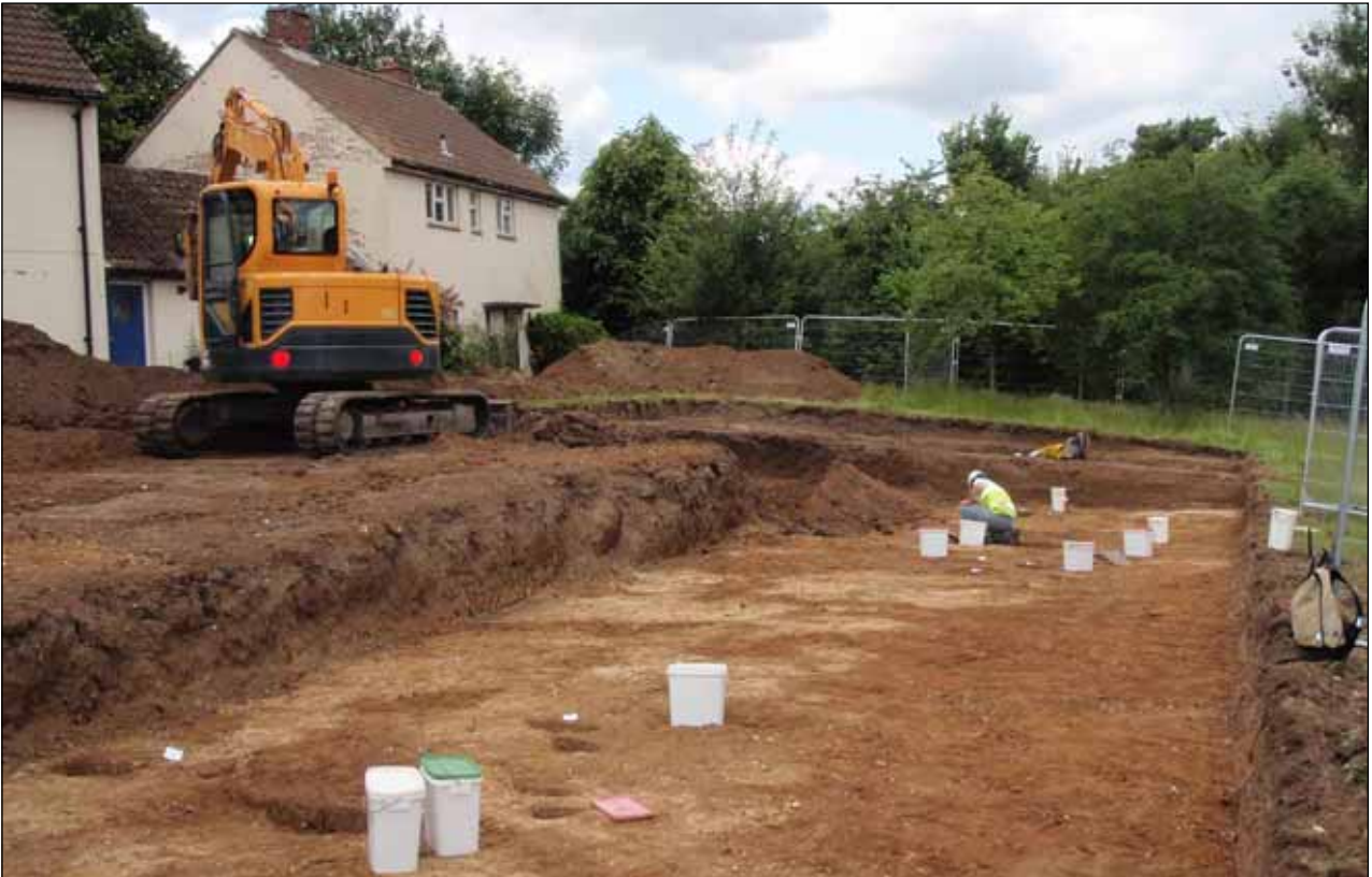
Plate 1: Working shot : site during excavation, from east
