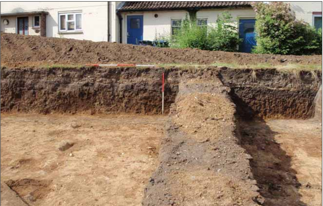
Plate 10: North-east facing section, showing demolition layers and terrace cut
