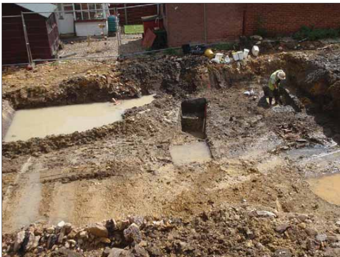
Plate 1: Excavation area looking east
