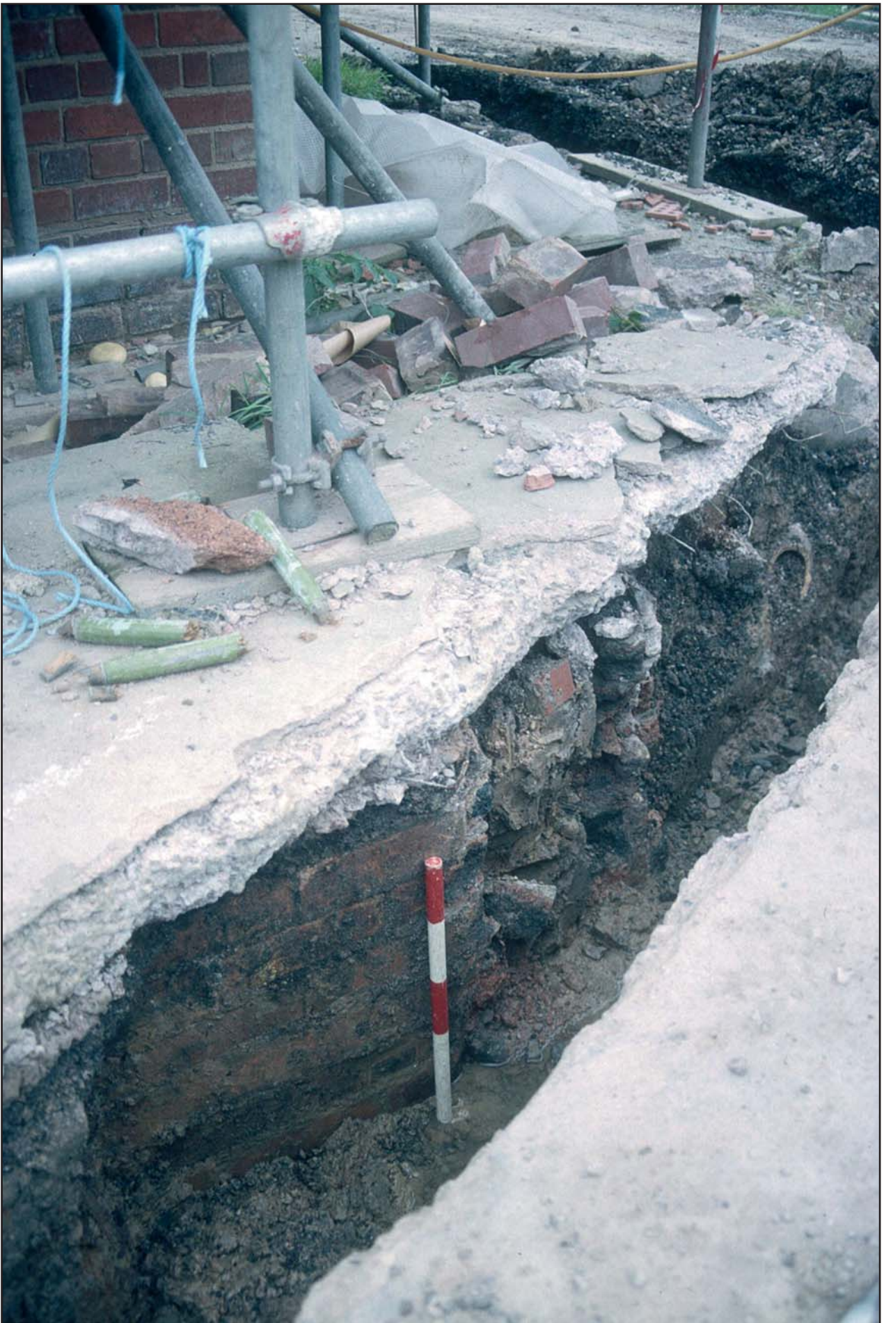
Plate 5: Foundations of lower laboratory building
