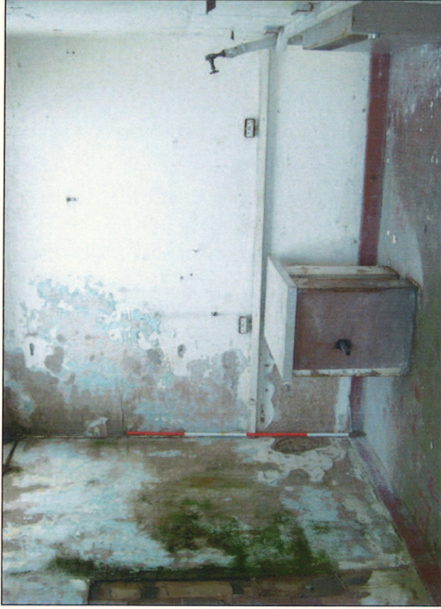
Plate 26: View within Room 2 looking north-east
