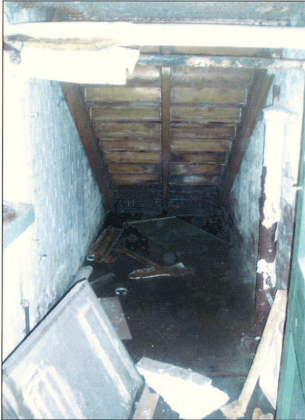
Plate 33: View beneath stairs looking south-west
