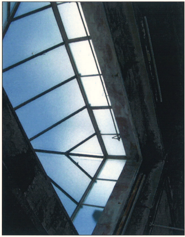
Plate 16: View of skylight in Room 1
