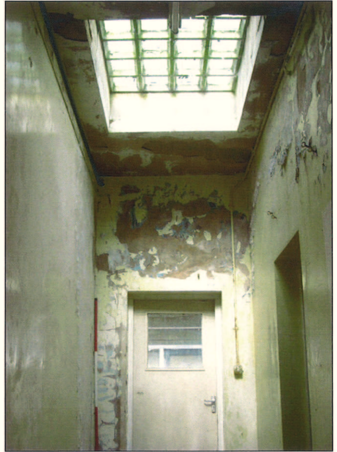
Plate 30: Roof light at north-west end of hall
