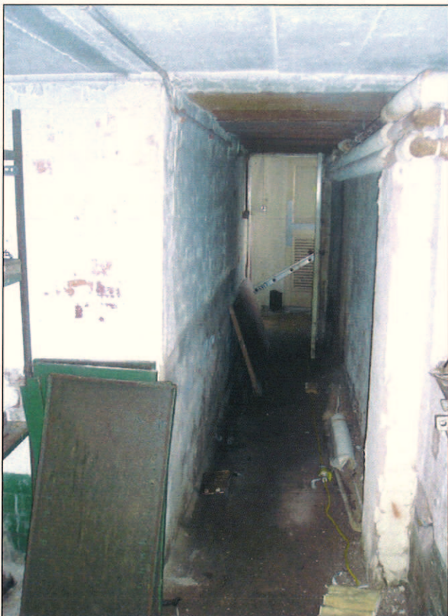
Plate 35: View of corridor looking south-west
